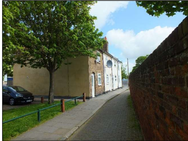
Photo 6. Terrace of 19 th century Cottages to north of the site
