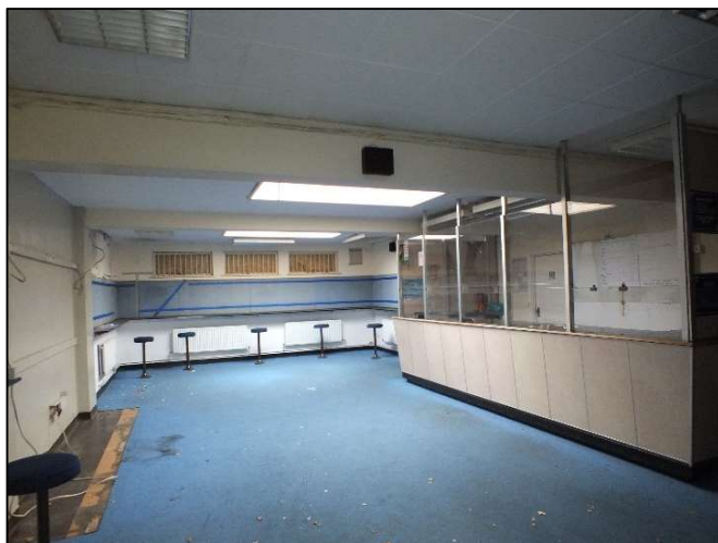
Photo 3. Ground Floor of No. 1 Cross Lane, looking south-east
