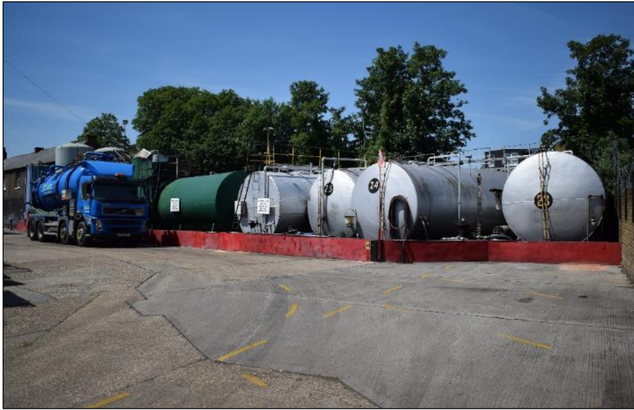
Photo 2: North-west corner of site, view from east
