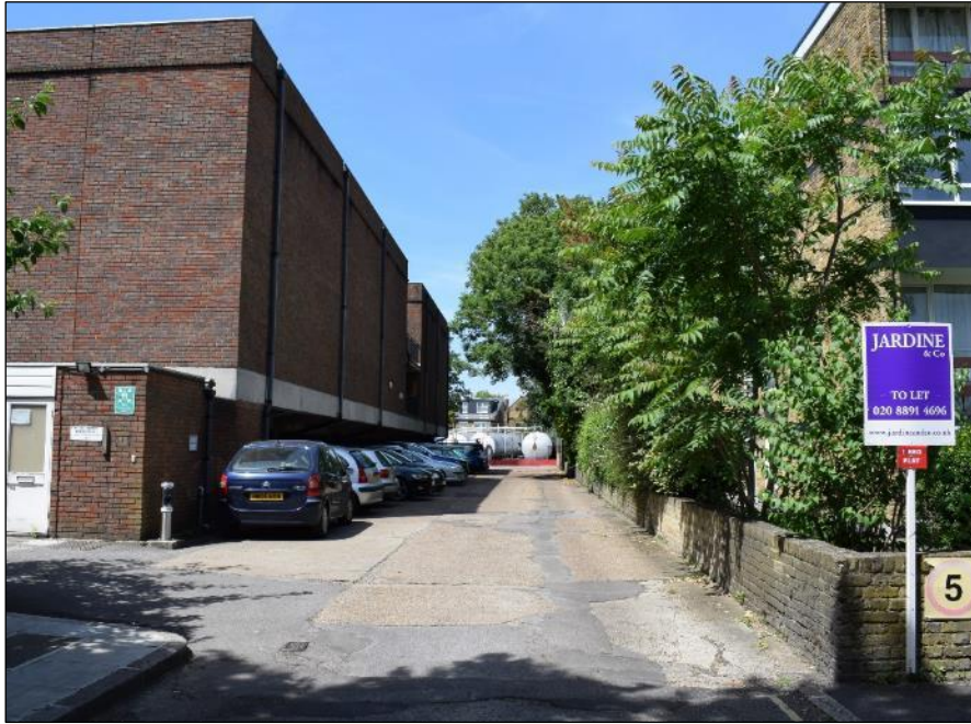
Photo 1: Approach to site from Arlington Road (view from south-west)
