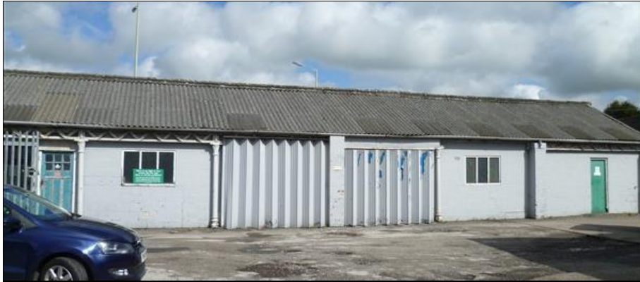
Photo 2: Northern Building: Southern façade looking north-west
