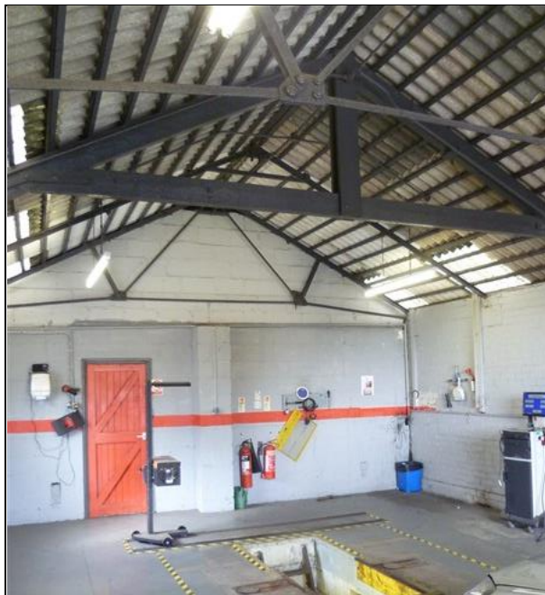
Photo 1: Northern Building: Internal view looking west
