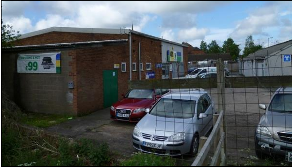
Photo 4: Southern Building: northern façade and eastern extension, looking south-west
