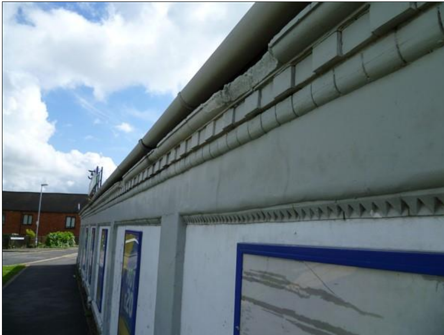
Photo 3: Northern Building: Northern façade looking north-east
