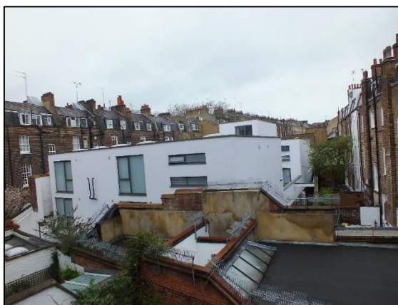
Photo 11: View from No.109, looking north-west
