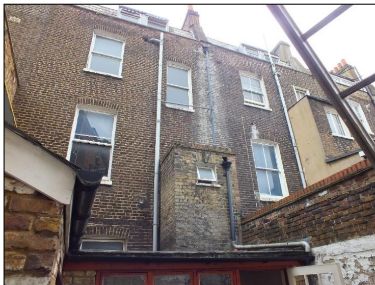
Photo 2: Rear elevation for Nos. 110 (left) and 109 (right) Guilford Street, looking south-east
