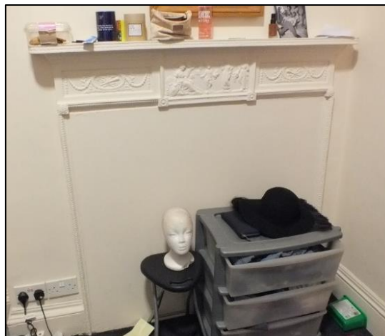
Photo 5: Original Regency fireplace in no 109: first floor, rear bedroom
