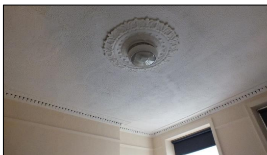
Photo 6: Ceiling rose and decorative cornice in no. 109: ground floor, front bedroom
