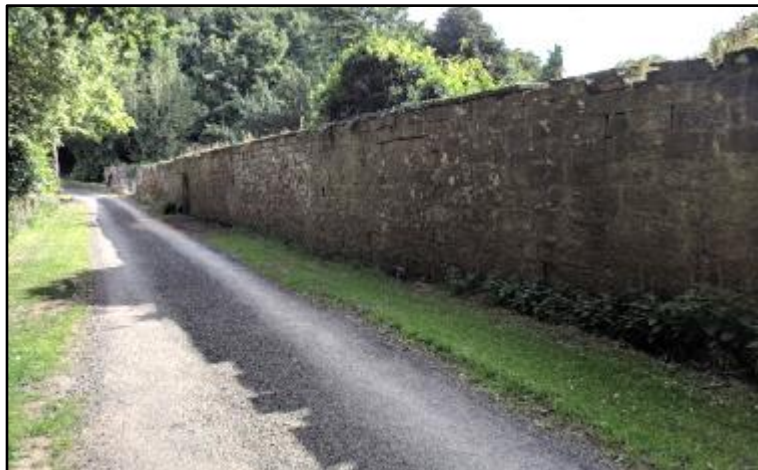
Photo 2. East boundary wall of the garden, looking south
