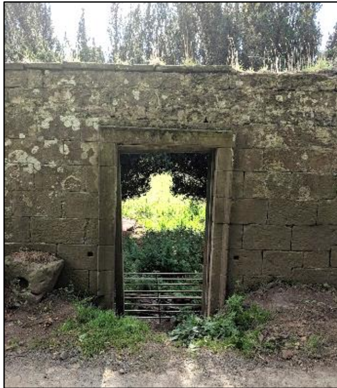
Photo 3. Entrance opening on eastern boundary wall, looking west
