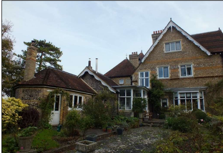
Photo 4: Side elevation of Darent Hulme, looking north-east
