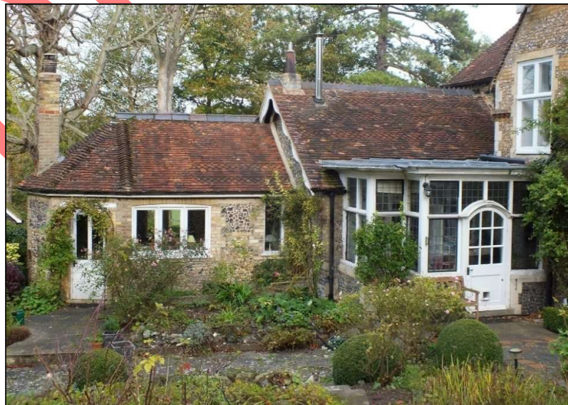
Photo 7: External view of study extension (left) and kitchen extension (right), looking north
