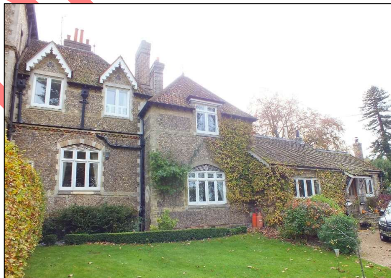
Photo 2: Front façade of Darent Hulme, looking south
