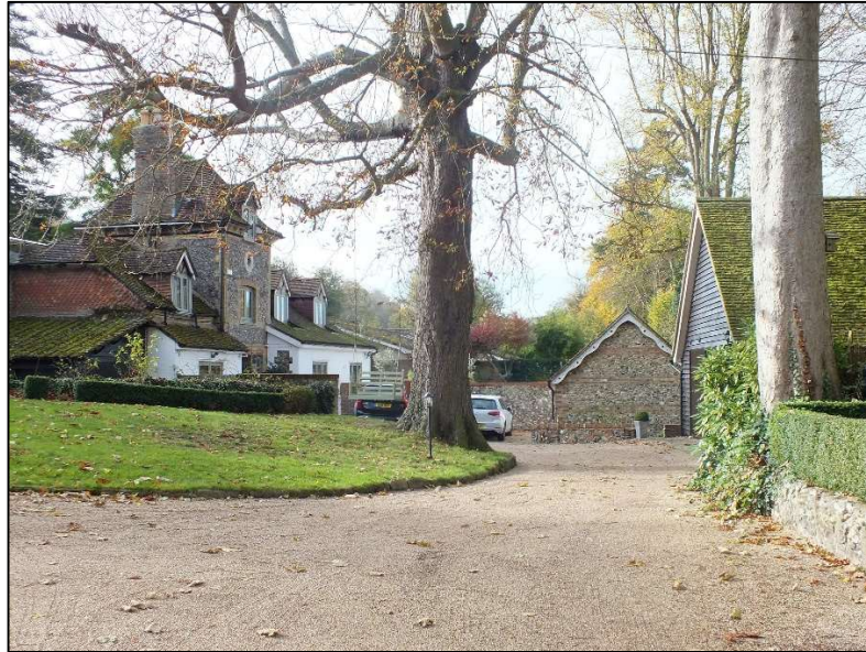
Photo 13: View of Coachhouse with modern garage/studio flat on right
