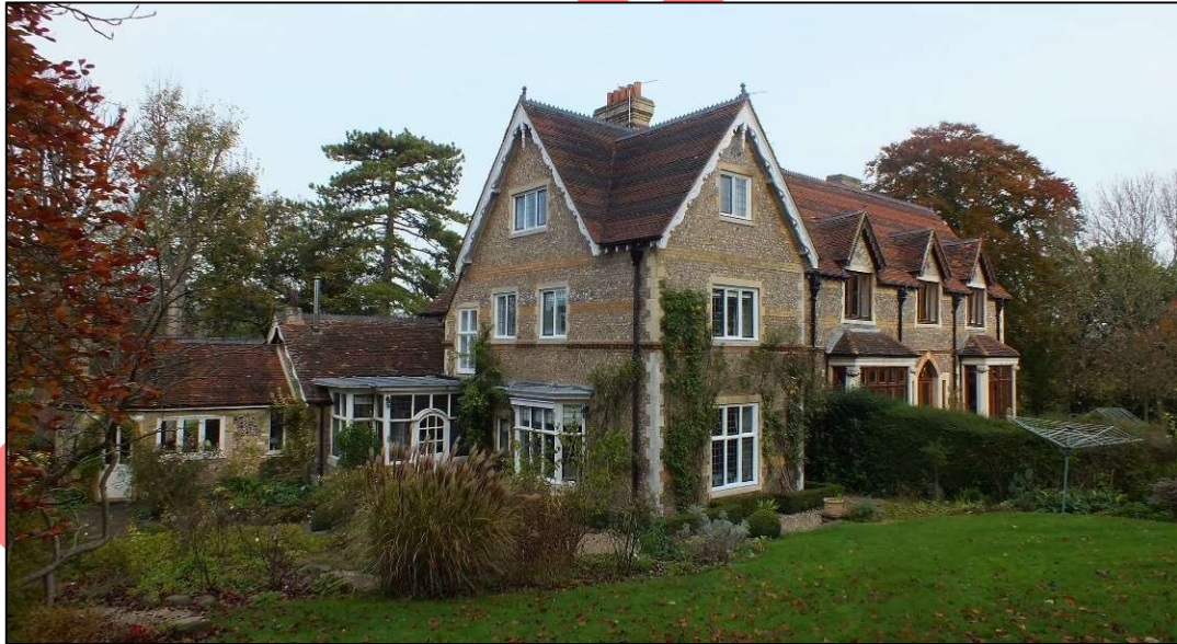
Photo 3: Side and rear elevations of Darent Hulme (with Darenth House on right), looking north-east
