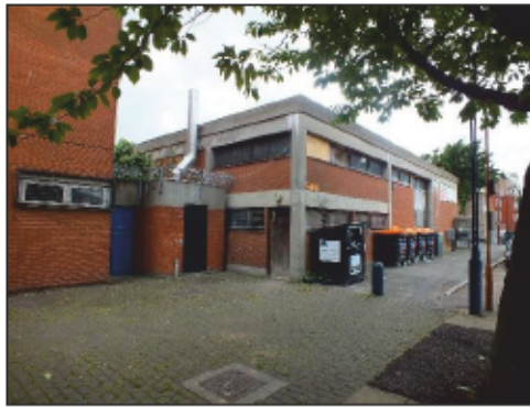
Photo 1: The site from the front of Pedro Street, looking north-east
