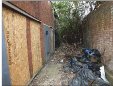
Photo 3: View of the western side of the site from Rushmore Road to the north
