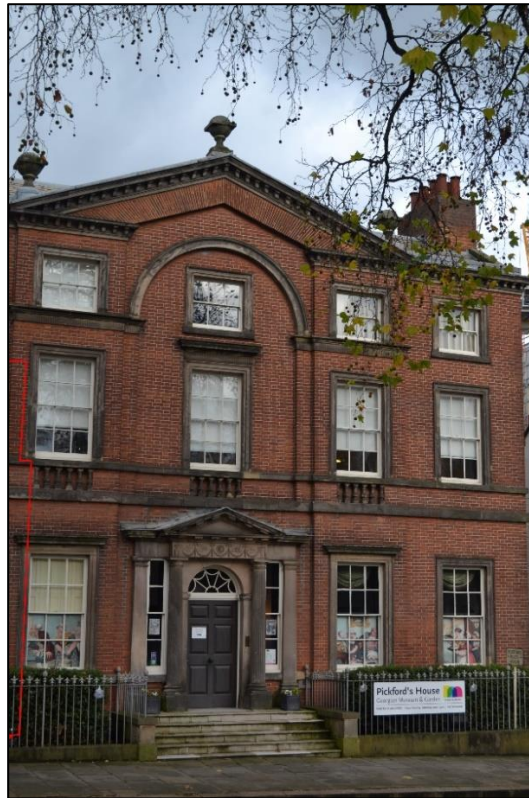
Photo 7. View towards the front of Pickford's House (Proposed Building shown as redline)
