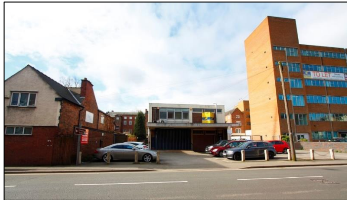
Photo 1. Looking SW. Number 18 Agard Street in the centre of the shot. Northgate house to the right of shot
