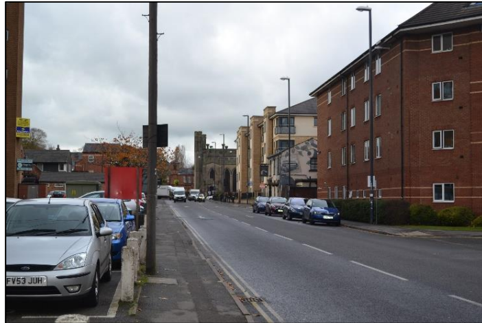
Photo 10. Looking north west towards the church
