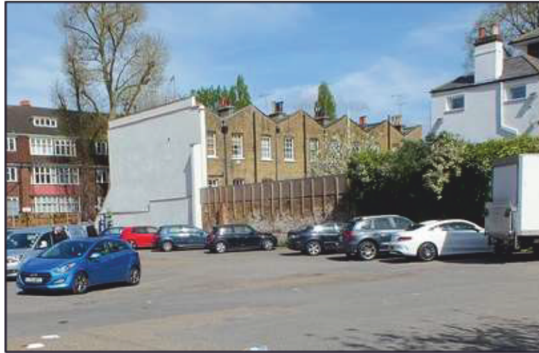
Photo 6: Rear of Queensberry Place [AB 116], from site, looking north
