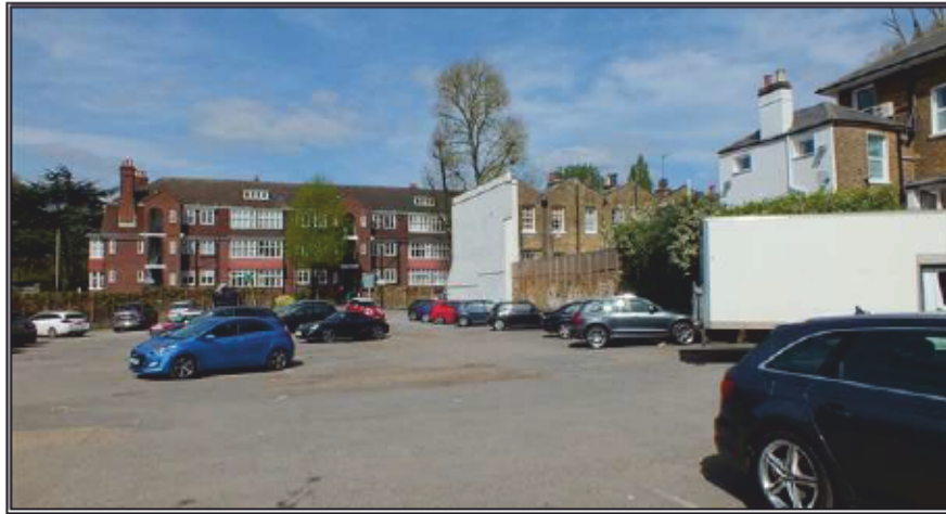
Photo 9: View across site towards the rear elevation of Queensberry House [AB 143], looking north-west
