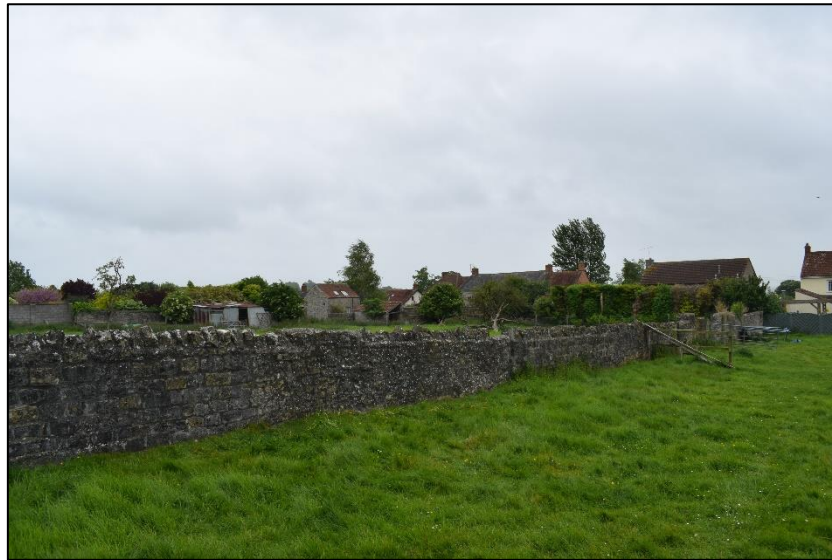
Photo 1: Looking East. Showing lias stone enclosing wall
