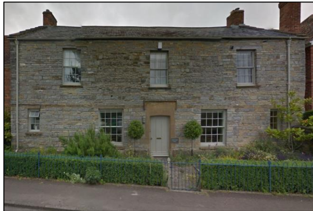
Photo 4: Front of Middlethorpe House
