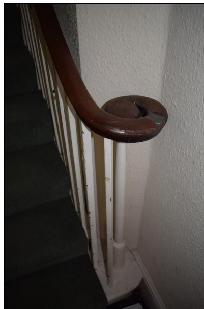
Photo 6: Spiral end of the main staircase handrail
