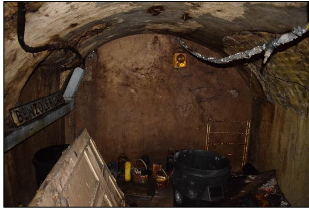
Photo 9: One of the basement vaults
