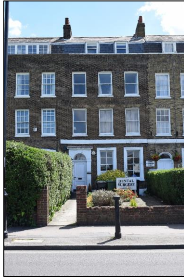
Photo 1: Front (north-west facing) elevation from Montpelier Row
