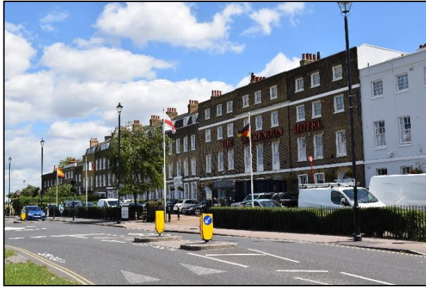
Photo 10: Montpelier Row from the south-west
