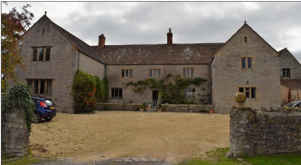
Photo 1: Lower Huxham Farmhouse, north elevation
