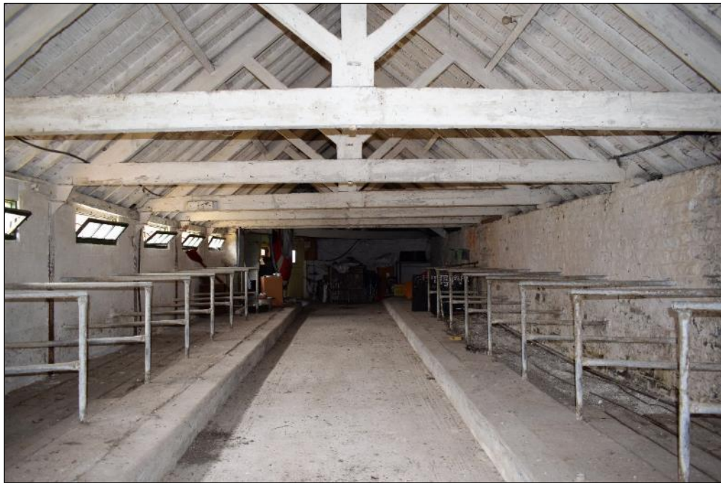
Photo 15: Interior of Barn E, north-south arm, looking north
