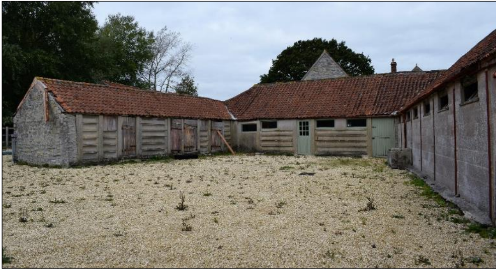
Photo 12: Barn E complex, view from south-west
