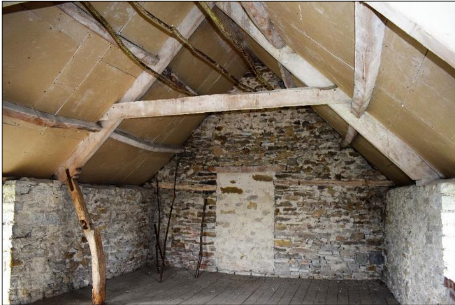
Photo 19: First floor of northern structure, Barn G
