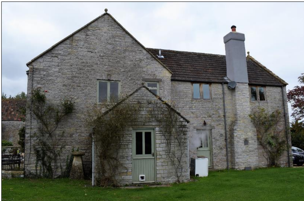
Photo 3: Eastern elevation of the house
