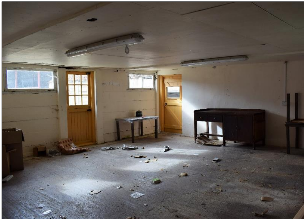
Photo 16: Internal room, northern range of Barn E
