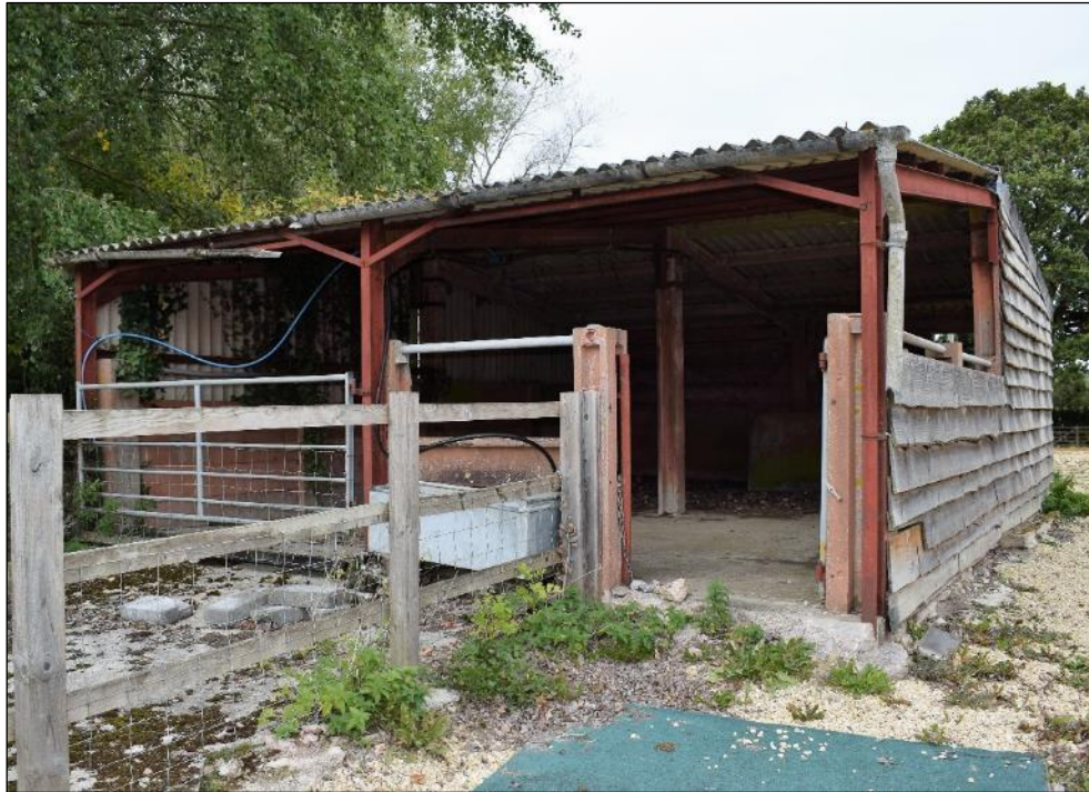
Photo 8: Barn D, view from south
