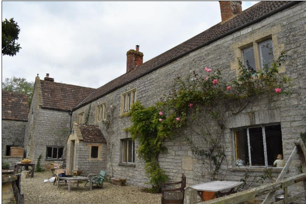
Photo 4: Southern elevation of the house, view from south-west
