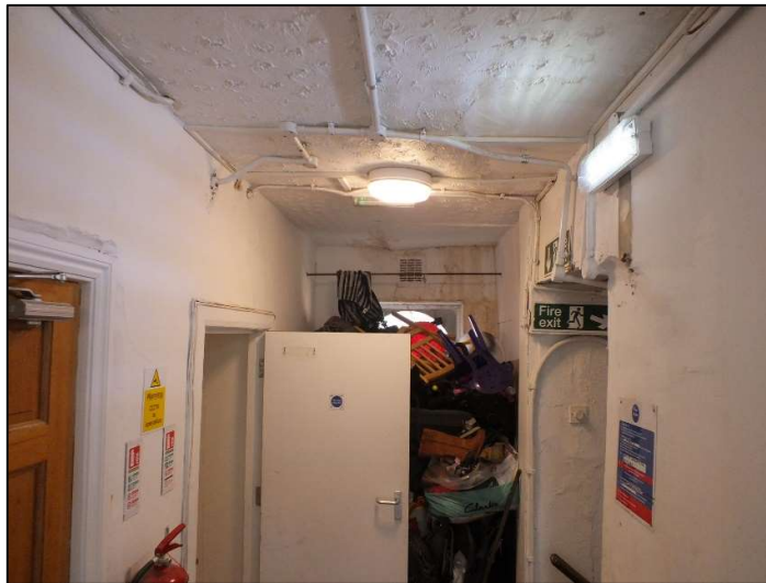
Photo 9. First Floor lobby looking west towards front of the building
