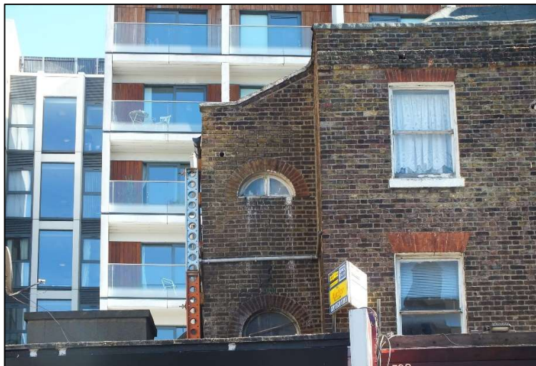
Photo 2. North wing of 592 Kingsland Road
