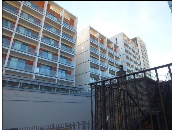
Photo 15. View from rear of 592 Kingsland Road
