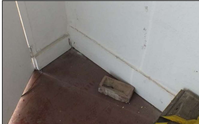
Photo 8. Historic length of skirting on internal wall
