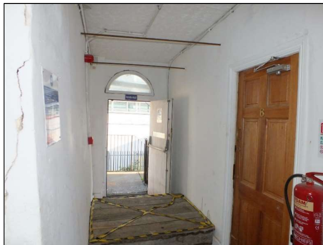
Photo 7. First floor lobby looking east to the rear of the building
