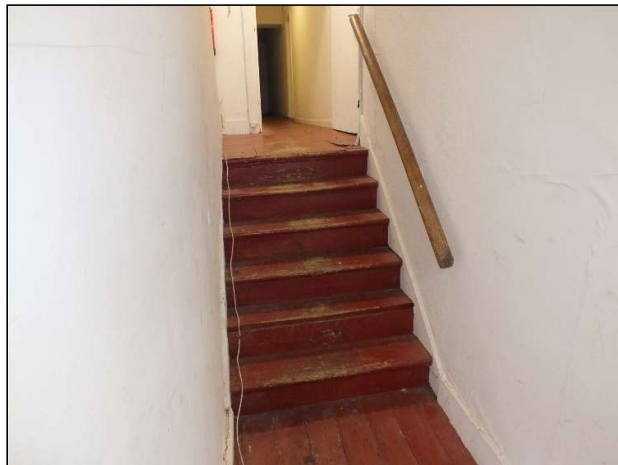
Photo 5. Stairs into first floor lobby
