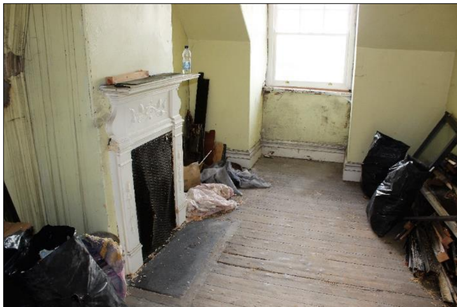
Photo 12: Iron fireplace on second floor
