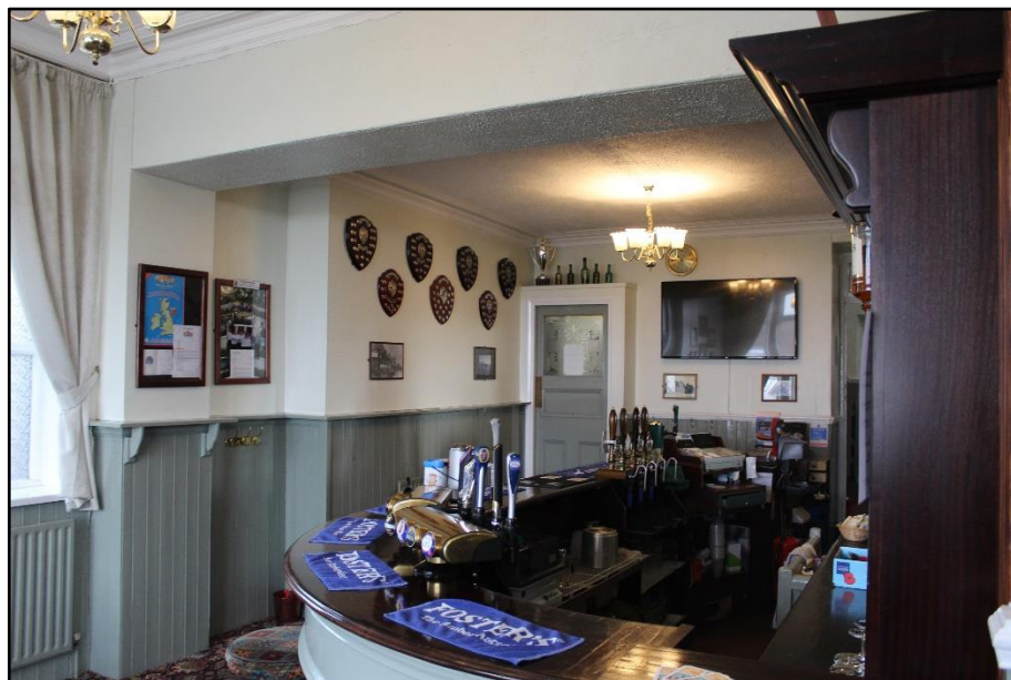
Photo 10: View of bar area showing supporting beam
