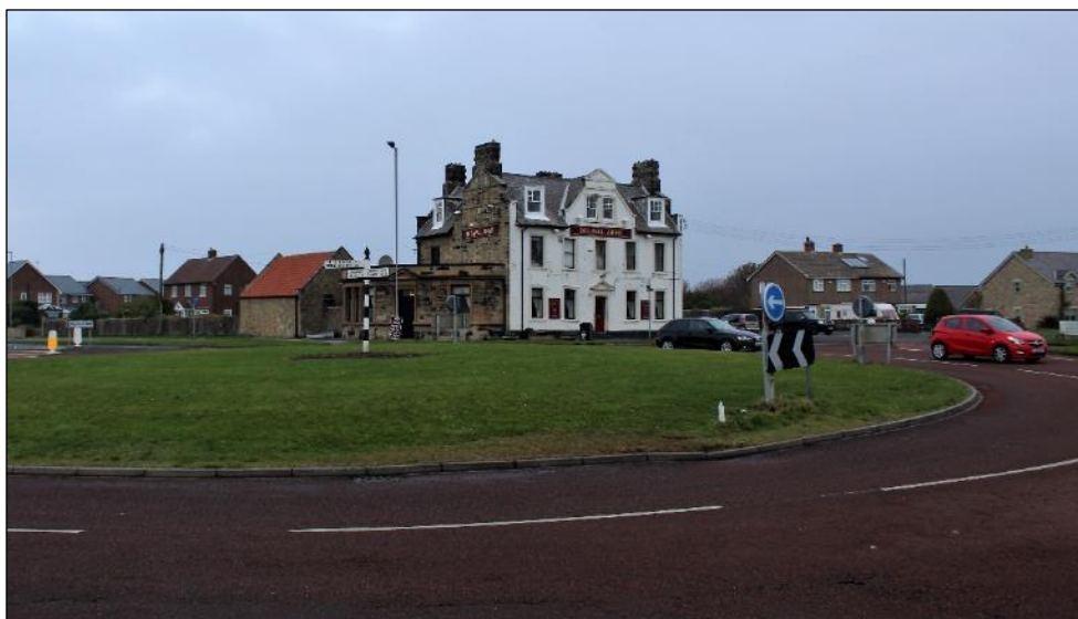
Photo 2: The Delaval Arms, view from south-west
