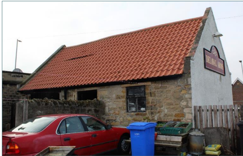
Photo 13: Coach House, view from north
