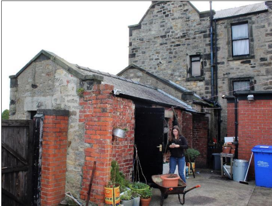
Photo 7: Rear of the Delaval Arms, view from south-east
