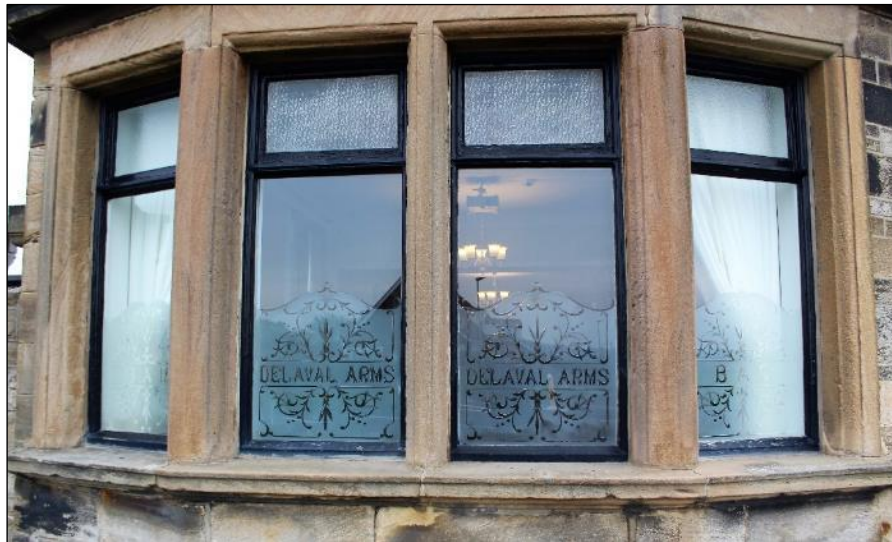
Photo 5: Detail of windows in the western elevation
