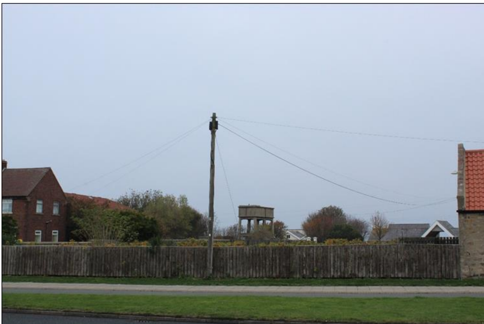
Photo 19: View from Beresford Road to the Grade II* Listed water tower of Roberts Battery
