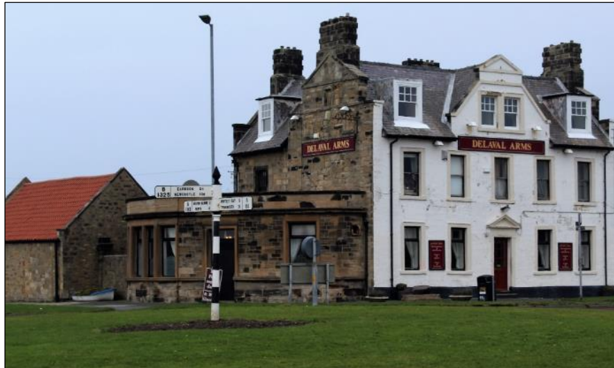
Photo 4: Western elevation, view from south-west
