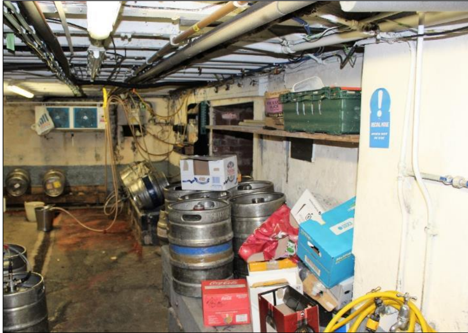
Photo 11: View of the cellar
