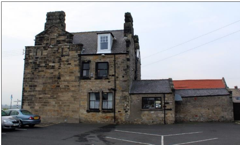
Photo 6: Eastern elevation of the Delaval Arms
