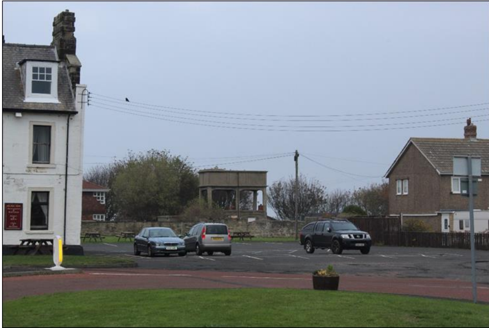
Photo 18: View from East End to the Grade II* Listed water tower and boundary wall of Roberts Battery
