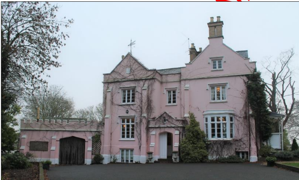
Photo 1: Western elevation of Woodlands Castle
