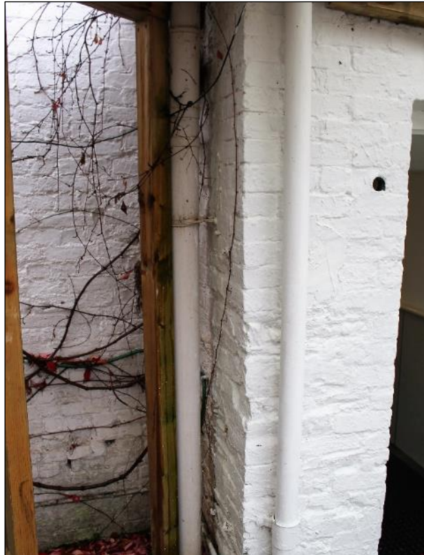
Photo 6: Brick porch and rough pointing, southern elevation of Woodlands Castle
