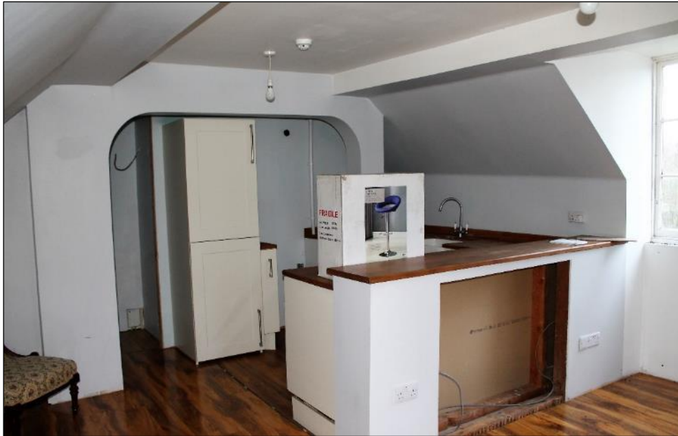
Photo 16: Second floor room in process of being modernised
