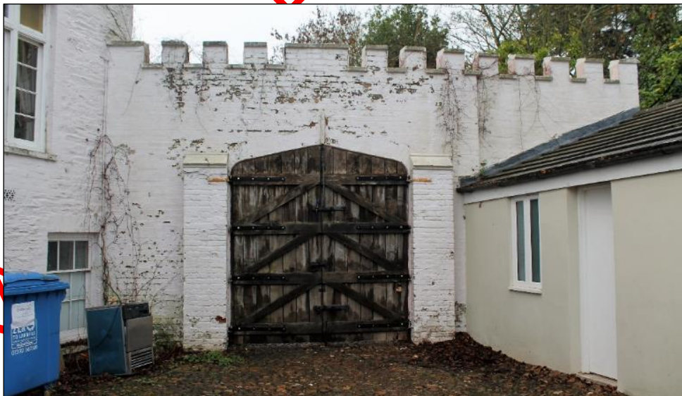
Photo 7: Inside of courtyard gateway, eastern elevation
