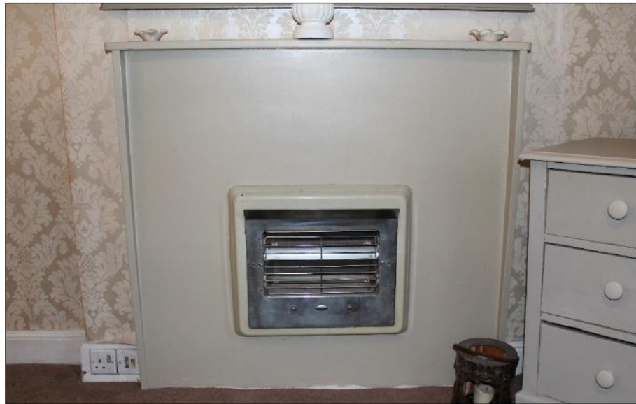
Photo 12: Gas fire insertion into possible former fireplace, first floor
