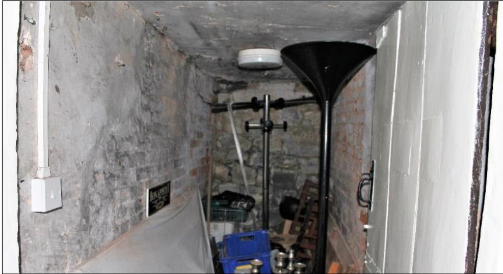
Photo 14: Stone and brick walls in basement store-room
