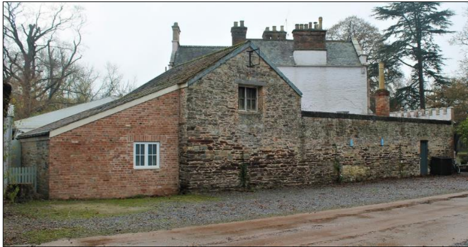
Photo 8: North facing elevation of stable buildings
