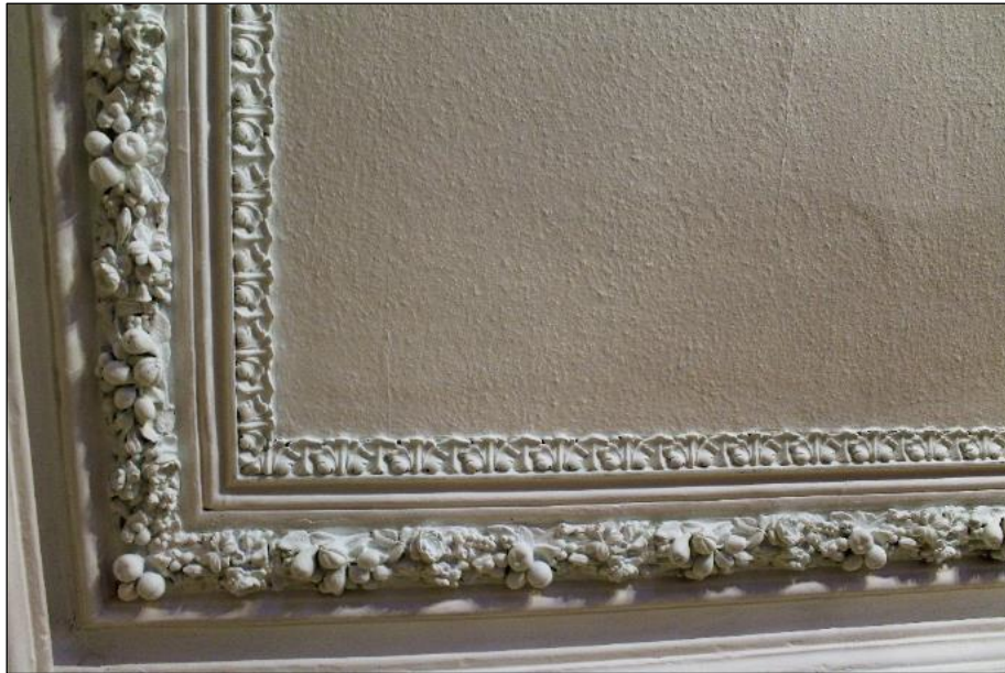
Photo 10: Decorated plaster moulding, ground floor
