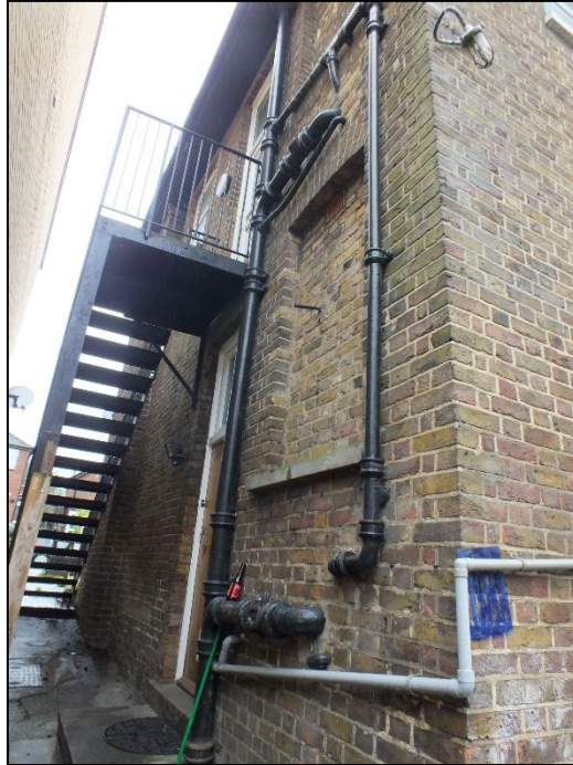
Photo 3. 4-6 Ealing Road, northern elevation (looking south-east)
