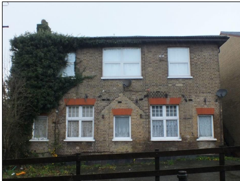
Photo 1. Nos 4-6 Ealing Road front elevation
