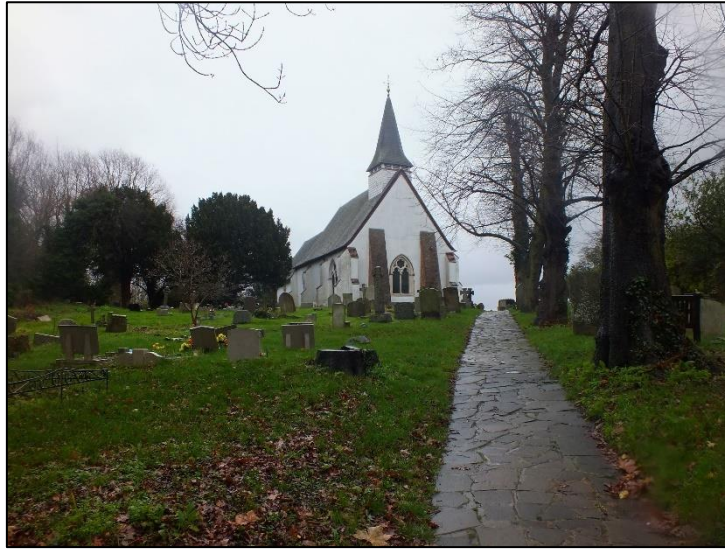
Photo 14. Church of St Mary [AB 7; Grade I Listed], looking south-east
