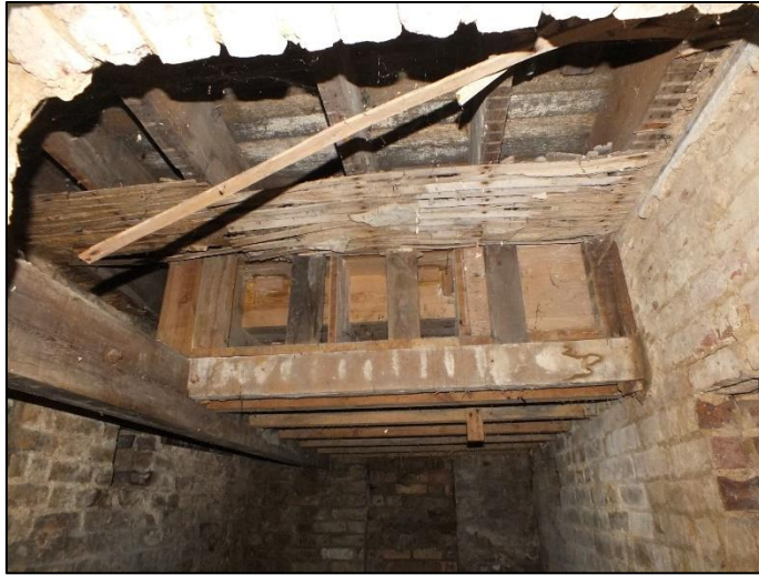
Photo 7. Lowered ceiling in basement
