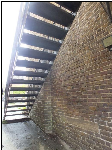
Photo 4. Northern elevation, infilled opening
