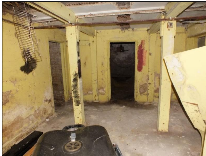
Photo 8. Central room in basement
