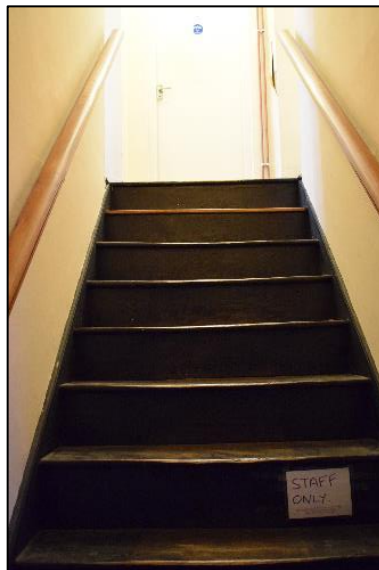
Photo 3: The original stairs from the entrance lobby
