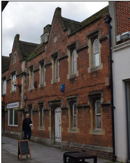
Photo 1: The east elevation from the north-east, taken from Magdalene Lane
