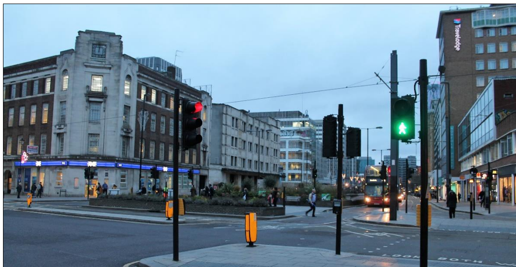
Photo 3: View towards northern underpass portal from junction of George Street and A212
