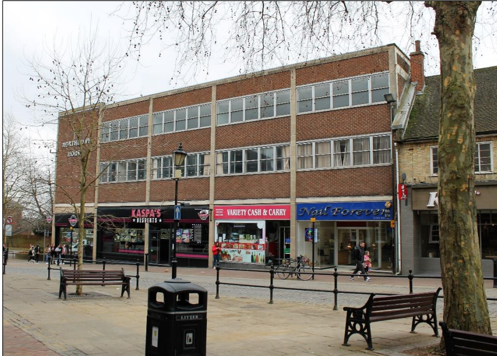
Photo 4: General shot of Northdown House (northern elevation)
