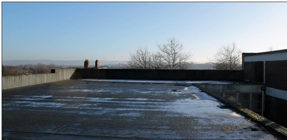
Photo 3: View east from Northdown House roof
