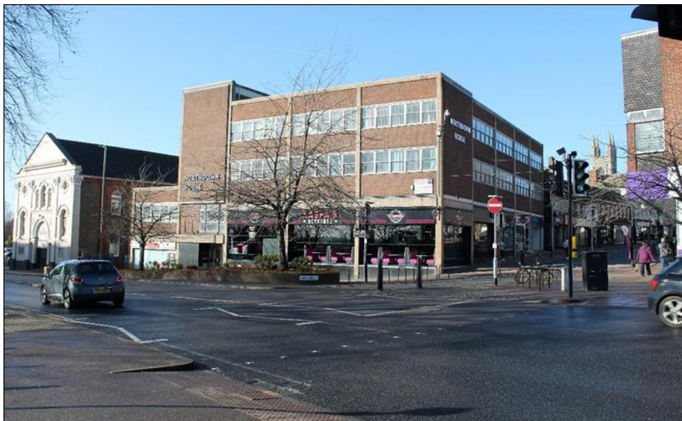
Photo 5: Northdown House, viewed from Wellesley Road (Baptist Church left of picture)
