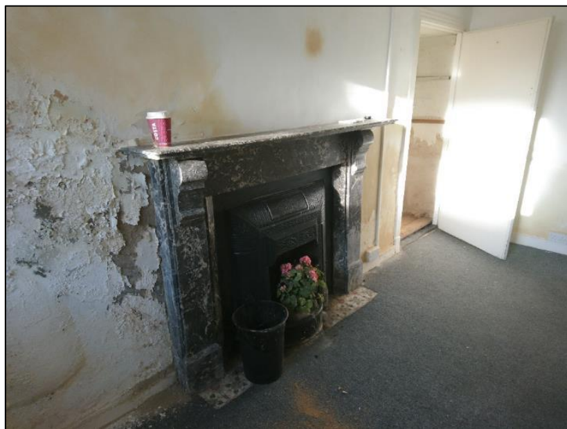
Photo 10. Fireplace in Basement front room
