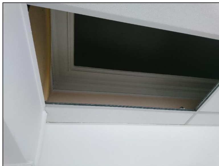
Photo 7. Showing coving behind modern suspended ceiling. Decorative door arch also visible
