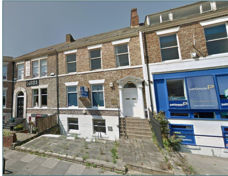
Photo 14. Oblique shot showing front elevation (courtesy of Google)
