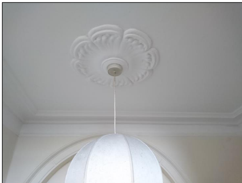
Photo 12. Ground Floor ceiling rose at door to base of stairs
