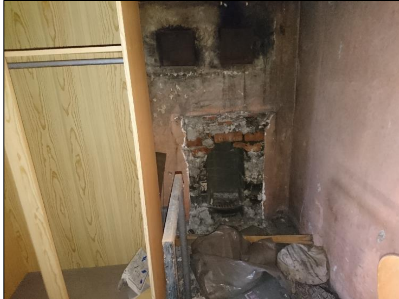
Photo 2. Showing fireplace in front attic room
