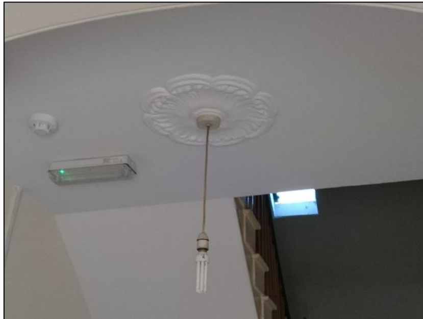
Photo 13. First Floor ceiling rose at landing
