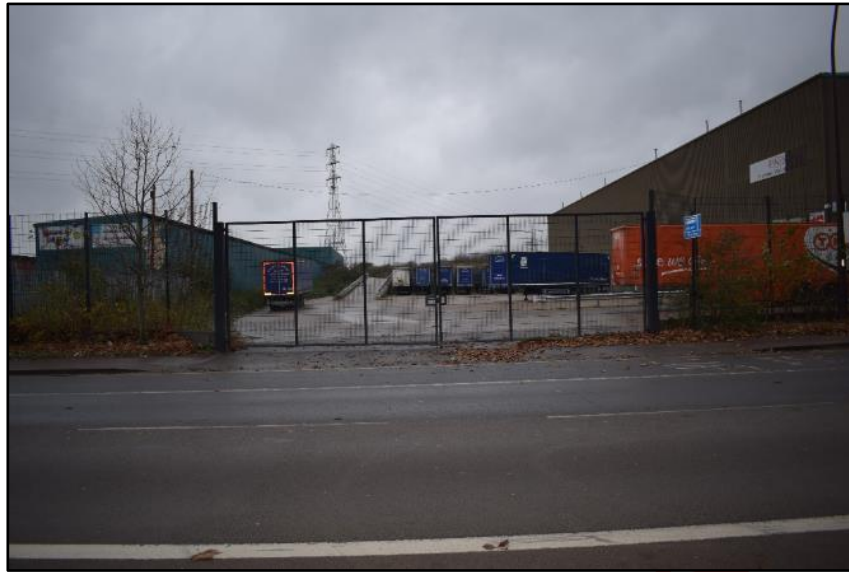
Photo 4: View of access ramp at southern end of raised quayside, looking west
