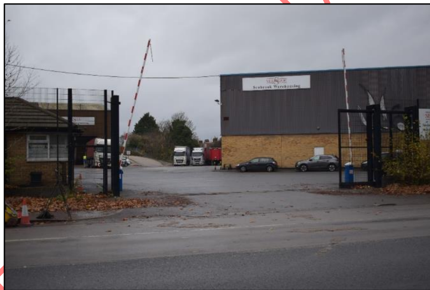
Photo 5: View to access ramp at northern end of raised quayside, looking west
