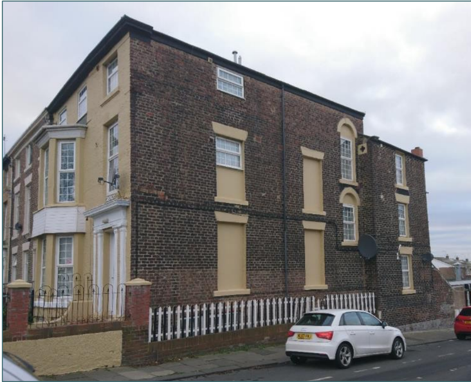
Photo 2. North-east elevation showing added wing towards rear
