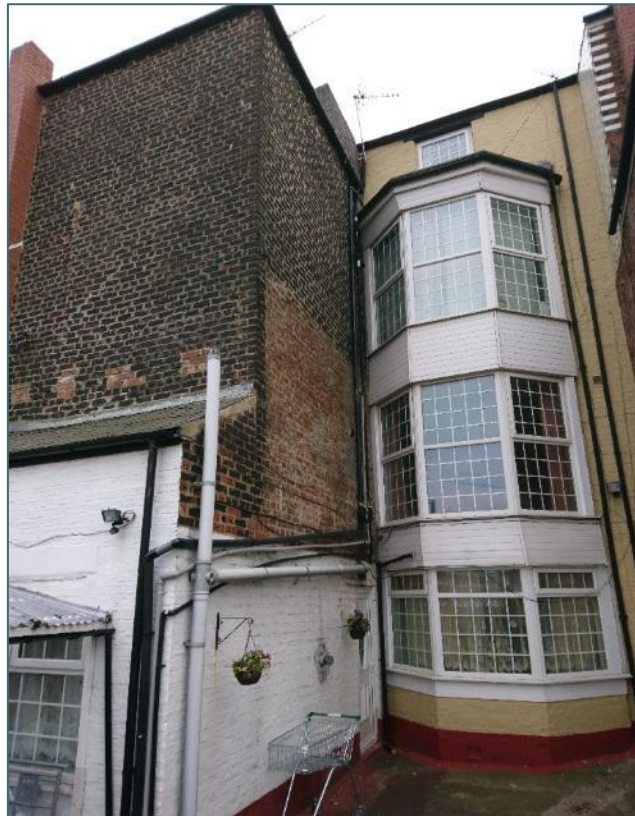
Photo 3. Rear (north-west) elevation
