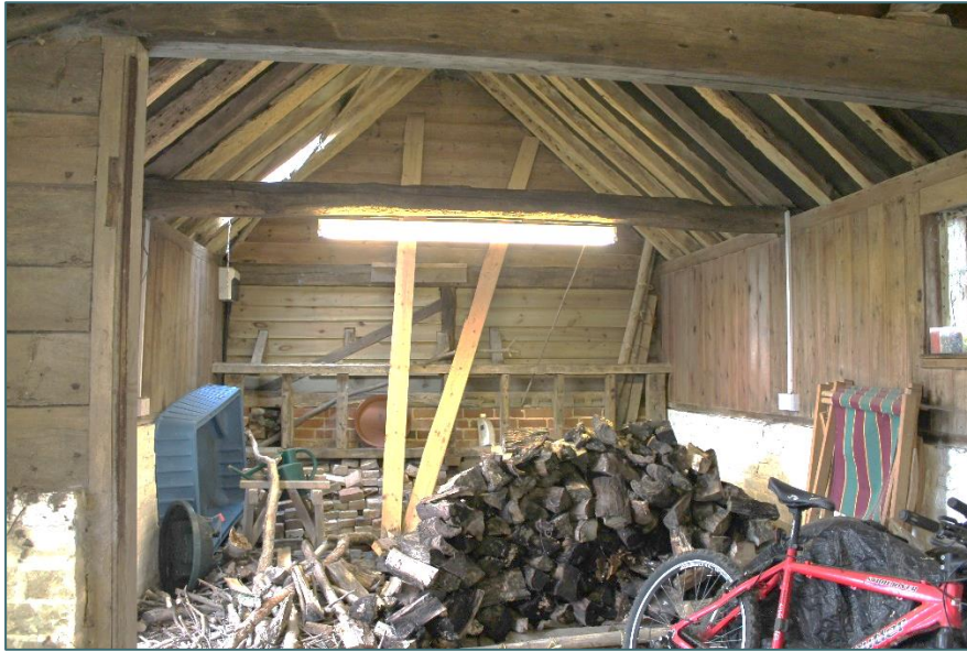
Photo 13. Showing interior of SE Outbuilding. Note modern brick, panels and rafters
