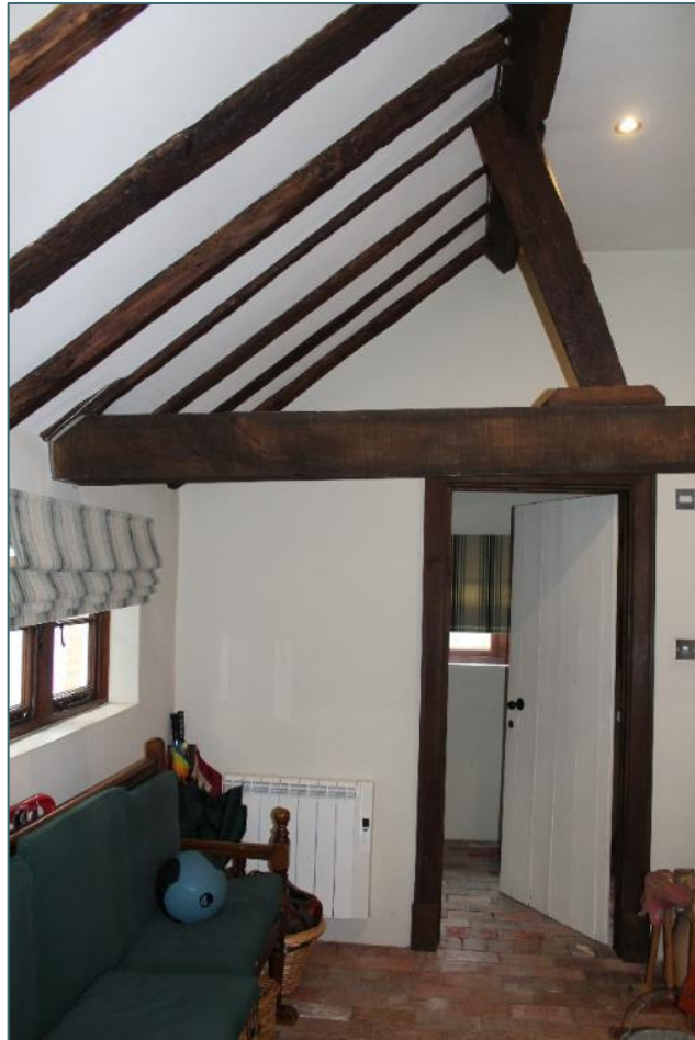
Photo 6. Boot Room and WC
