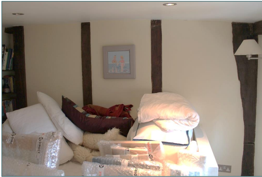
Photo 7. Bedroom 5 looking East
