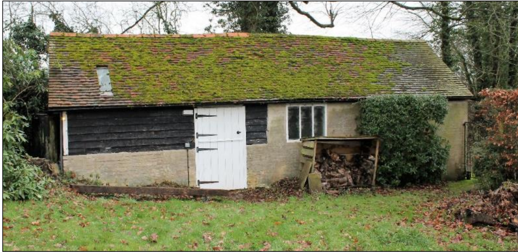
Photo 11: South East Outbuilding (West elevation)
