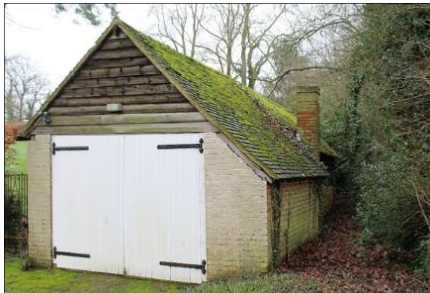
Photo 12. South East Outbuilding (South elevation)
