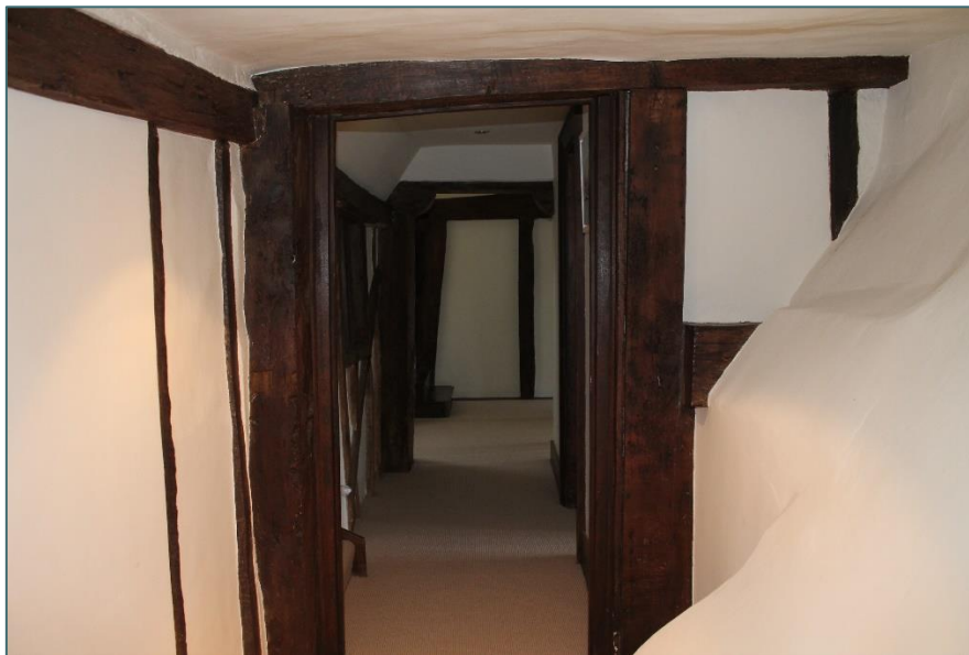
Photo 8. Bedroom 5 with the original chimney breast at the right of shot
