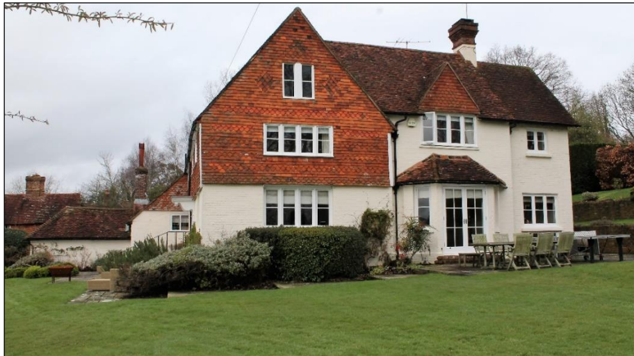
Photo 1: General Site Shot of Doubleton Farmhouse (East Elevation)
