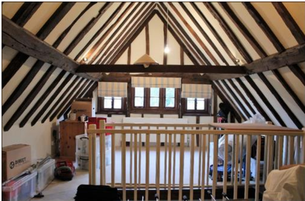
Photo 10: Existing Attic space
