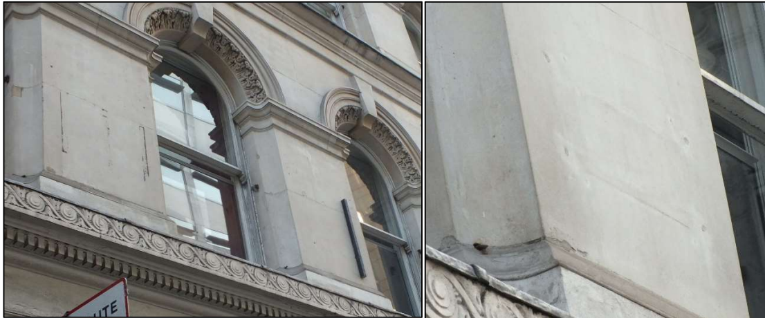
Photo 4. Details of previous fixings
