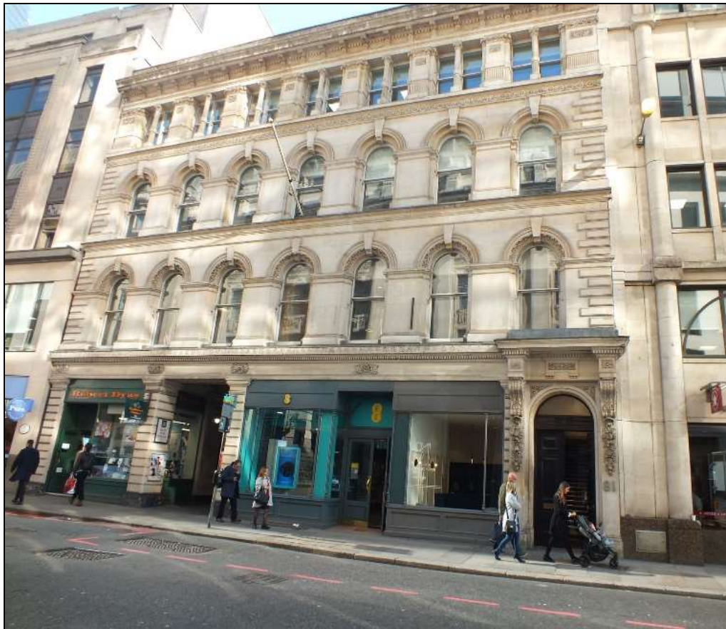
Photo 1. Front façade of 81-82 Gracechurch Street
