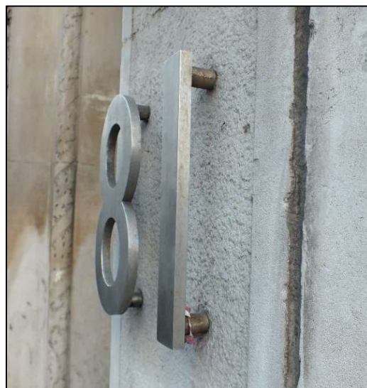
Photo 3. Detail of existing number fixing
