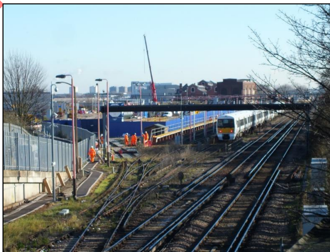
Photo 25. View from railway bridge at Plumstead High Street.
