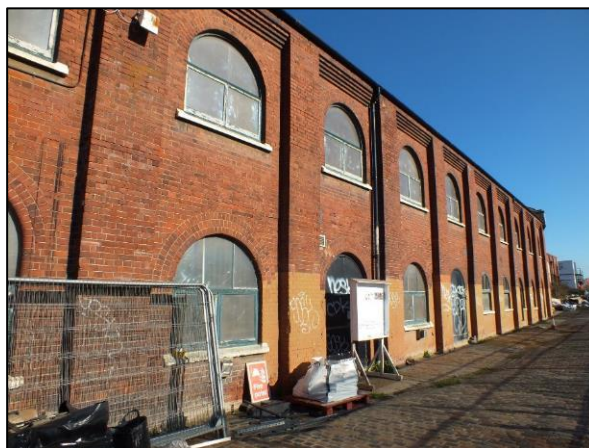
Photo 21. Southern elevation, western end
