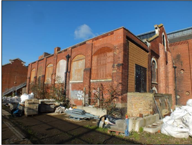
Photo 14. Southern elevation, eastern end
