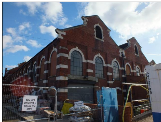
Photo 17. Western façade of the depot building, northern side
