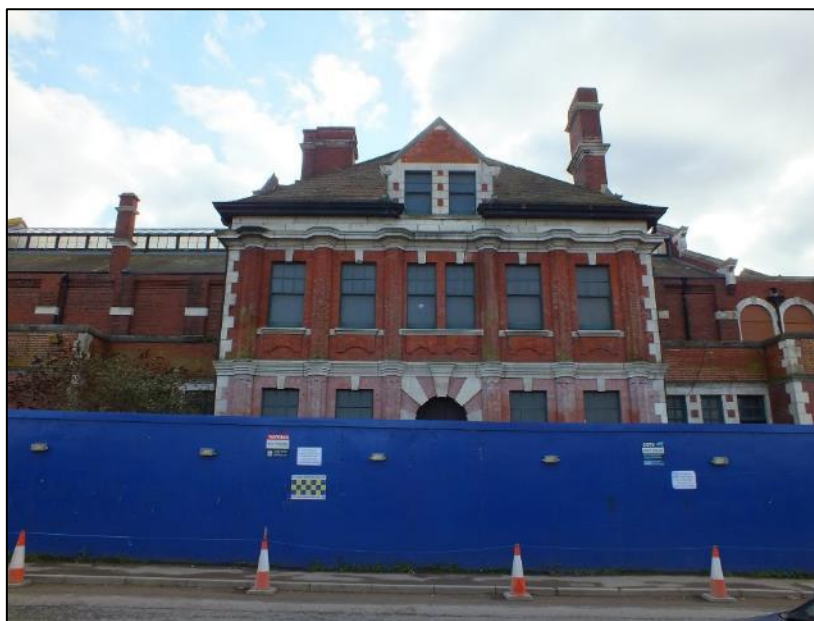
Photo 4. Northern elevation (centre): Office frontage
