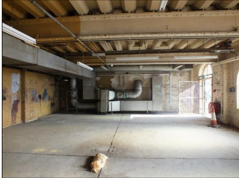
Photo 22. Hall 5, Ground floor (Direction E)
