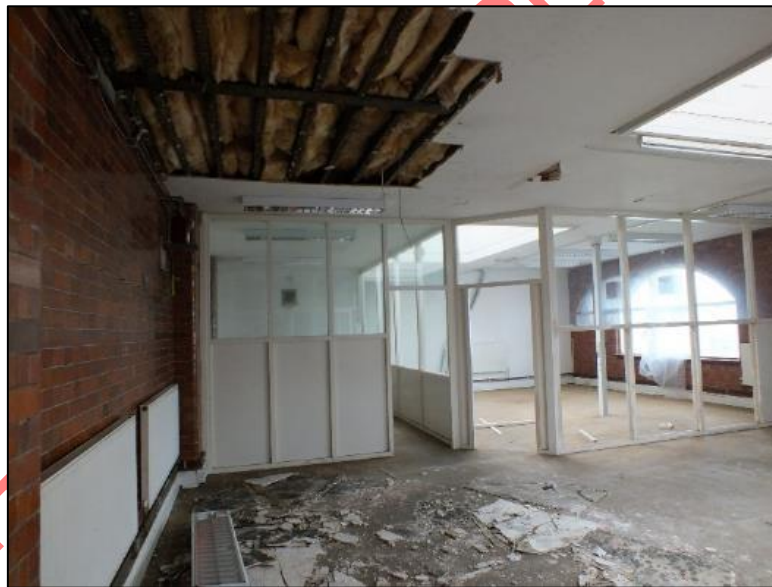
Photo 7. Interior of ancillary office
