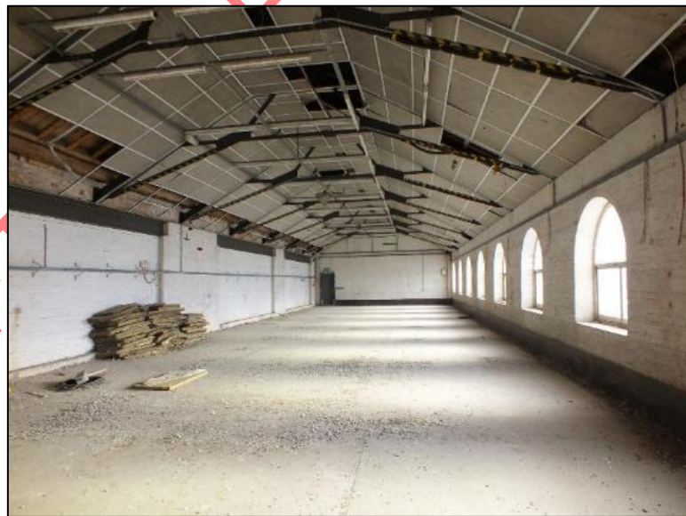
Photo 23. Hall 5, First floor (Direction E)
