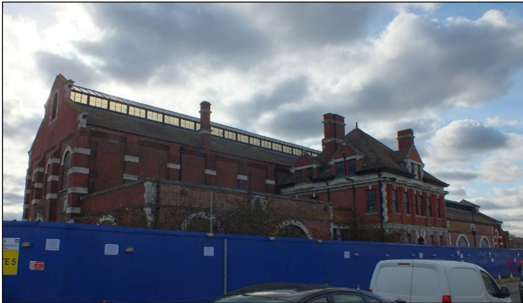
Photo 8. Northern elevation, eastern end
