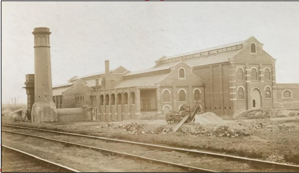
Plate 8. Photograph of southern and eastern elevations of power station /depot building [AB 21], c. 1923 (Greenwich Heritage Centre)
