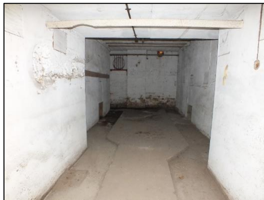
Photo 11. Basement below Generator Hall
