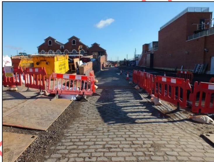
Photo 3. Cobbled surface in south of the site (direction E)
