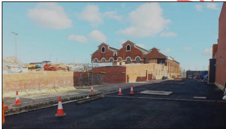
Photo 20. Western end of depot building, including retaining wall for ramped access
