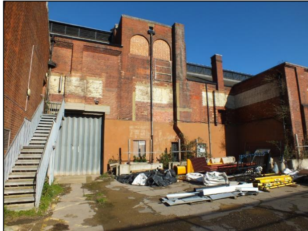
Photo 24. Southern elevation, central section
