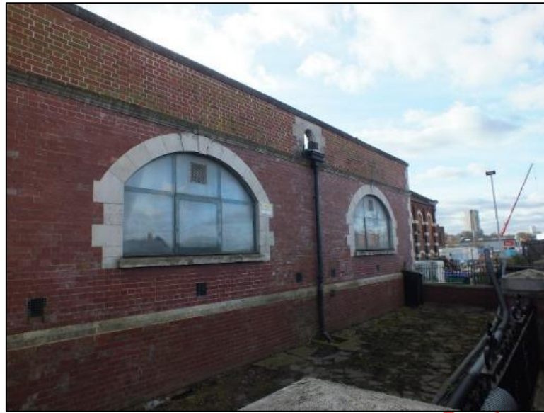
Photo 6. Exterior of ancillary office
