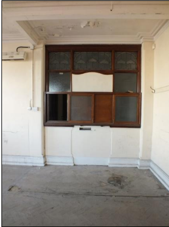
Photo 5. Glazed Partition / reception area
