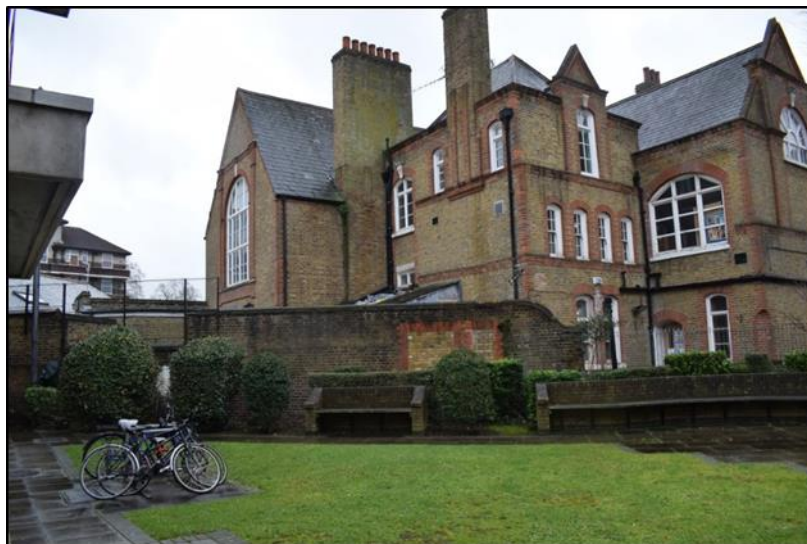
Photo 6: View of boundary wall and Macbeth Centre, looking southwest
