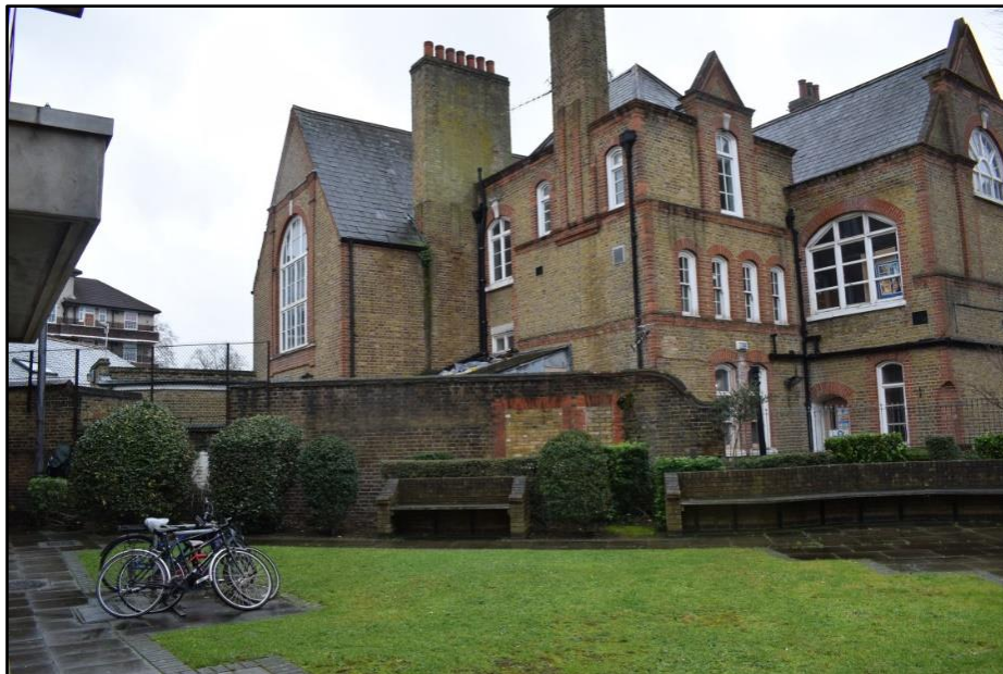
Photo 14: View towards the Macbeth Centre from Princess Mews, looking southwest
