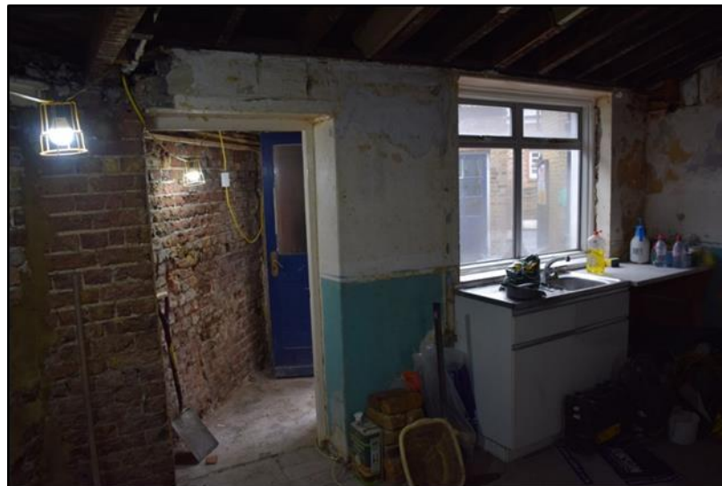
Photo 9: interior view of lean-to entrance way, looking east
