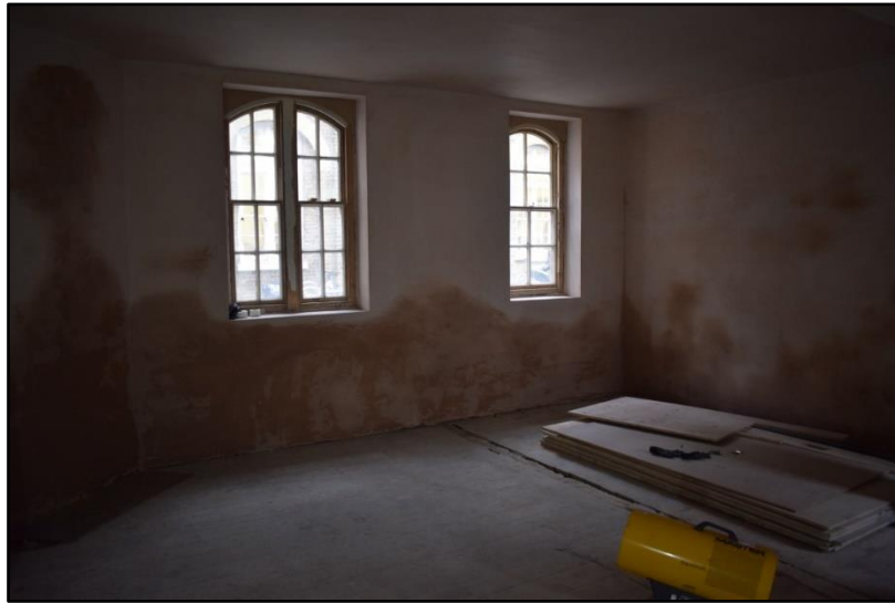
Photo 10: Internal view of western room, looking west
