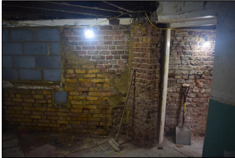
Photo 5: Phases of brick repair and infilling in boundary wall, looking northeast
