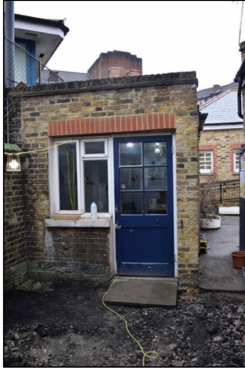
Photo 7: View of detached room, looking southeast
