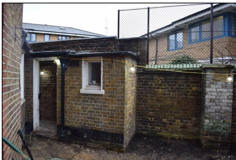
Photo 4: View of entrance to managers rooms and boundary wall, looking northeast
