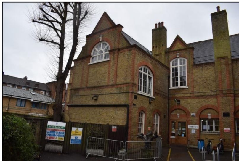
Photo 2: 19 th Century former school buildings, looking southeast towards managers accommodation
