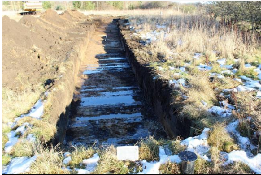
Photo 9: Trench 5, looking west (1m & 2m scales)
