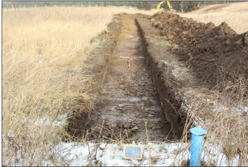
Photo 17: Trench 9, looking north (1m & 2m scales)
