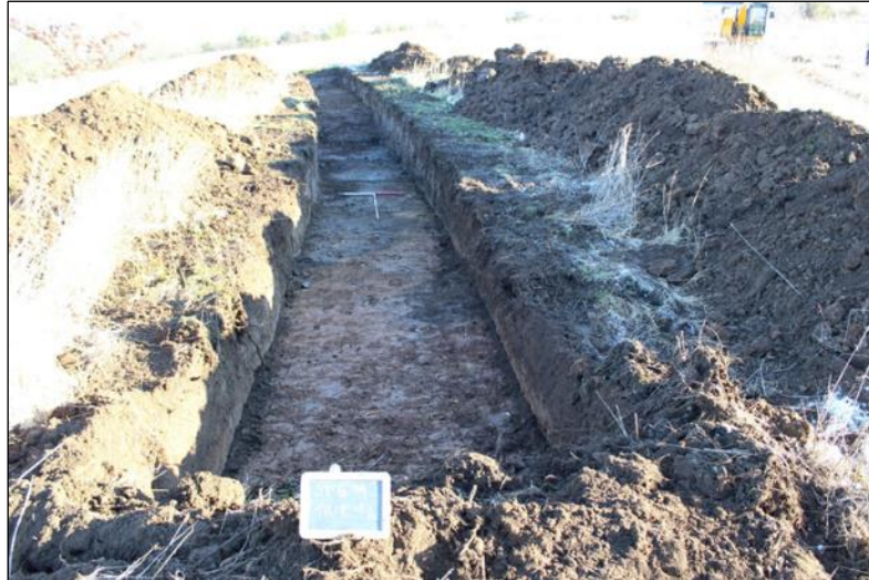
Photo 15: Trench 8, looking north-east (1m & 2m scales)
