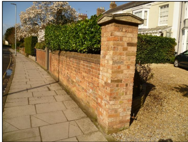
Photo 2: The front boundary wall of 66 Staplegrove Road
