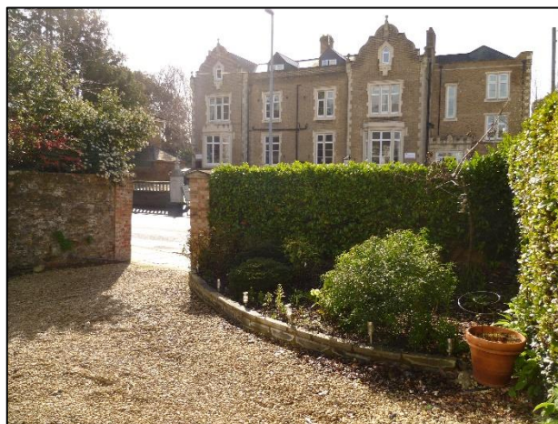
Photo 3: View from 66 Staplegrove Road towards the boundary wall & Staplegrove Road
