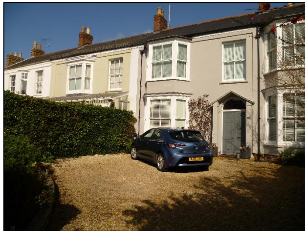
Photo 1: 66 Staplegrove Road (right), from the driveway entrance
