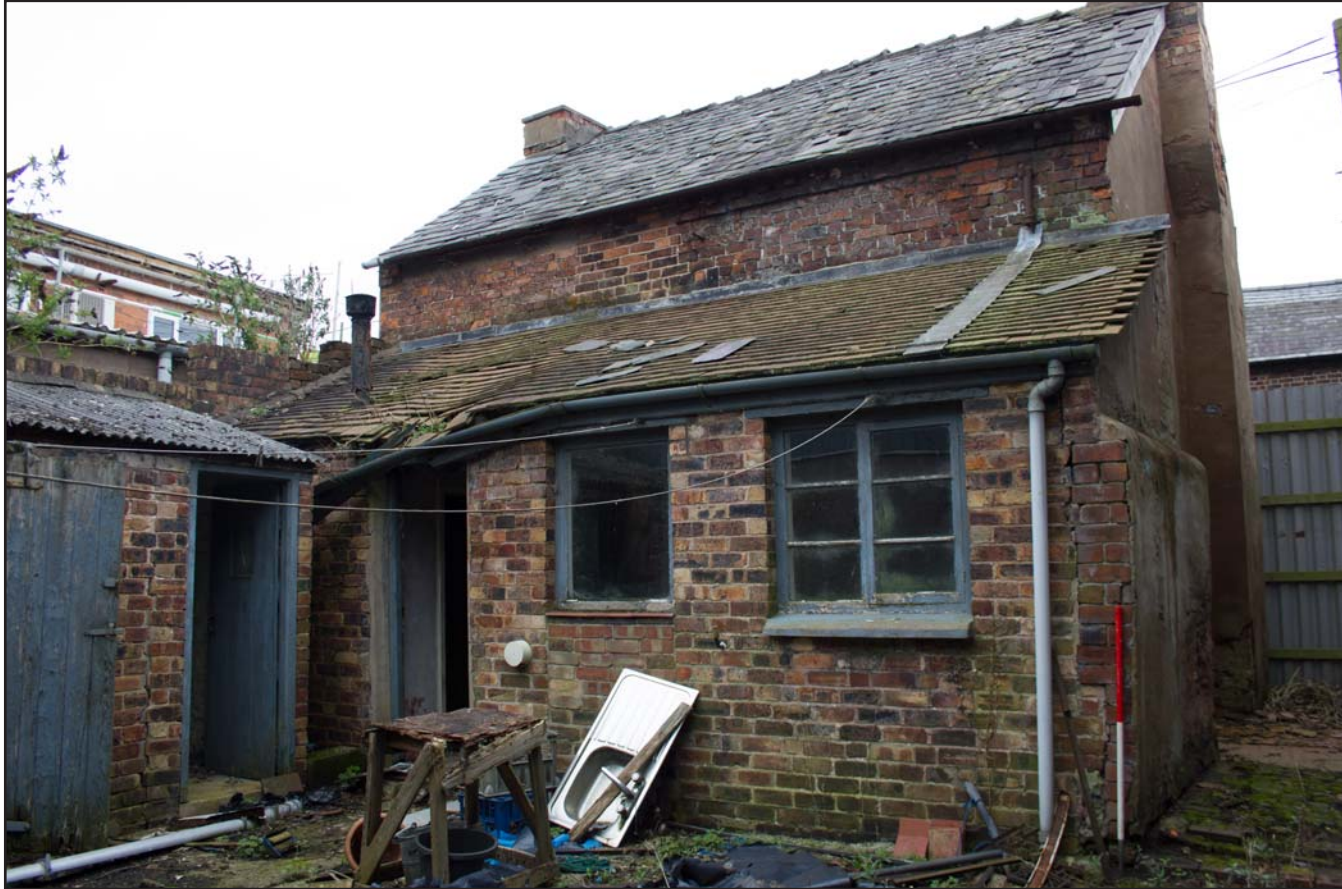
Plate 05: Northwest facing external elevation, from the west. Scale 1.0m.
