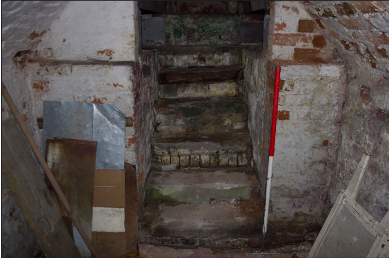
Plate 20: Room 6 (Cellar) showing steps, from the southeast. Scale 1.0m.
