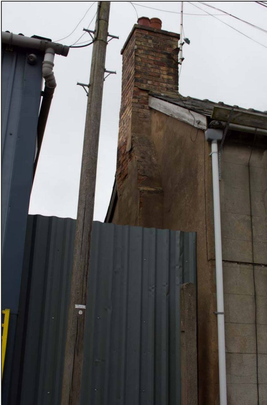
Plate 03: Southwest facing external elevation, from the south.
