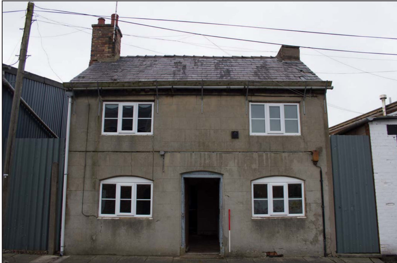
Plate 01: Southeast facing principle external elevation, from the southeast. Scale 1.0m.
