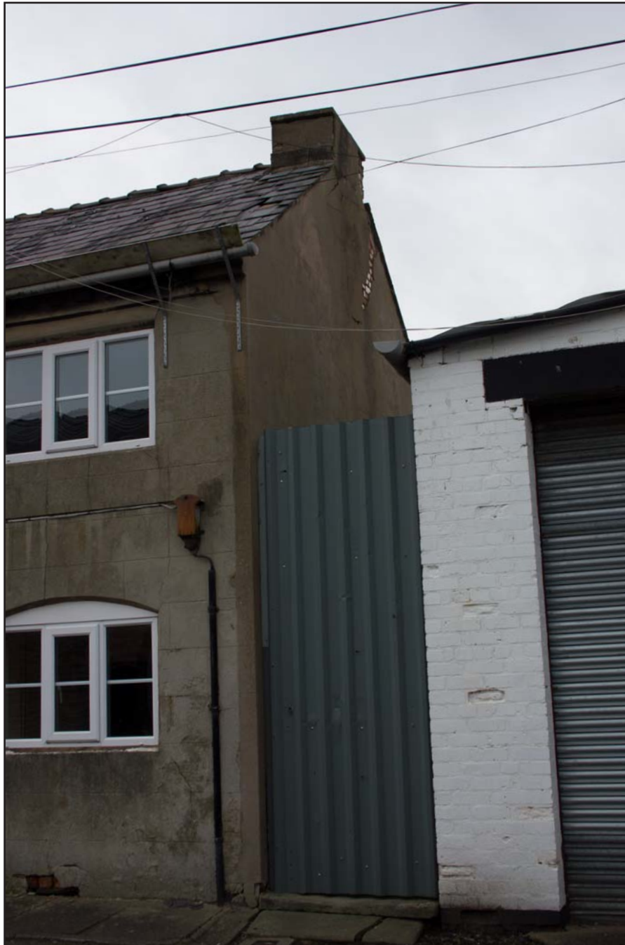
Plate 07: Northeast facing external elevation, from the east.
