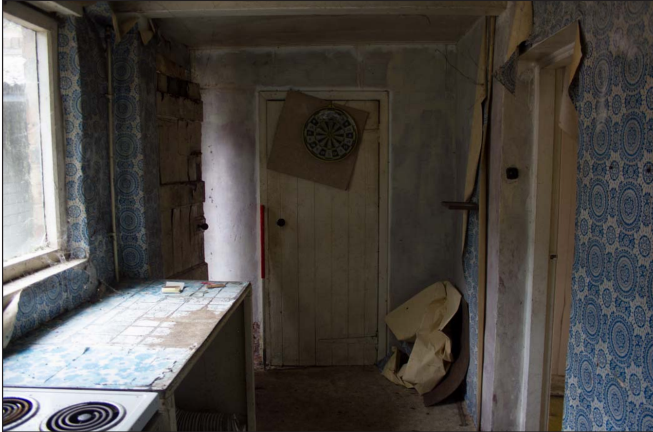
Plate 15: Room 3 (Kitchen), from the southwest. Scale 1.0m.
