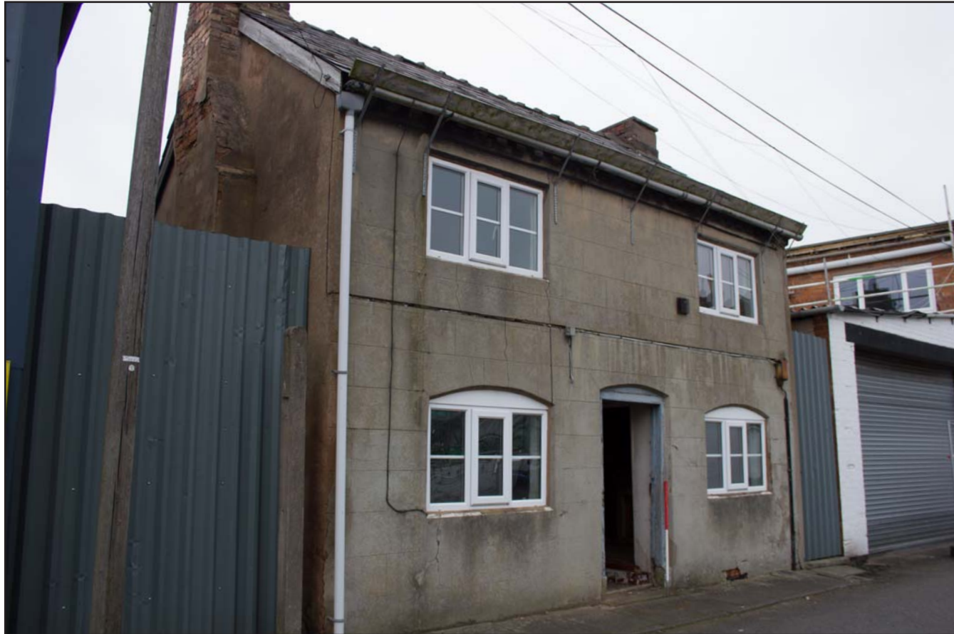
Plate 02: Southeast and southwest facing external elevations, from the south. Scale 1.0m.
