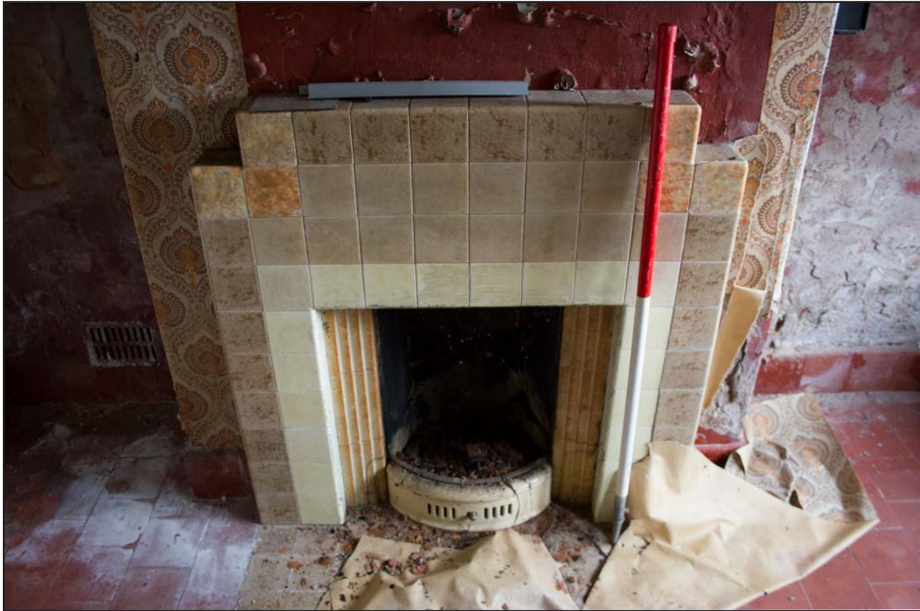
Plate 14: Room 2 (Parlour) showing fireplace, from the southwest. Scale 1.0m.
