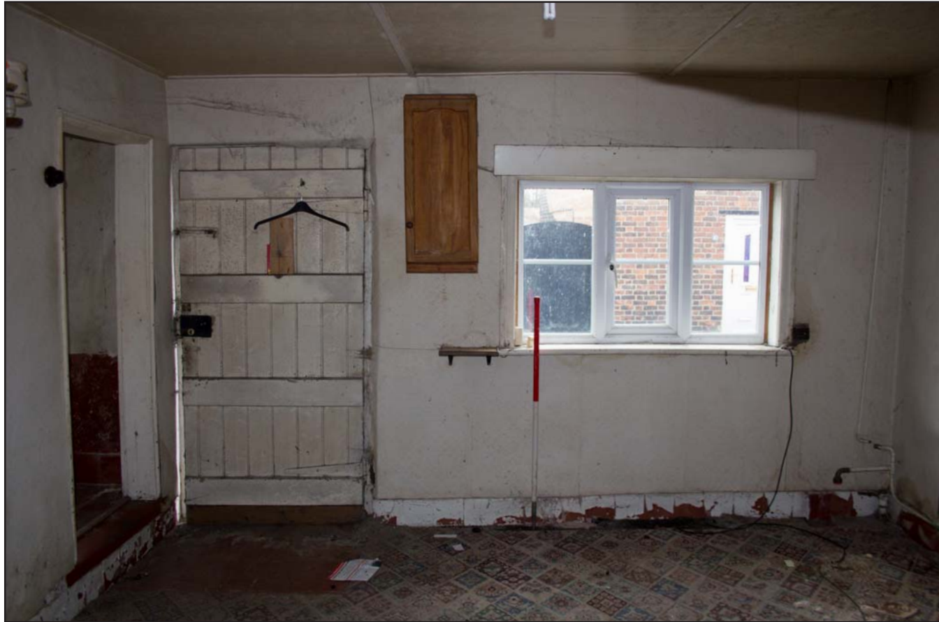
Plate 09: Room 1 (Living Room), from the northwest. Scale 1.0m.
