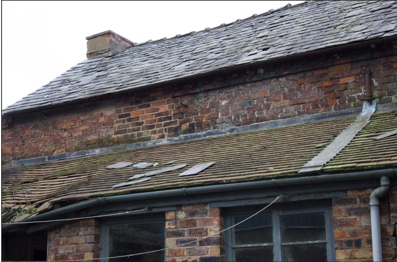
Plate 06: Northwest facing external elevation showing blocked windows, from the west.
