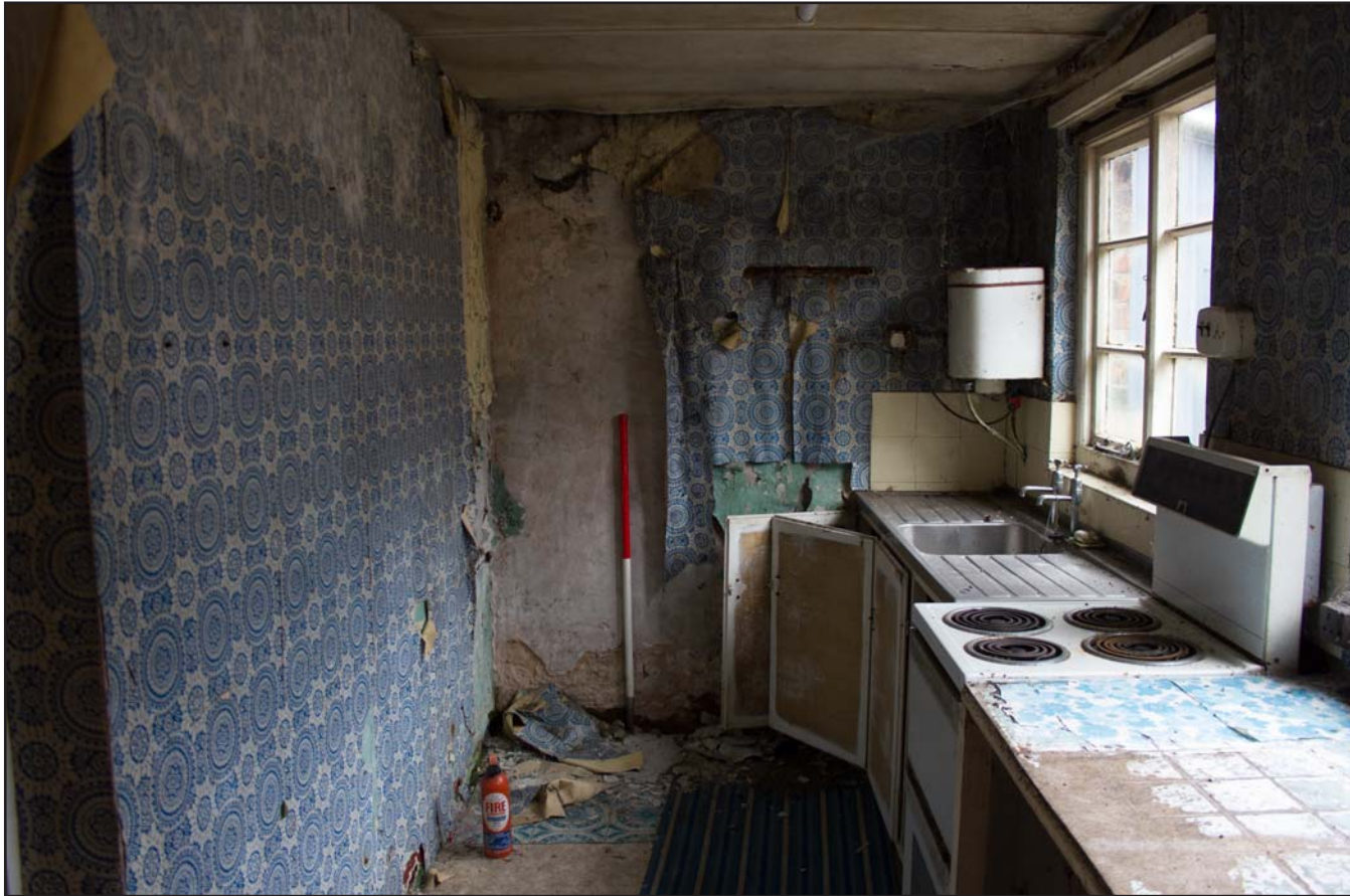
Plate 16: Room 3 (Kitchen), from the northeast. Scale 1.0m.
