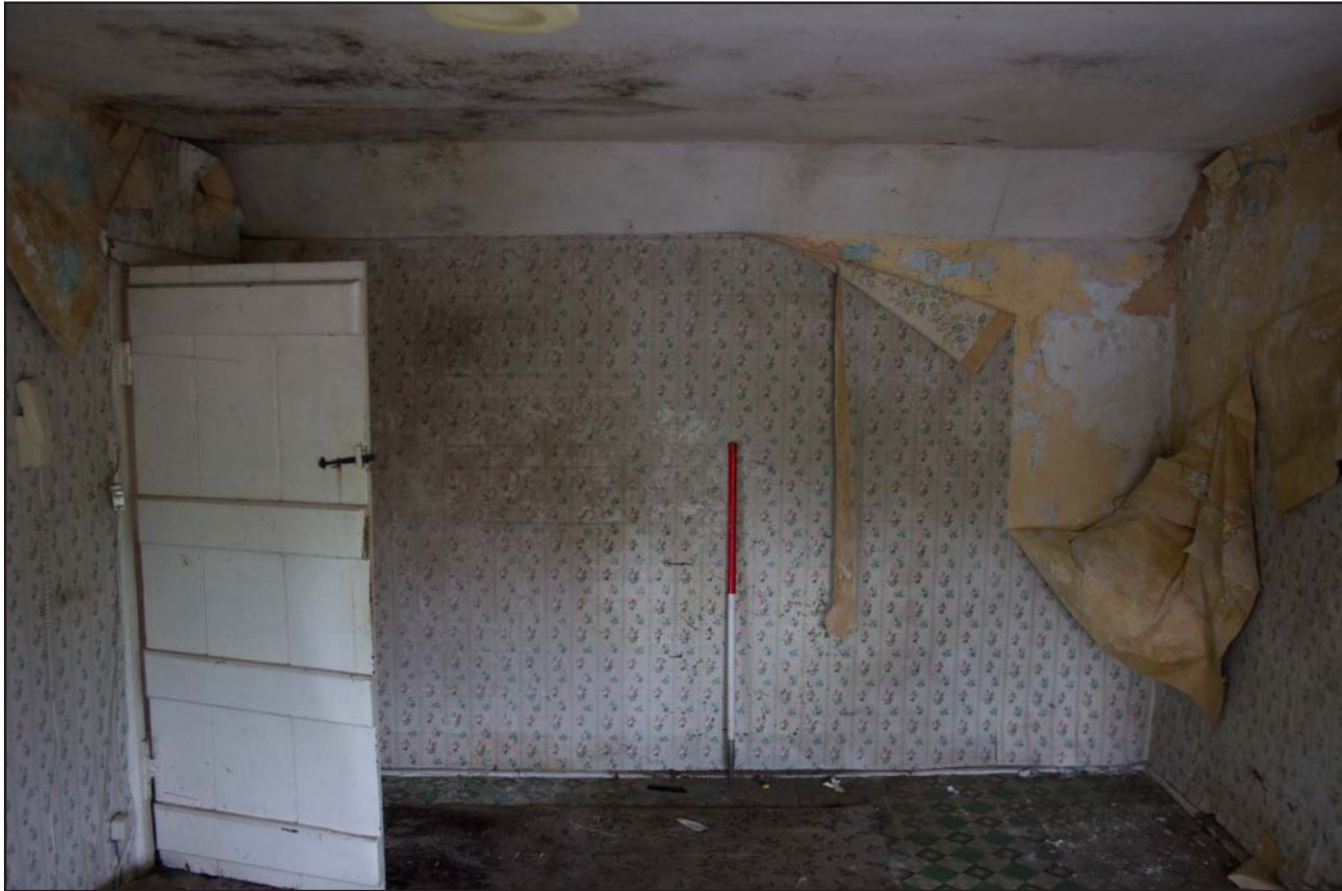
Plate 22: Room 8 (Bedroom), from the southeast. Scale 1.0m.
