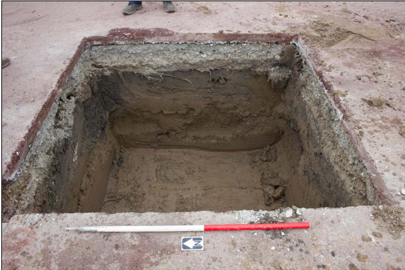
Plate 24: Parabol Base 3 for Parade Ring Canopies at Chester Racecourse, Chester - from the west - 1.00m scale
