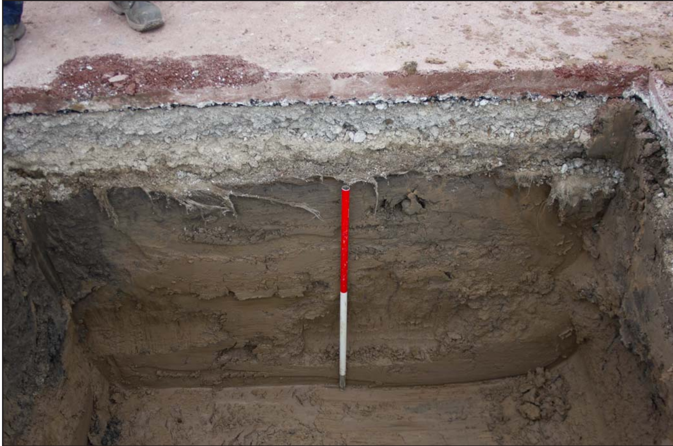
Plate 25: Parasol Base 3 for Parade Ring Canopies at Chester Racecourse, Chester - from the west - 1.00m scale
