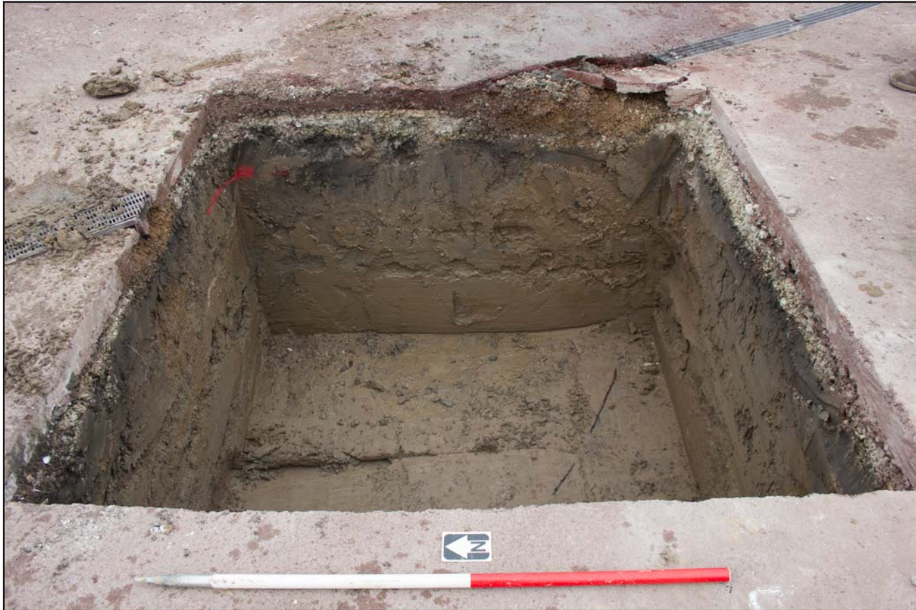
Plate 26: Parasol Base 4 for Parade Ring Canopies at Chester Racecourse, Chester - from the west - 1.00m scale
