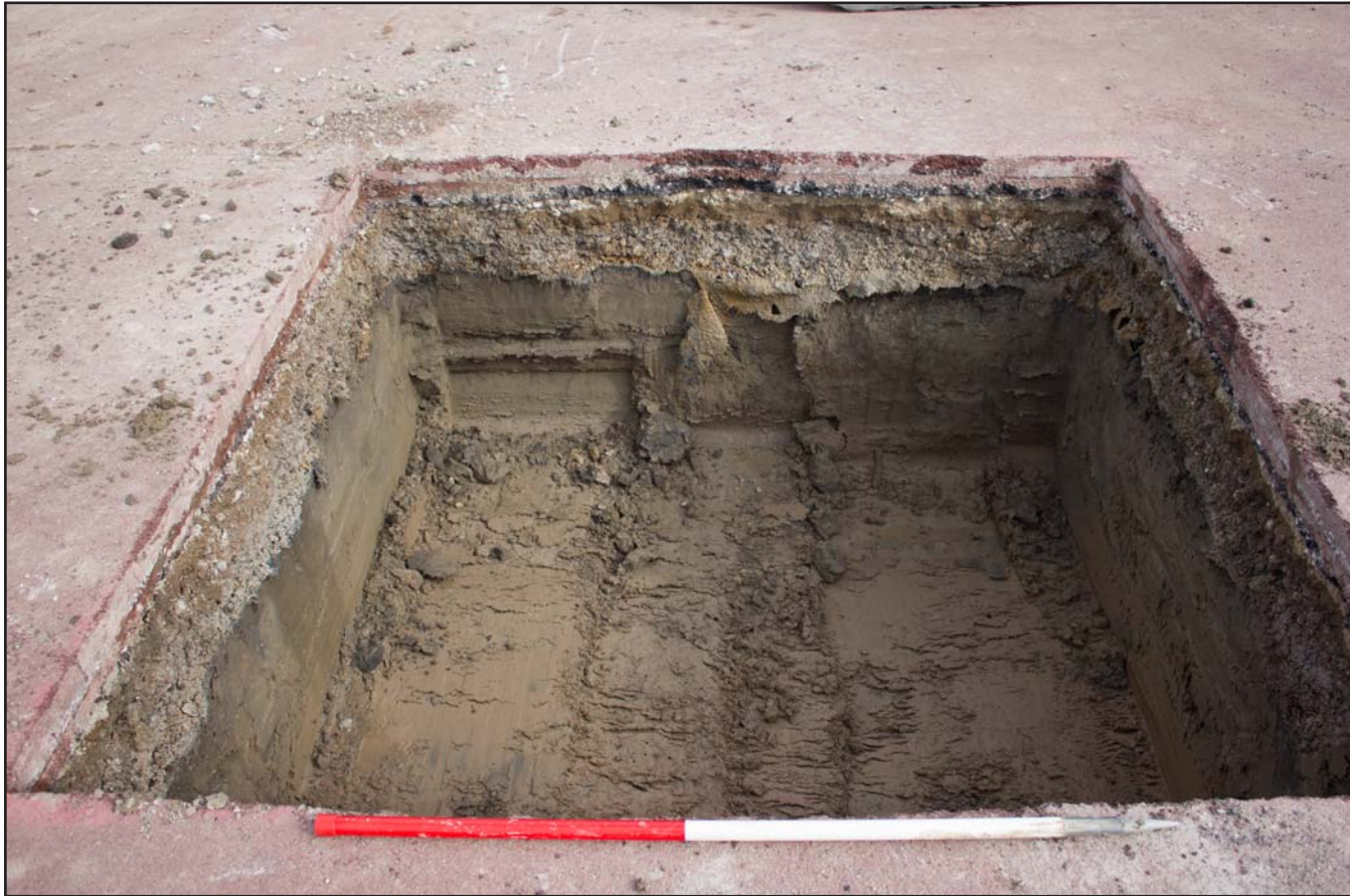
Plate 42: Parasol Base 12 for Parade Ring Canopies at Chester Racecourse, Chester - from the southwest - 1.00m scale
