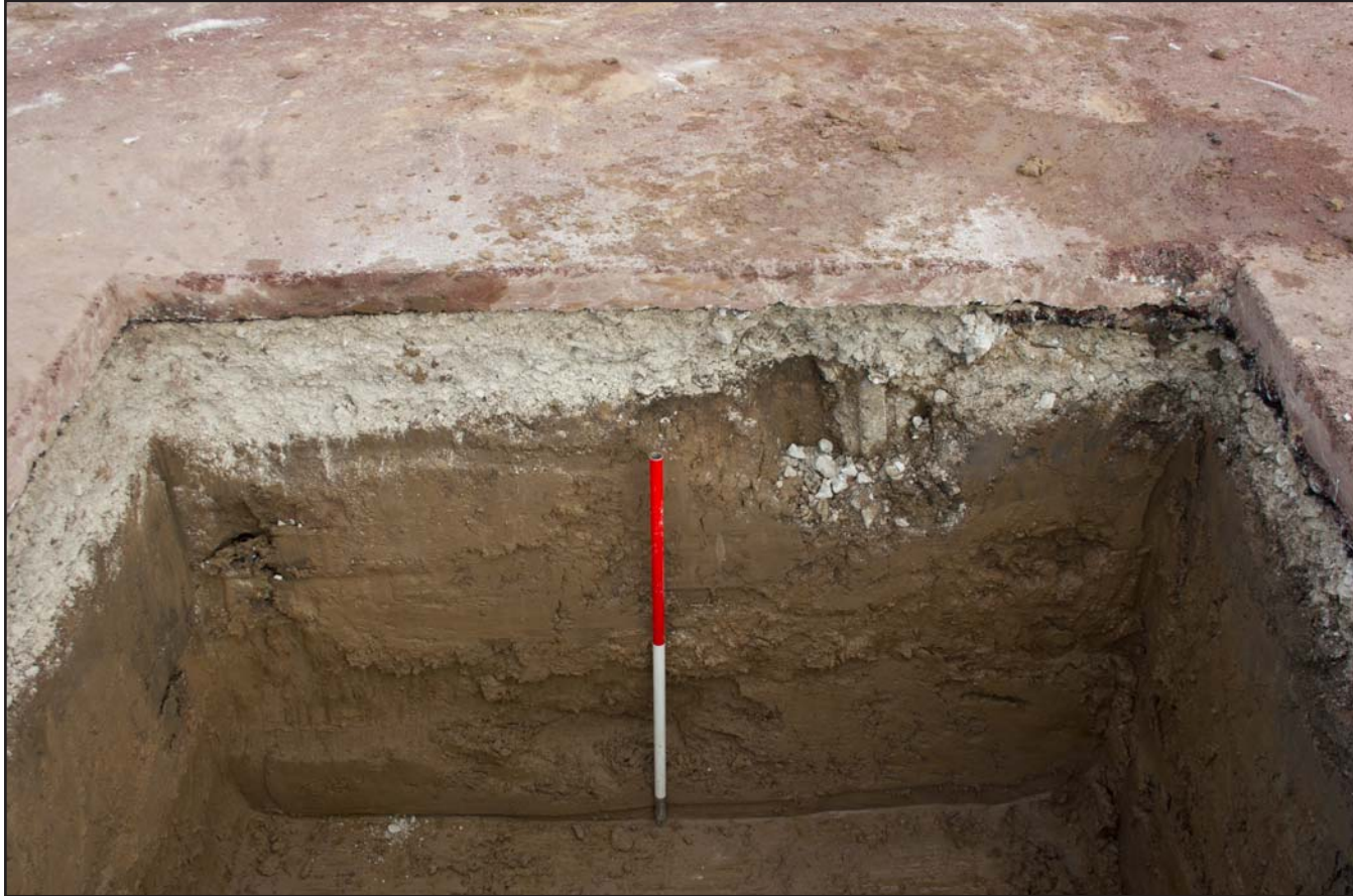
Plate 31: Parasol Base 6 for Parade Ring Canopies at Chester Racecourse, Chester - from the west - 1.00m scale
