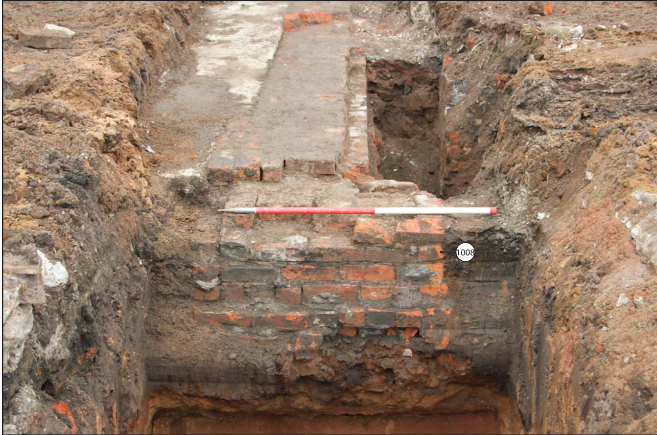
Plate 15: Trench 3 showing red-brick wall foundations (1008), from the west. Scale 1.0m.
