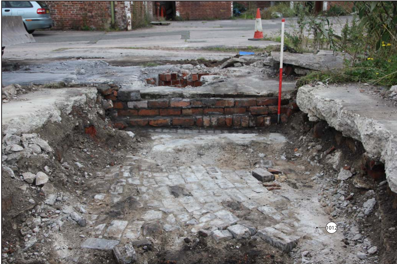
Plate 19: Trench 3 showing external brick surface (1012), from the west. Scale 1.0m.
