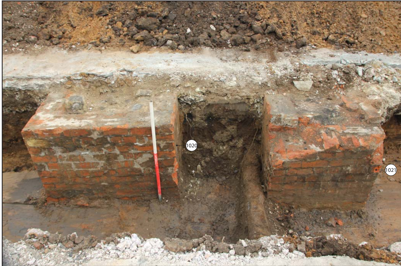
Plate 04: Trench 1 showing brick-built girder bases (1020) and (1021), from the west. Scale 1.0m.
