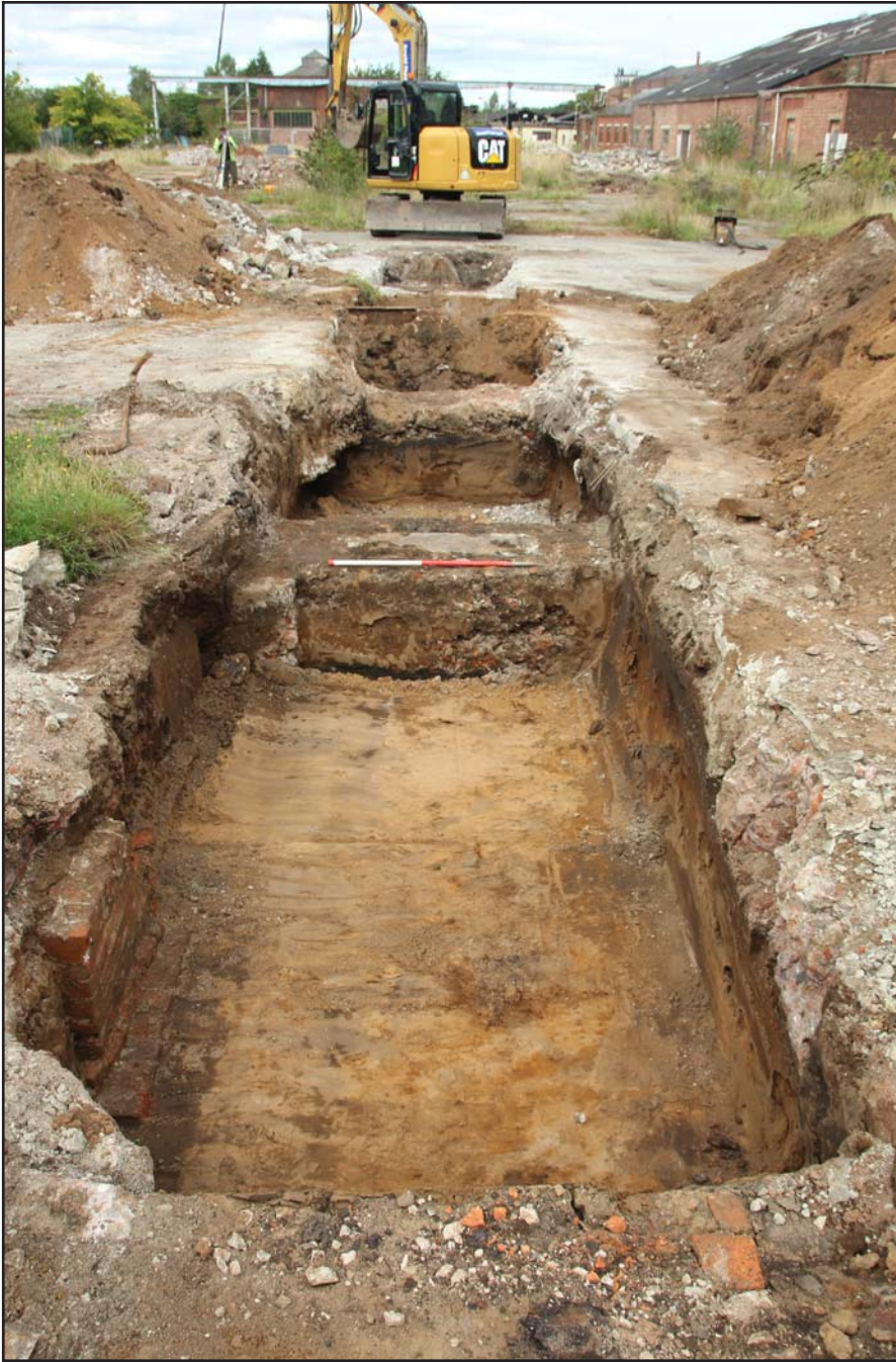
Plate 06: Trench 2, from the south. Scale 1.0m.
