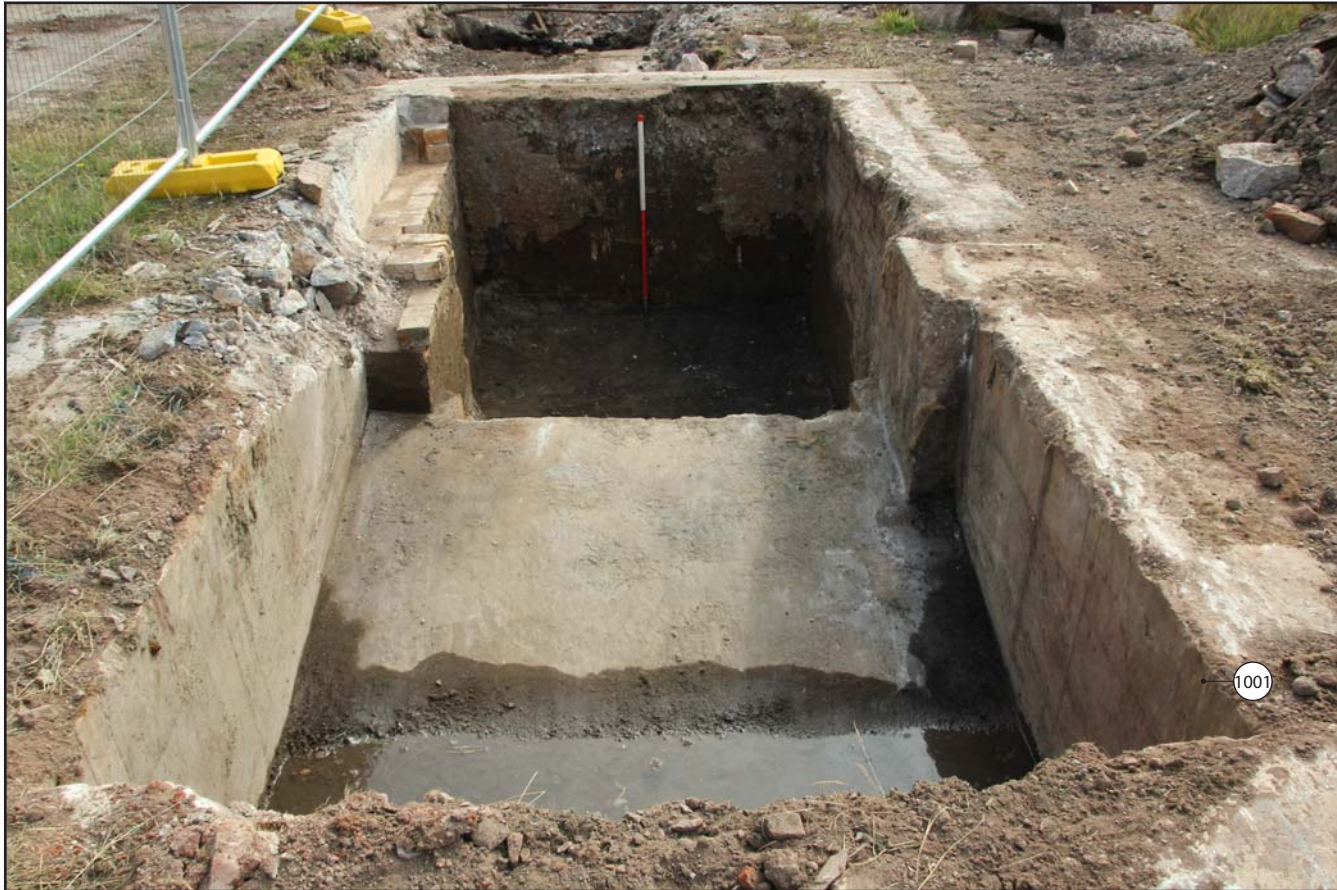
Plate 22: Trench 5 showing concrete and brick tank (1001), from the north. Scale 1.0m.
