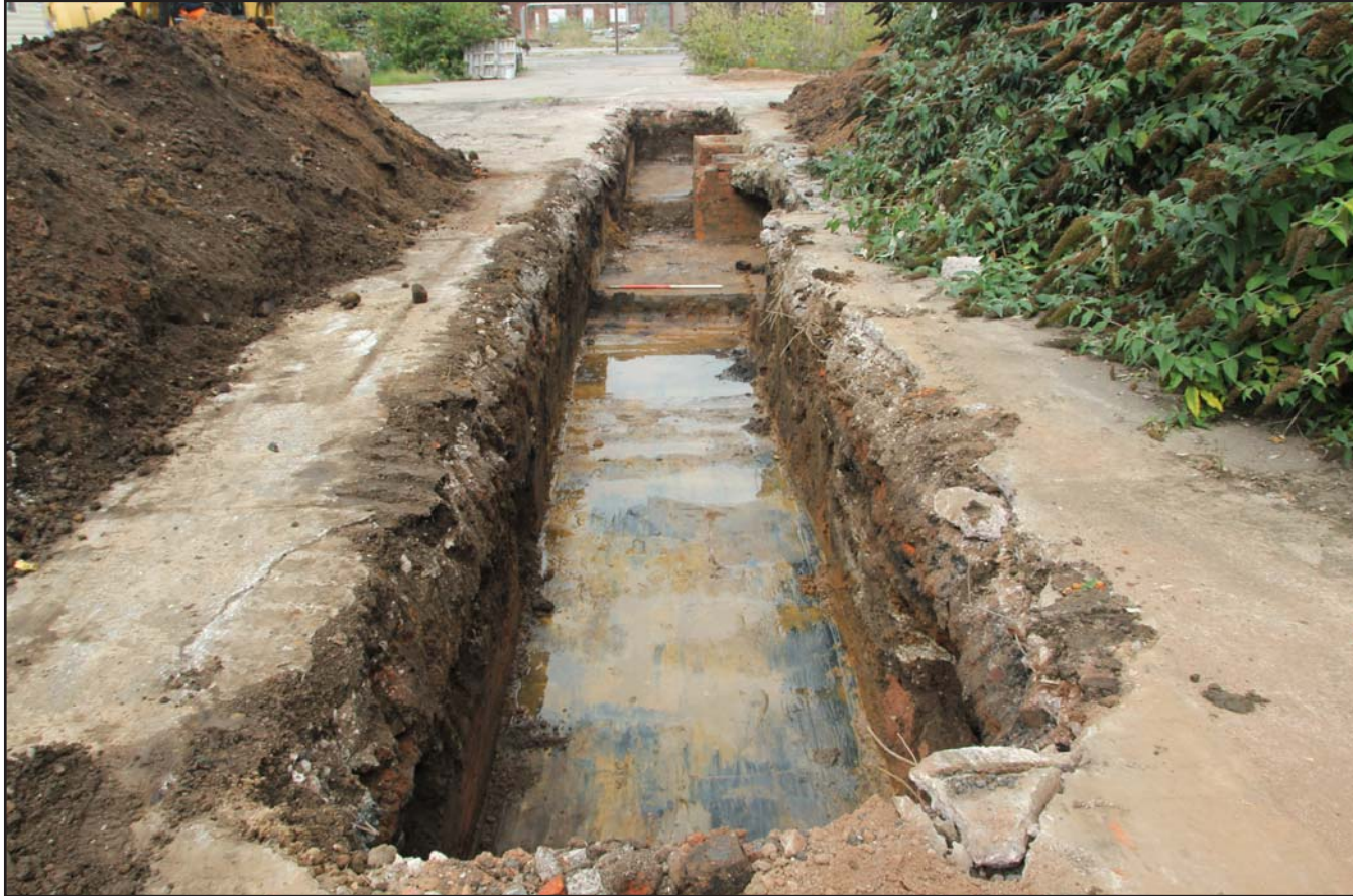
Plate 01: Trench 1, from the south. Scale 1.0m.
