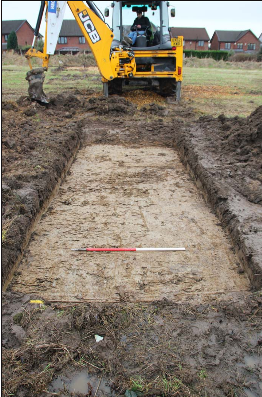
Plate 19: Trench 11, from the north. Scale 1.0m.
