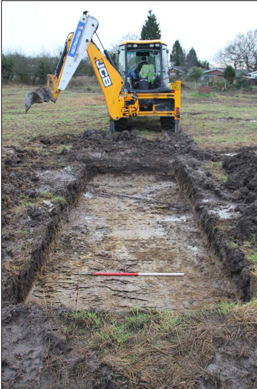
Plate 29: Trench 21, from the north. Scale 1.0m.
