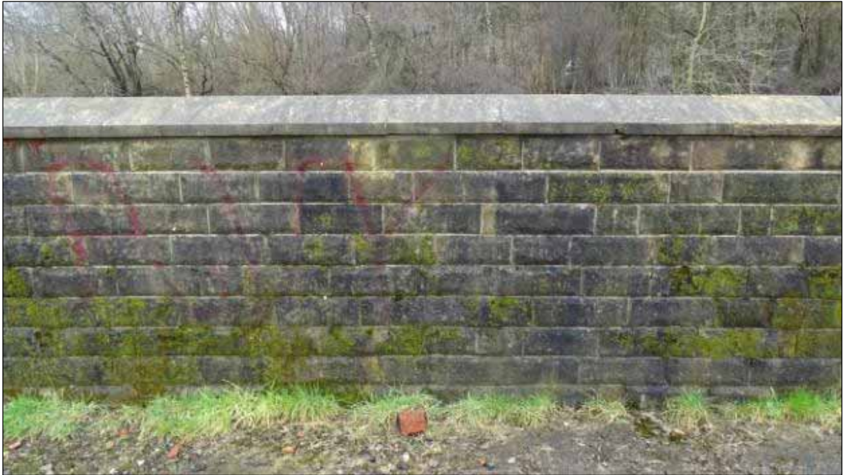
Plate 11: Upstanding stone-built wall atop the northern embankment of the River Roch
