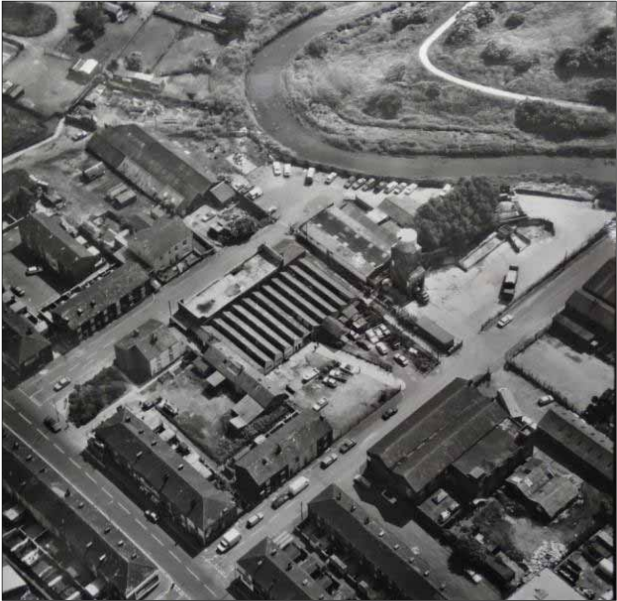
Plate 3: - aerial photograph of the Site, mid 1980s, from the north-east
