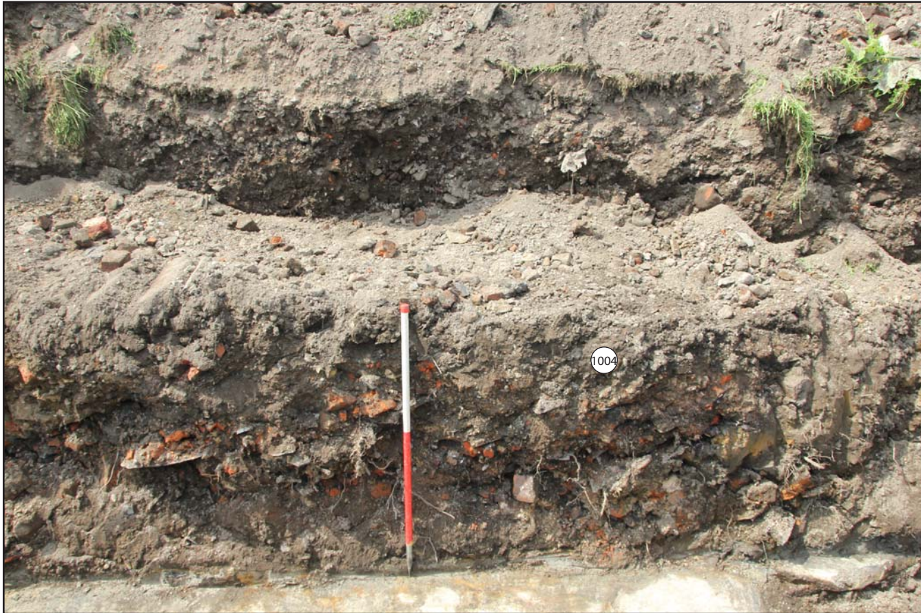
Plate 18: Trench 4 southeast facing section showing demolition deposit (1004), from the southeast. Scale 1.0m.
