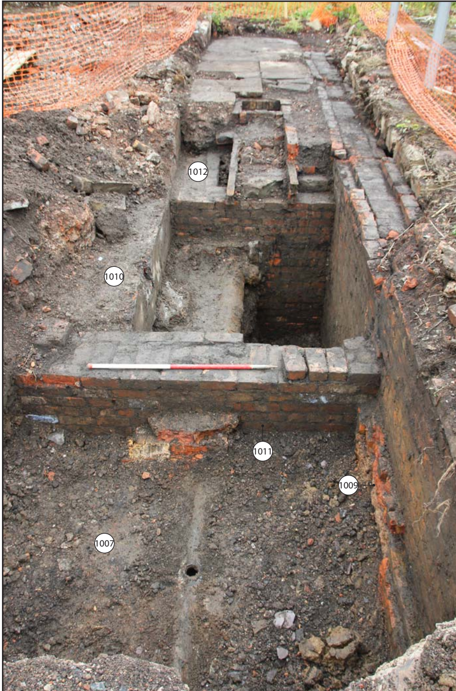
Plate 02: Trench 1 showing remains of the Salford Dyeing and Finishing Works, from the east. Scale 1.0m.
