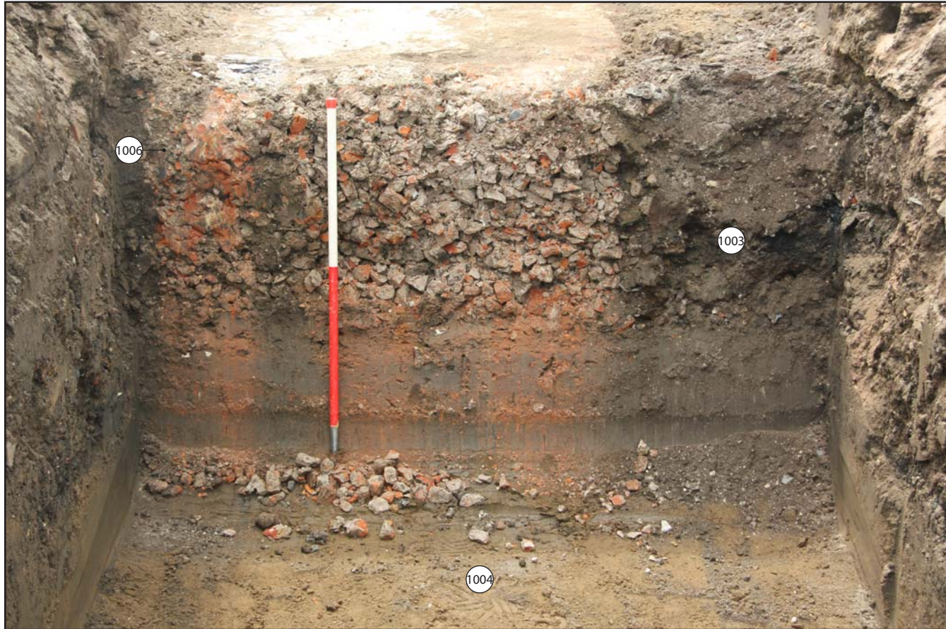
Plate 11: Trench 2 showing concrete anchor block (1006) of Dyeing and Finishing Works, from the north. Scale 1.0m.
