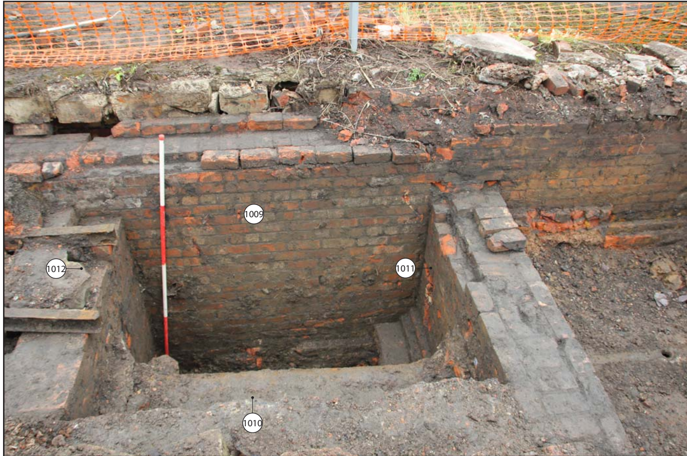
Plate 04: Trench 1 showing inspection chamber, from the south. Scale 2.0m.
