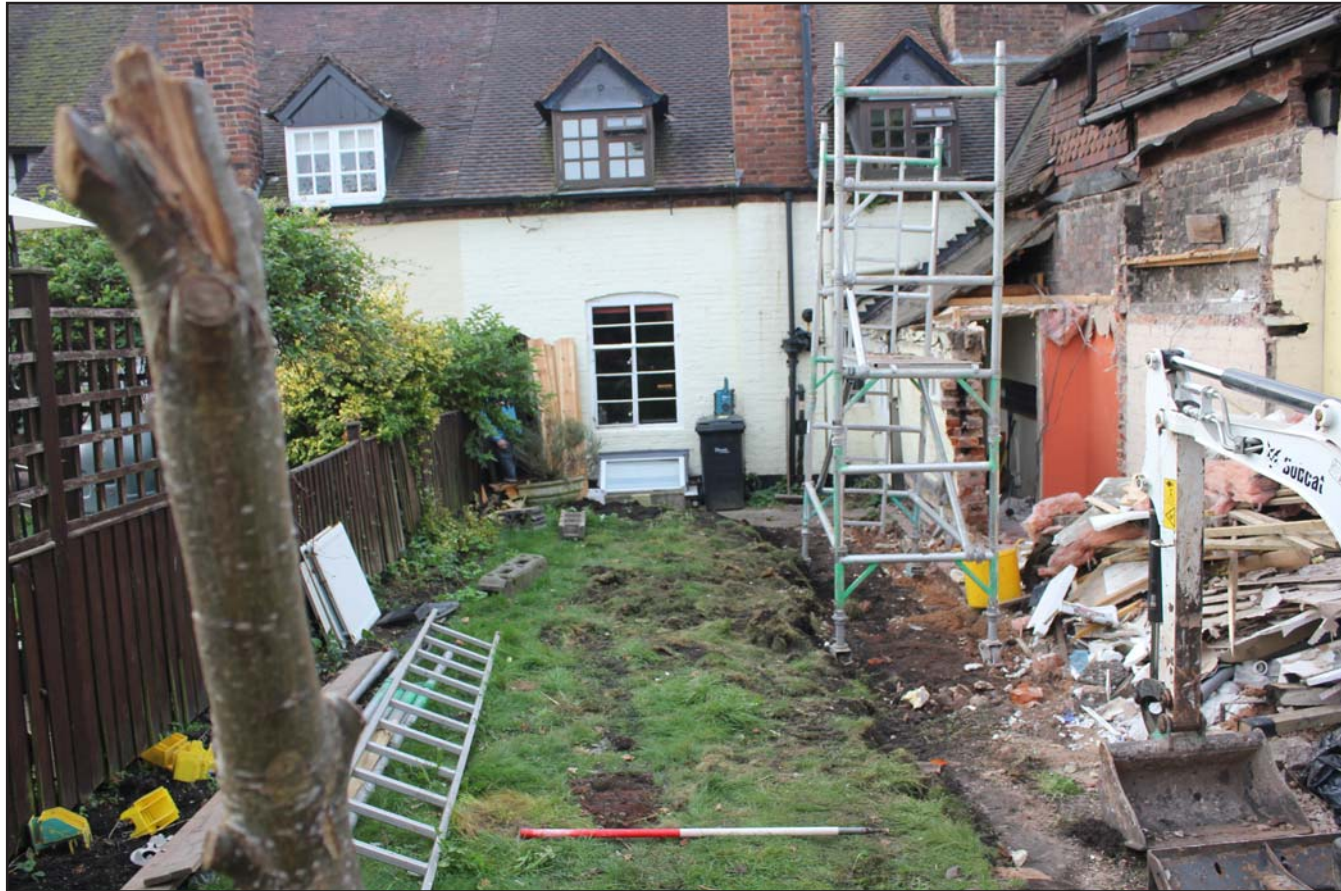
Plate 02: Pre excavation shot - from the north - scale 1m
