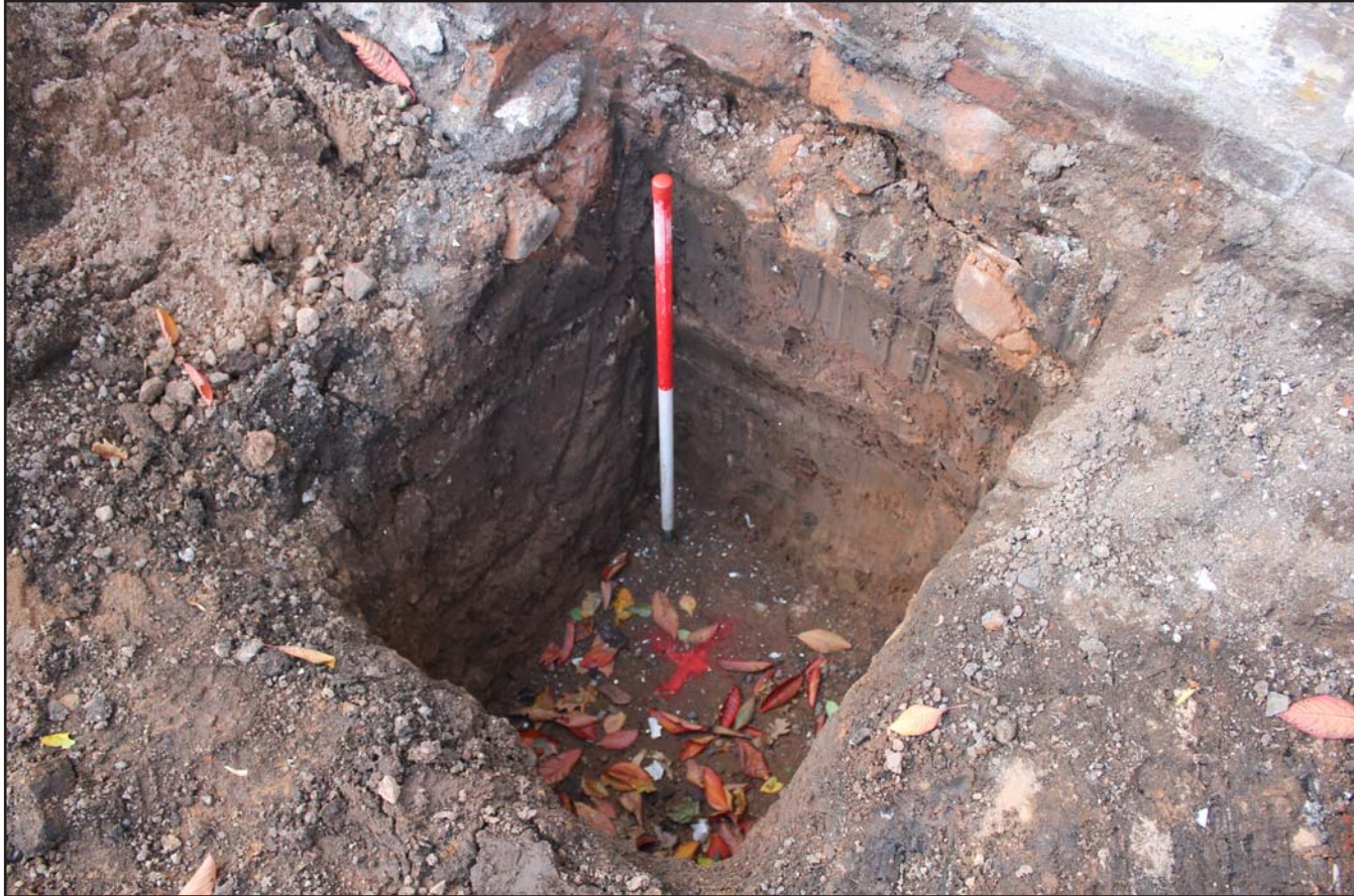
Plate 18: Box excavation for concrete pad - from the northeast - scale 1m
