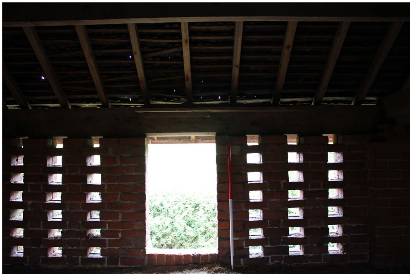
Plate 12: Eastern elevation of hayloft showing ventilation slots, access hatch and roof batons - From West - Scale 1m
