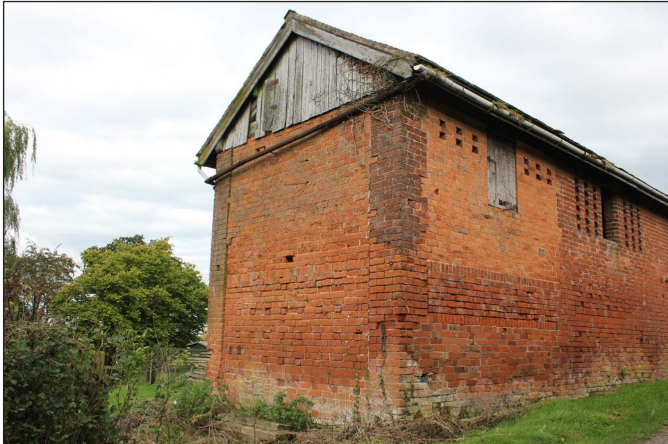
Plate 04: Southern gable showing piers and weather boards - from Southeast - Scale 1m
