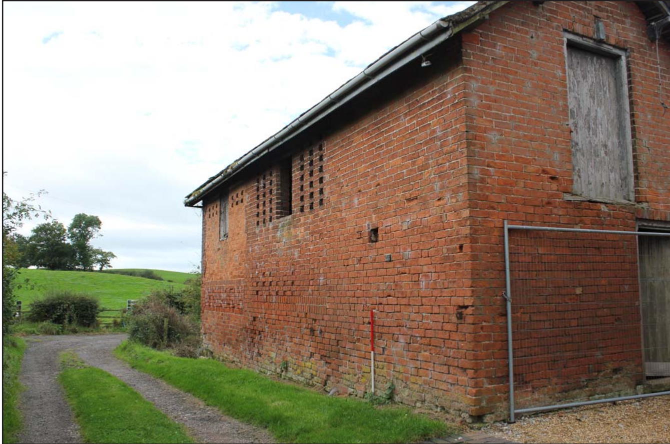
Plate 03: Eastern elevation showing hatches and ventilation slots - from Northeast - Scale 1m
