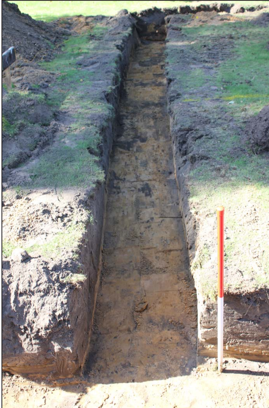
Plate 15: Trench Shot - trench "stepped in" from southern end of footings - from East - Scale 1m
