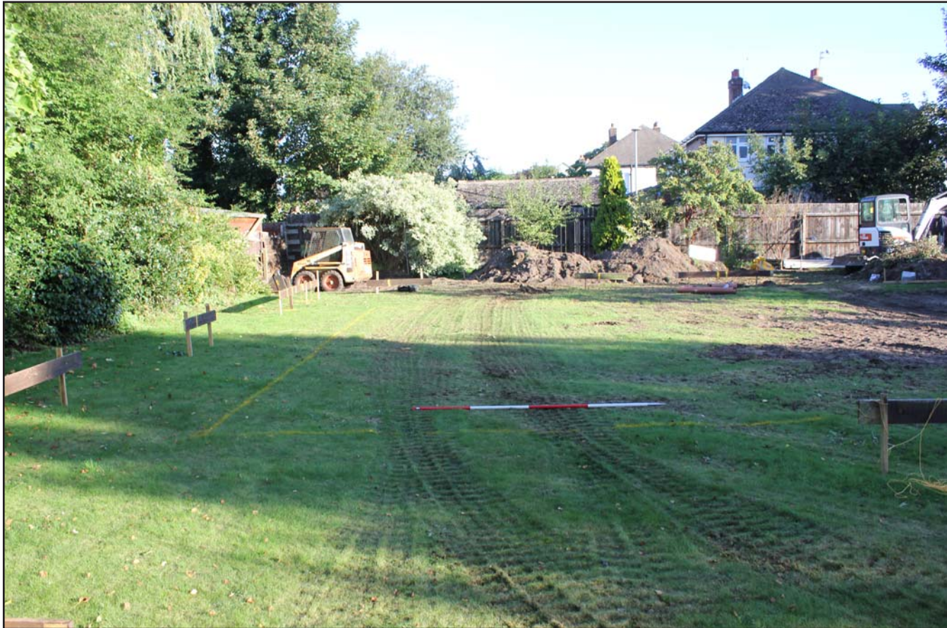
Plate 01: Site Shot - Pre excavation from the South - scale 2m
