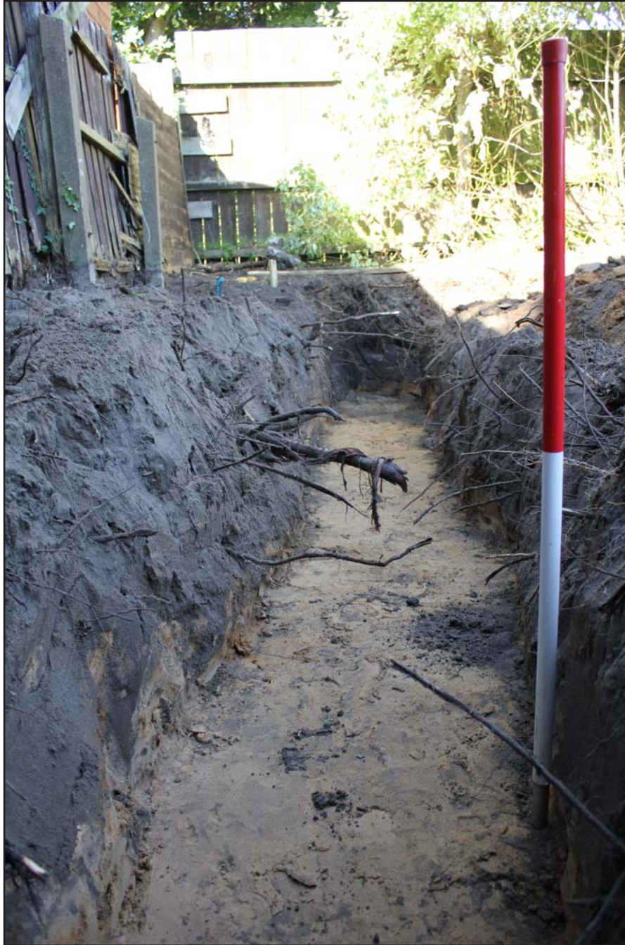
Plate 19: Trench shot - Back of garage - from South - Scale 1m
