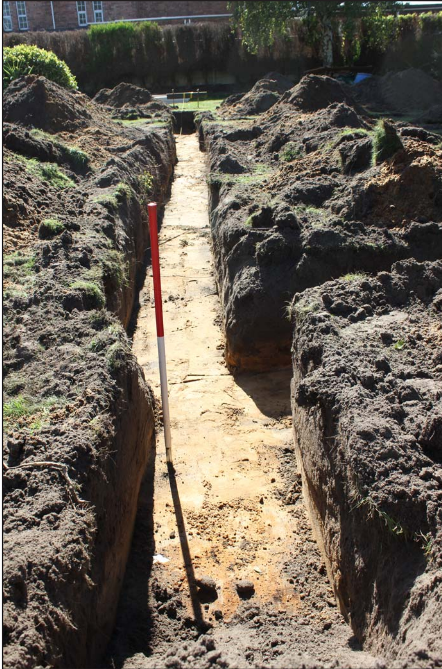
Plate 06: Trench Shot - to north of footings; east of central trench - from North - Scale 1m
