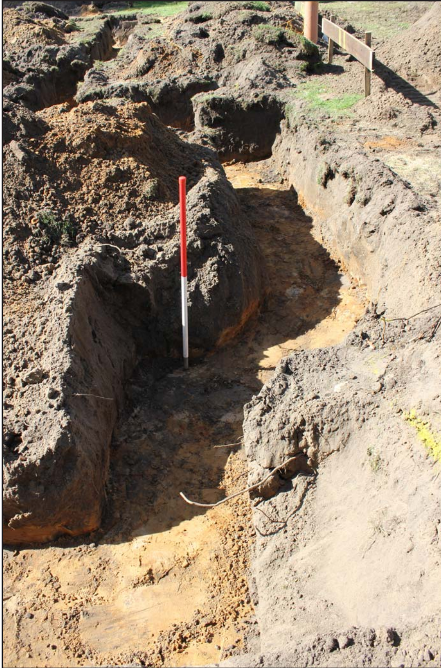
Plate 16: Trench Shot - east of bay window - from East - Scale 1m
