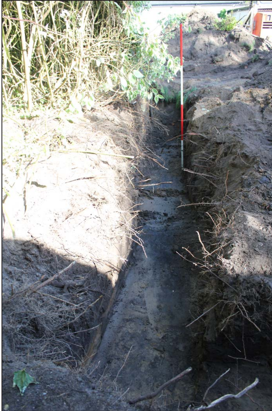
Plate 18: Trench shot - Northern arm of garage - from West - Scale 2m
