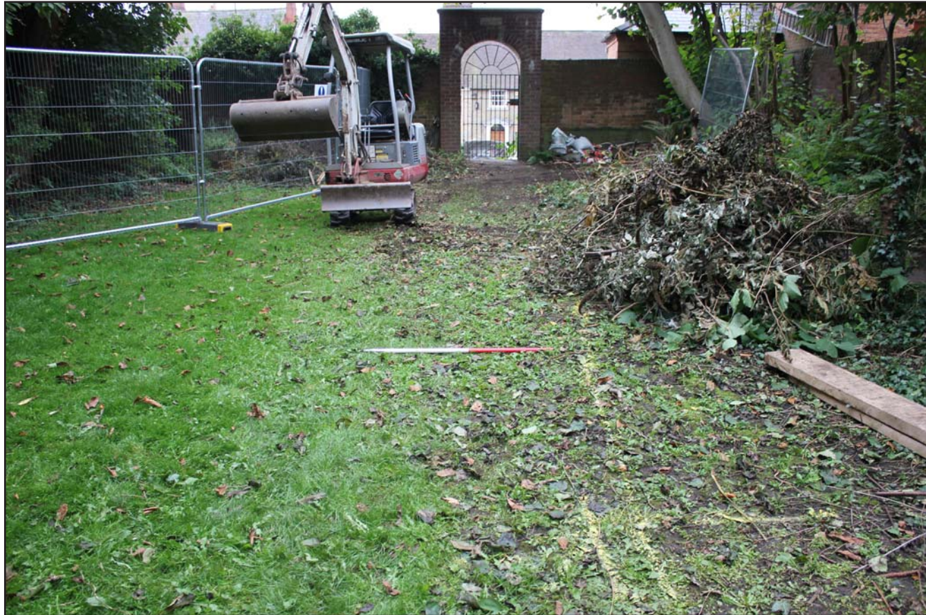
Plate 01: Pre excavation of trench 2 from north- scale 1m
