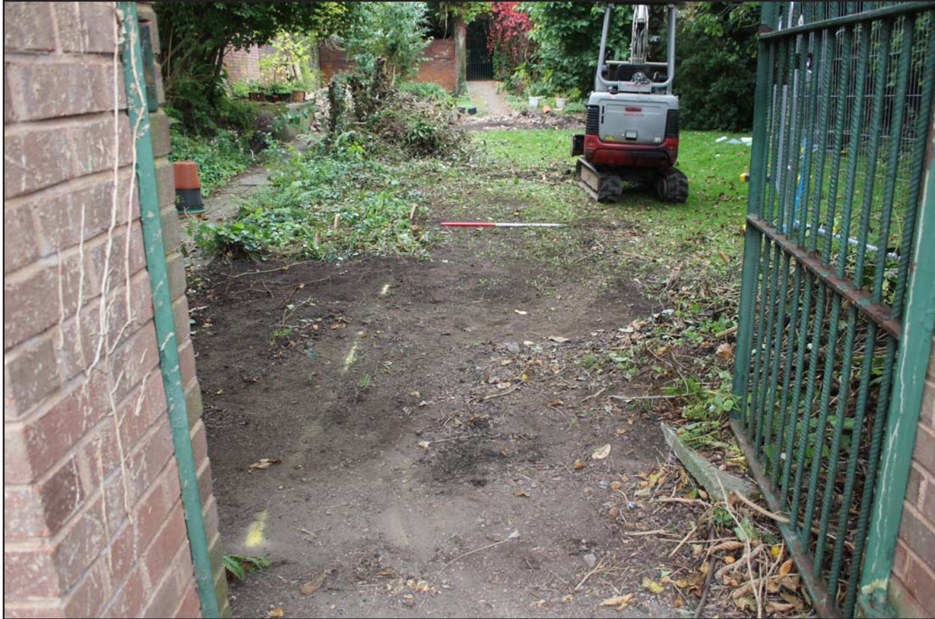
Plate 02: Pre excavation of trench 2 from south - scale 1m
