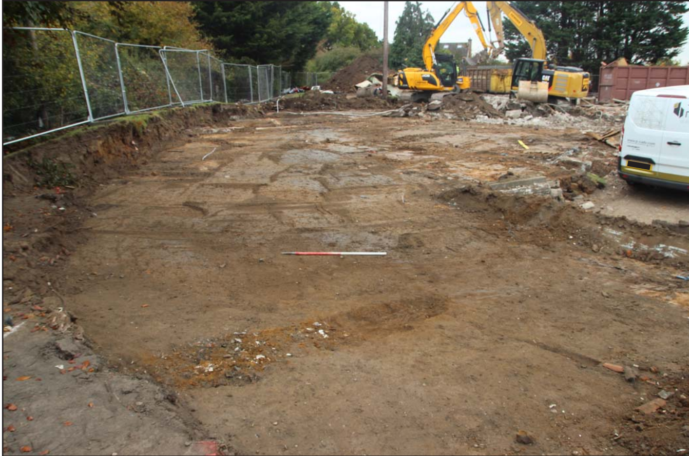
Plate 08: Post excavation shot of northern portion of site following reduced excavation - from north - scale 1m
