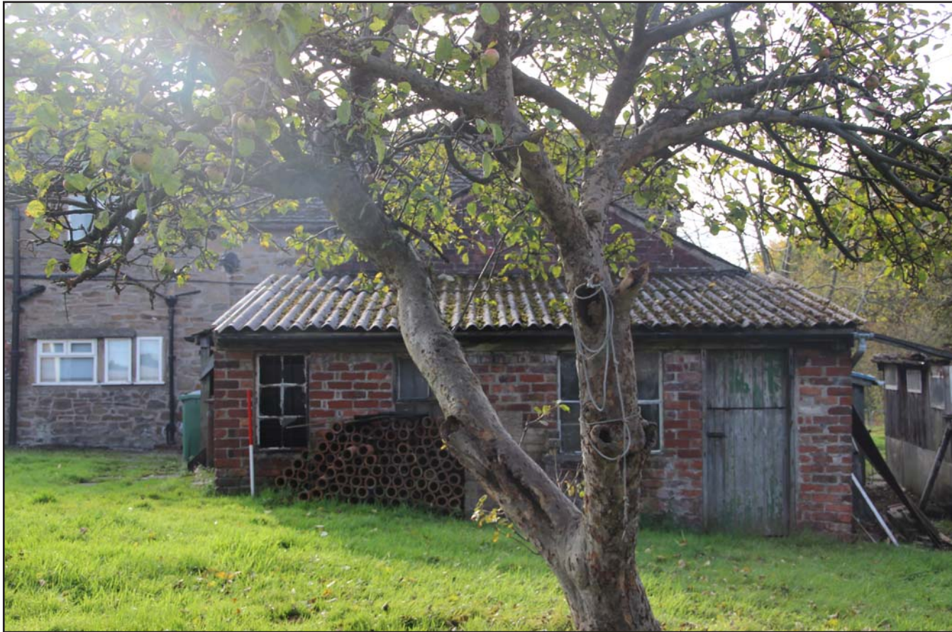
Plate 08: North facing outbuilding external elevation, from the north. Scale 1.0m.
