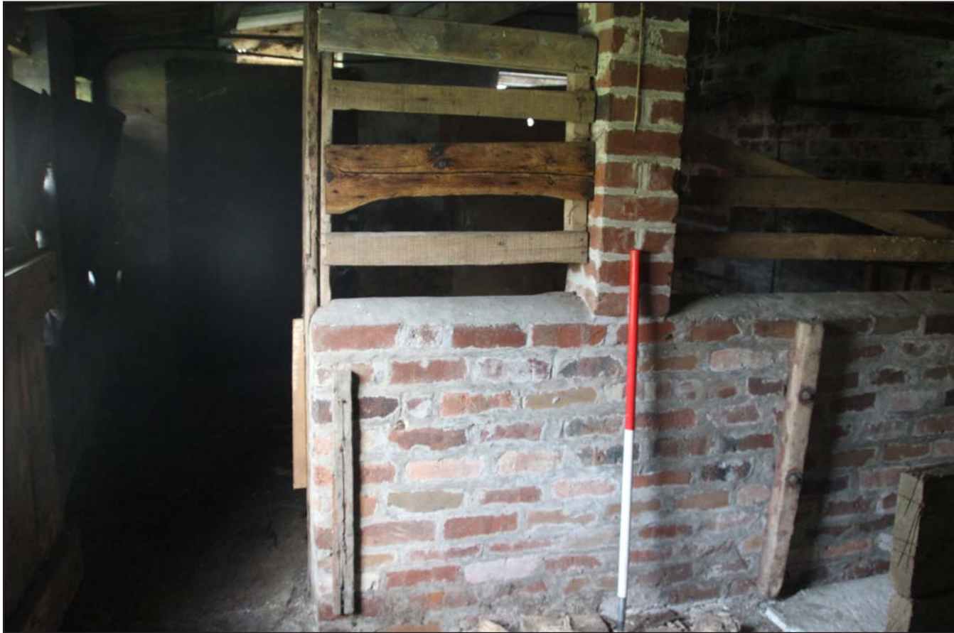
Plate 36: Outbuilding store/kennel, from the northwest. Scale 1.0m.
