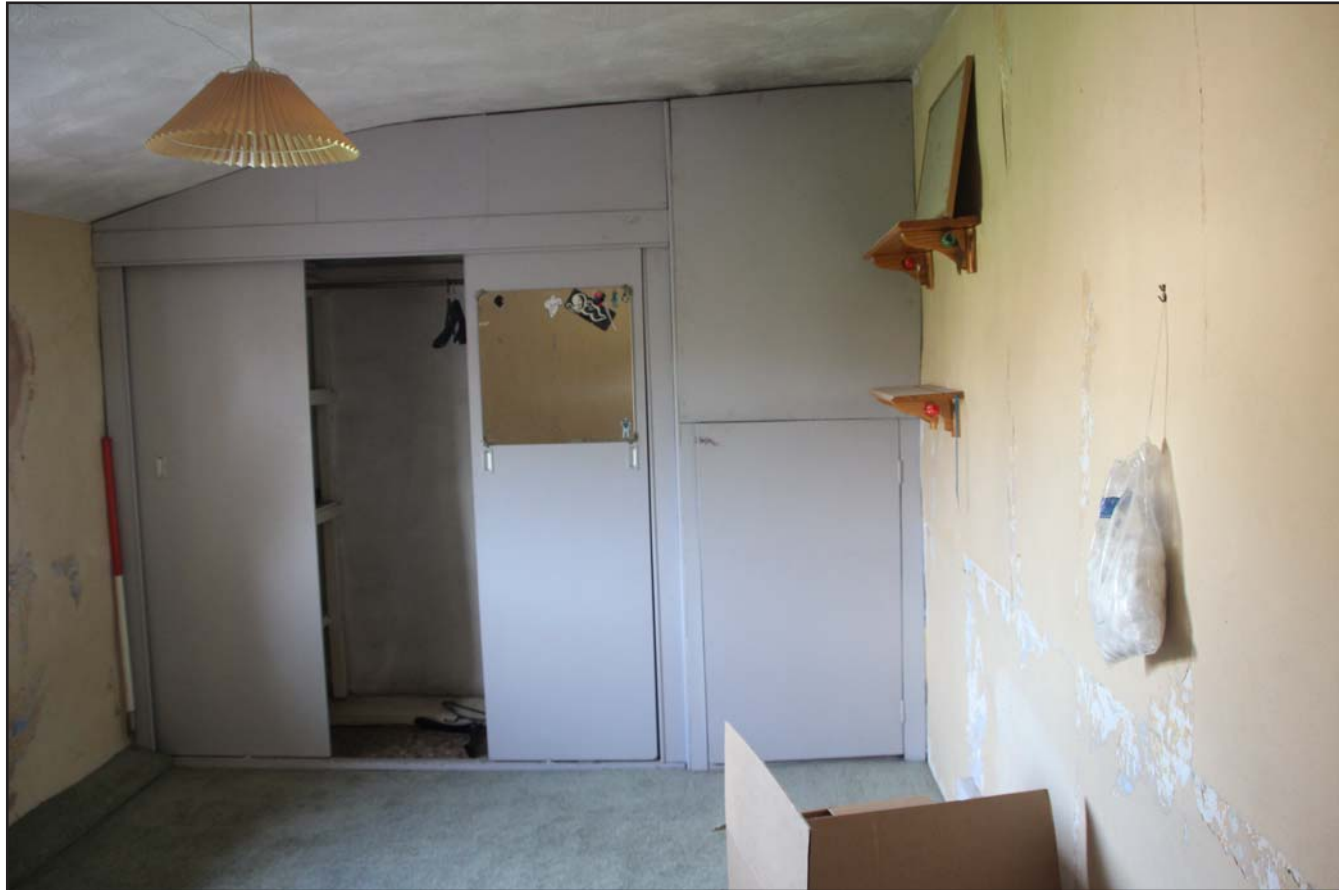
Plate 27: Bedroom 1, from the west. Scale 1.0m.
