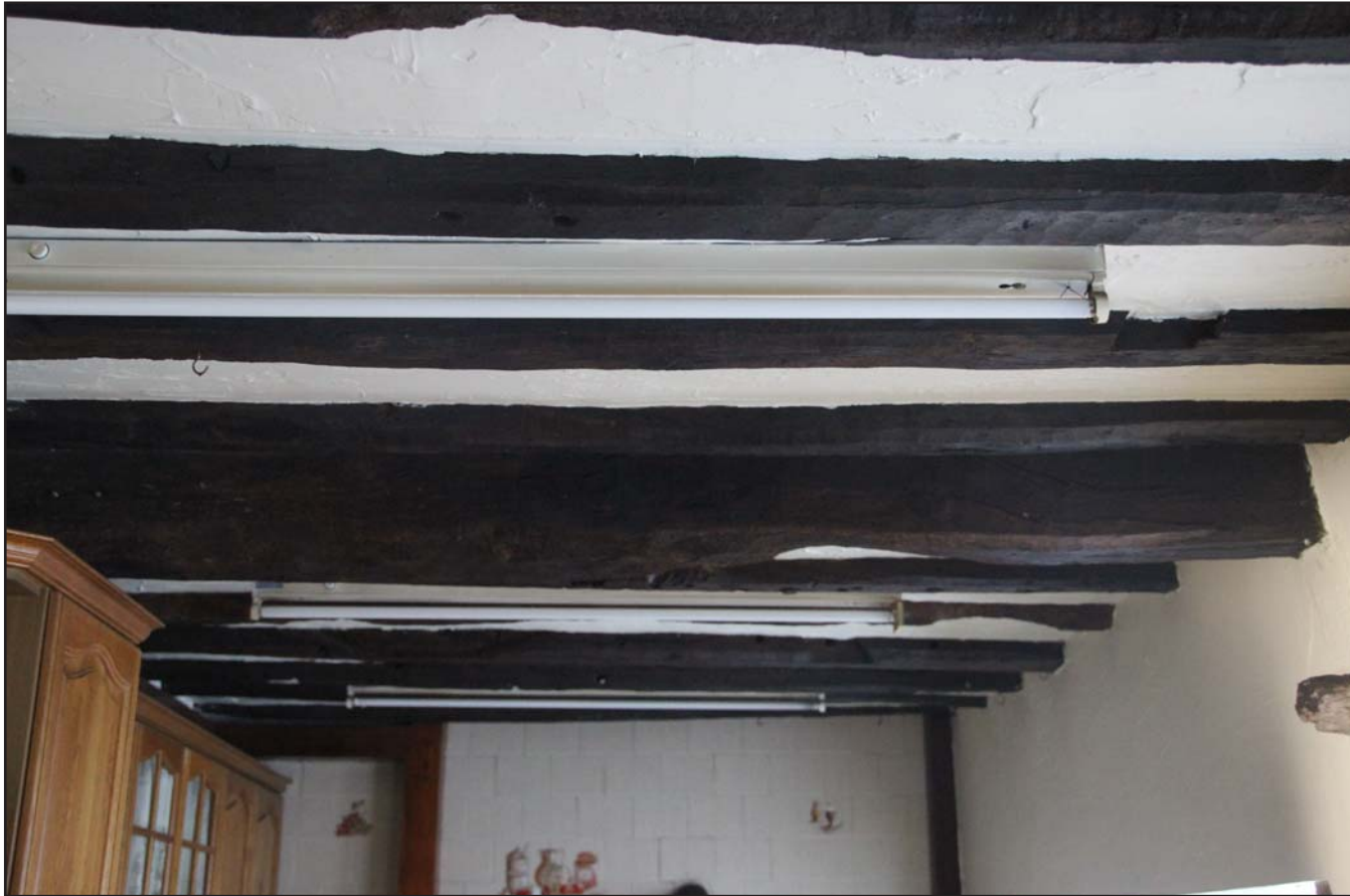
Plate 15: Kitchen/diner roof beam, from the east.
