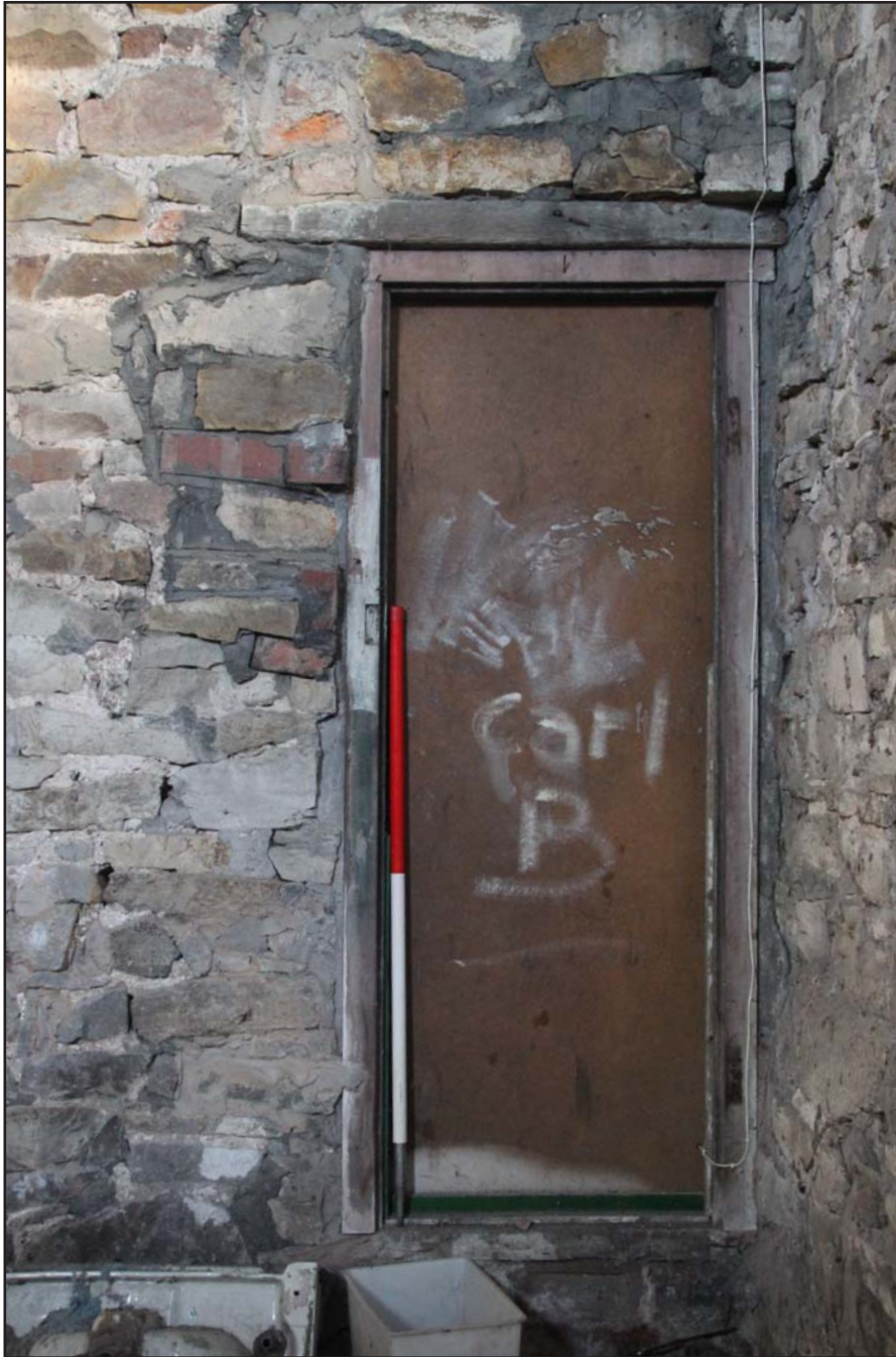
Plate 33: Byre 1 blocked doorway, from the west. Scale 1.0m.
