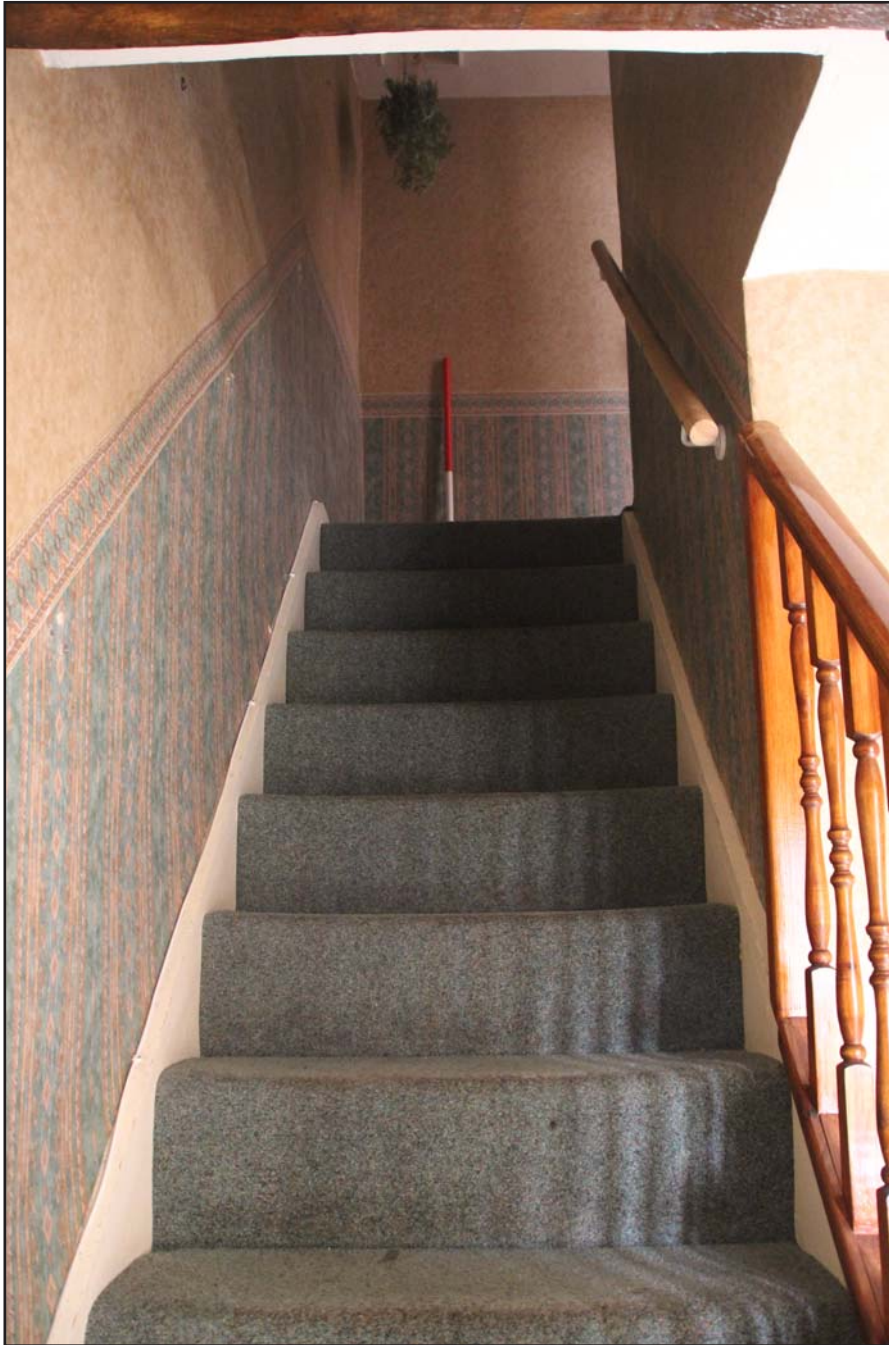
Plate 24: Stairwell, from the south. Scale 1.0m.
