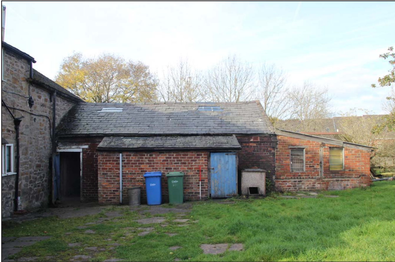
Plate 06: East facing outbuilding external elevation, from the east. Scale 1.0m.
