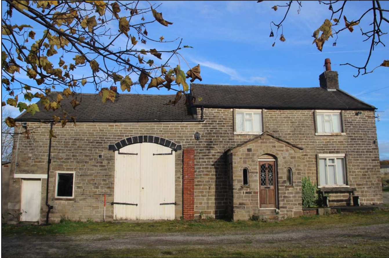
Plate 01: South facing external elevation, from the south. Scale 1.0m.
