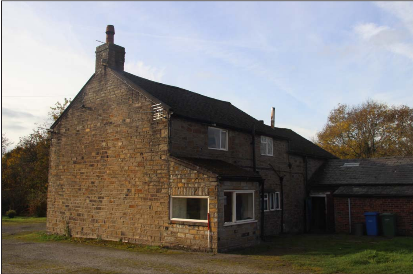
Plate 04: East and north facing external elevations, from the northeast. Scale 1.0m.
