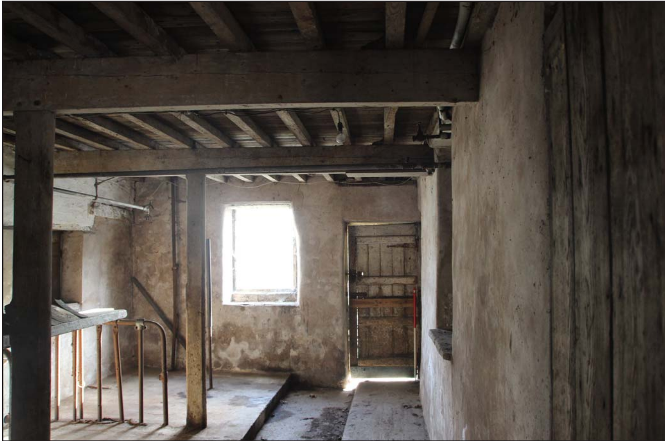
Plate 34: Byre 2, from the north. Scale 1.0m.
