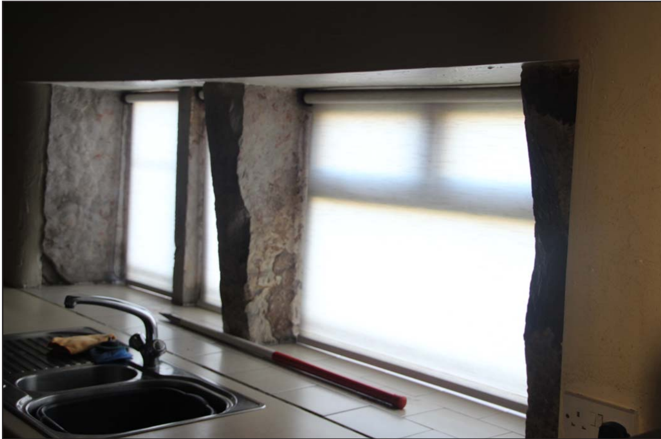
Plate 16: Kitchen/diner windows, from the southeast. Scale 1.0m.
