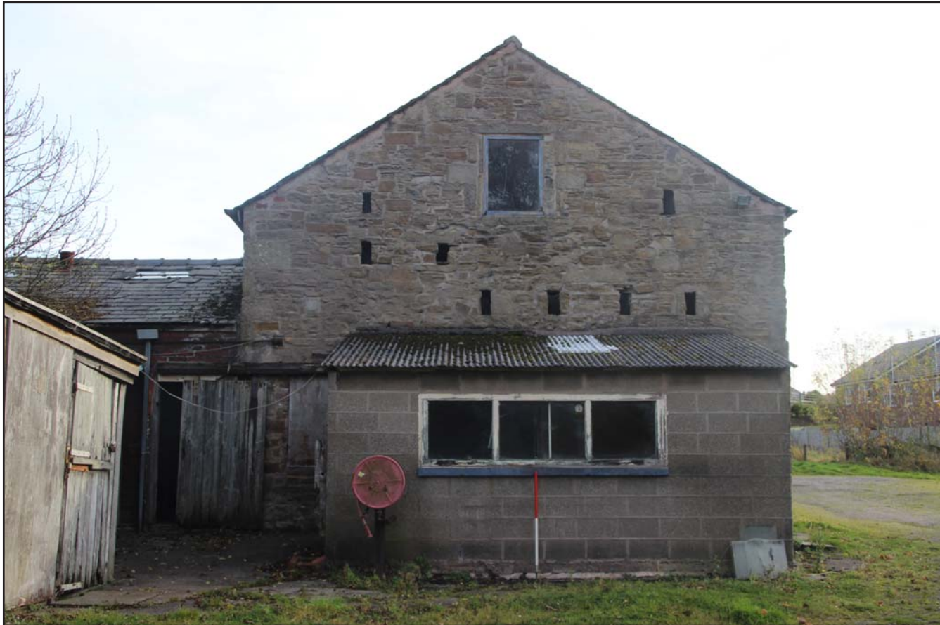
Plate 10: West facing external elevation, from the west. Scale 1.0m.
