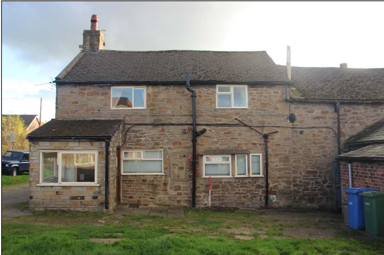
Plate 05: North facing external elevation, from the north. Scale 1.0m.
