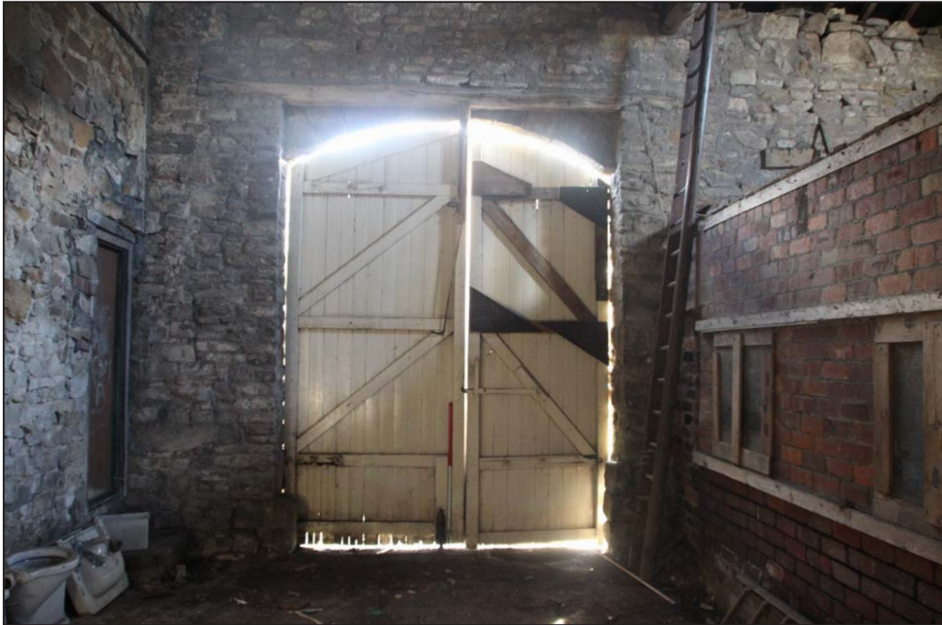
Plate 30: Byre 1, from the north. Scale 1.0m.
