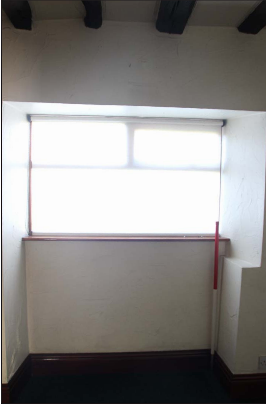
Plate 17: Kitchen/diner blocked door, from the south. Scale 1.0m.
