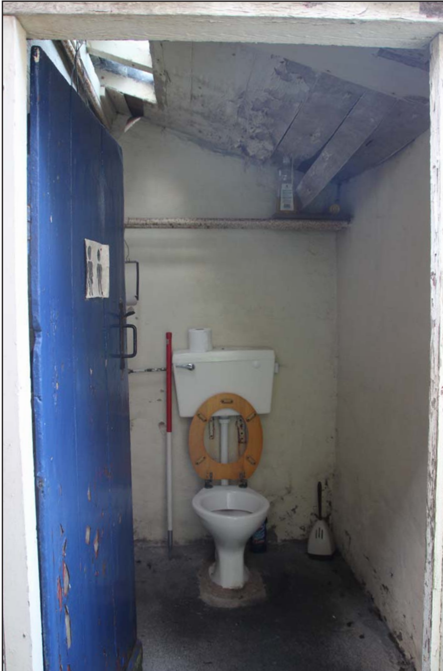
Plate 37: Outbuilding toilet block, from the south. Scale 1.0m.
