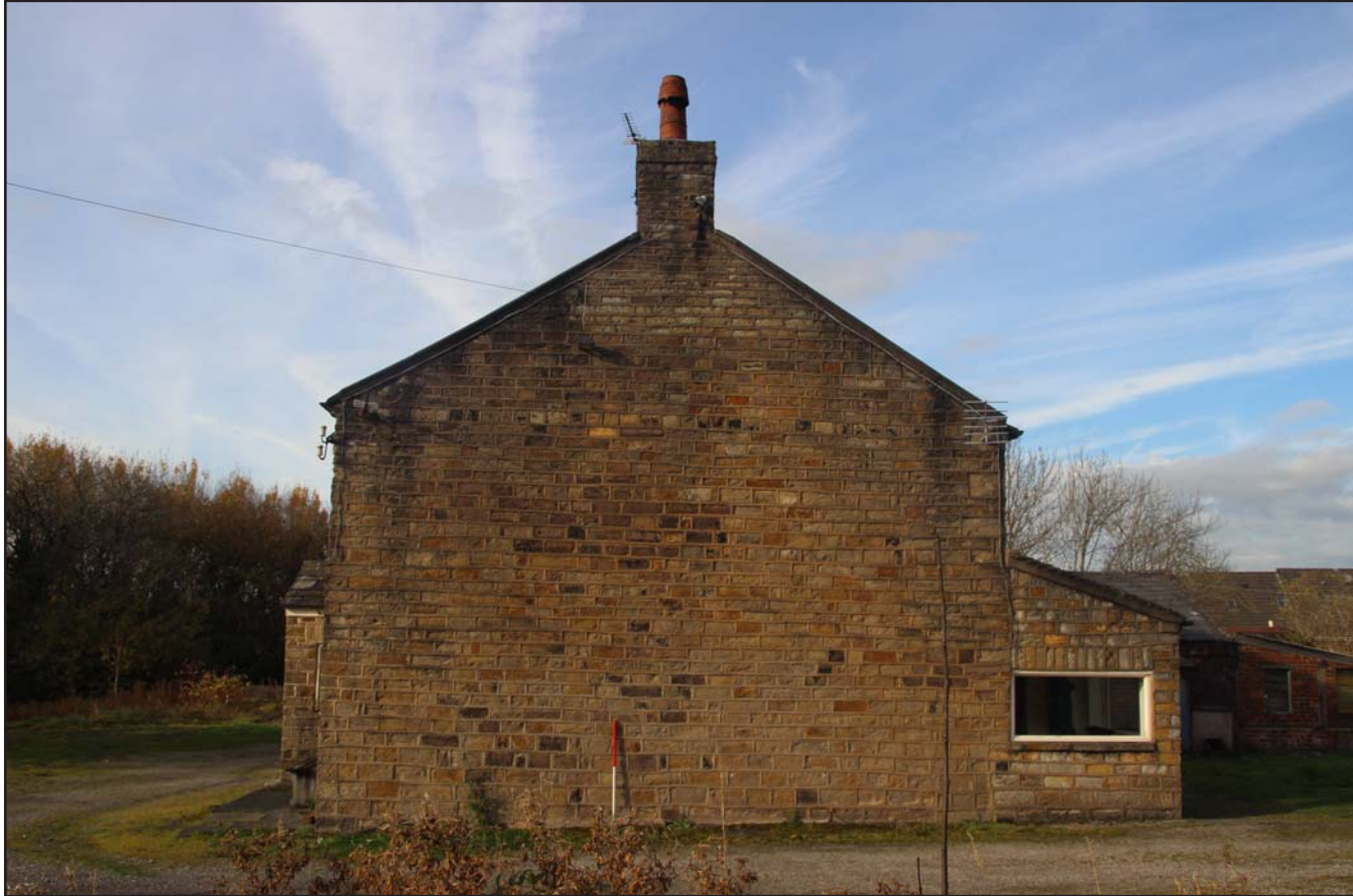
Plate 03: East facing external elevation, from the east. Scale 1.0m.
