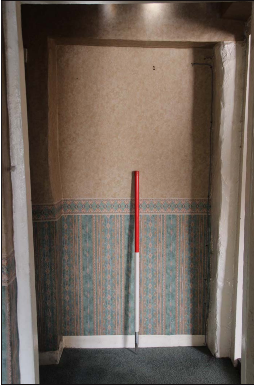
Plate 21: Cloak Room blocked doorway, from the south. Scale 1.0m.
