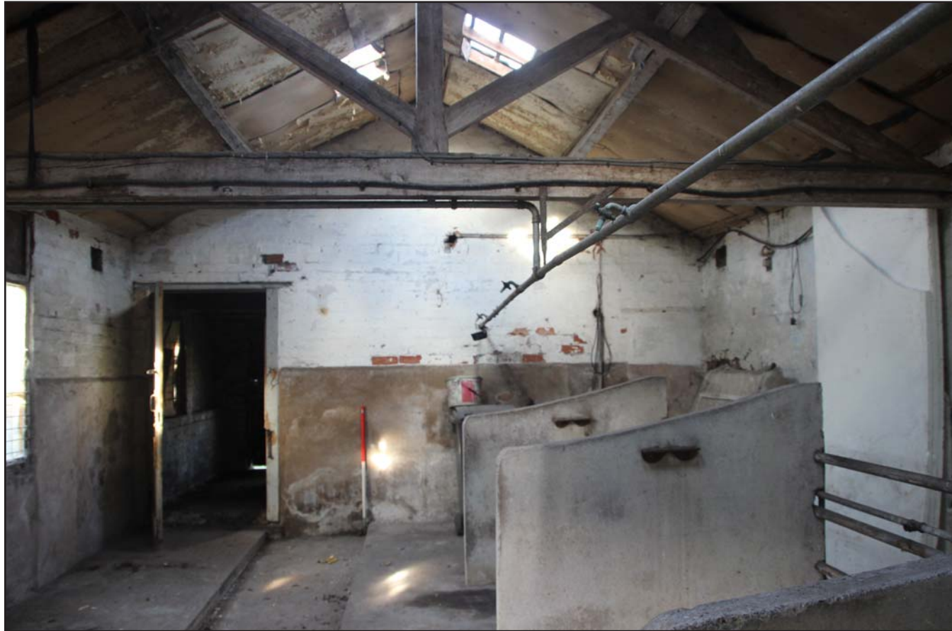
Plate 35: Outbuilding milking parlour, from the north. Scale 1.0m.
