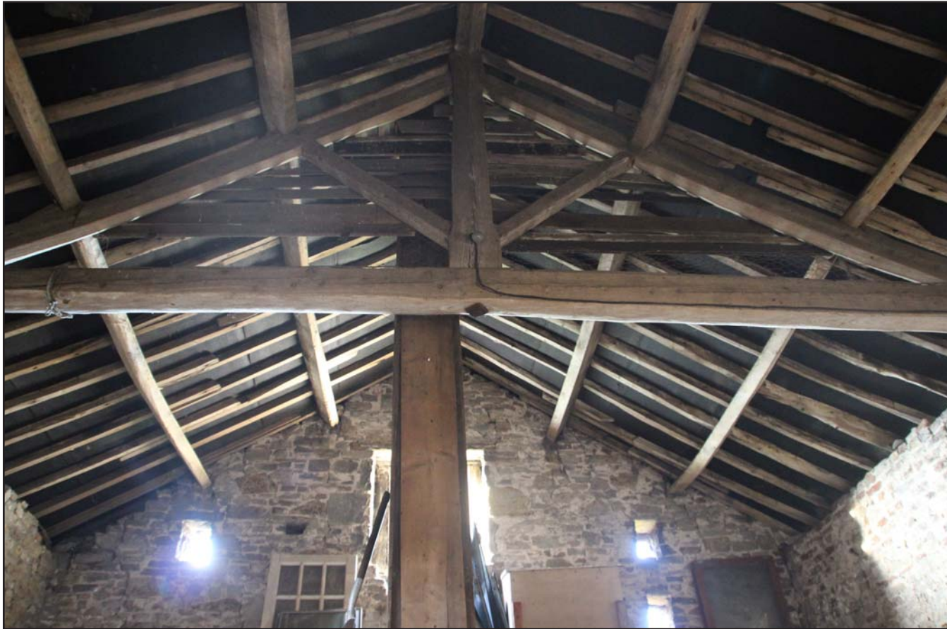
Plate 32: Byre roof showing truss and purlins, from the east.
