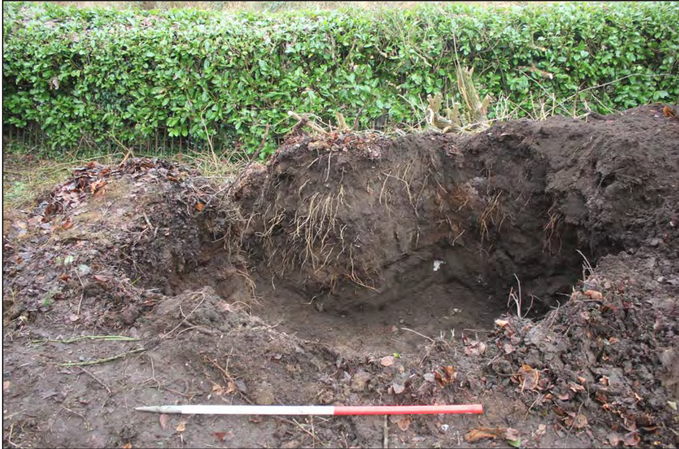
Plate 15: General shot of Drop Shaft Excavation - 1m scale
