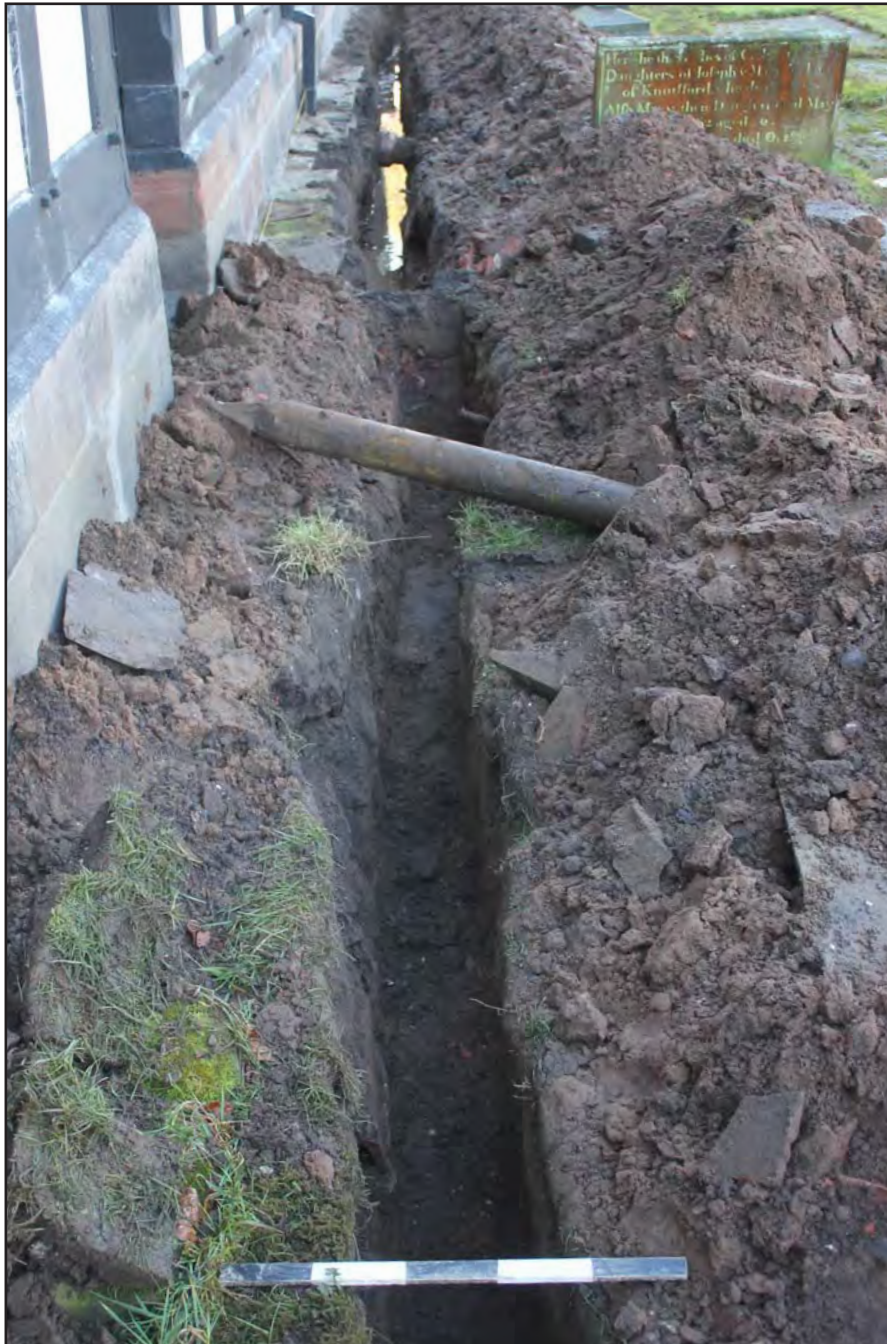
Plate 26: Shot of excavated service trench - from east - 0.5m scale
