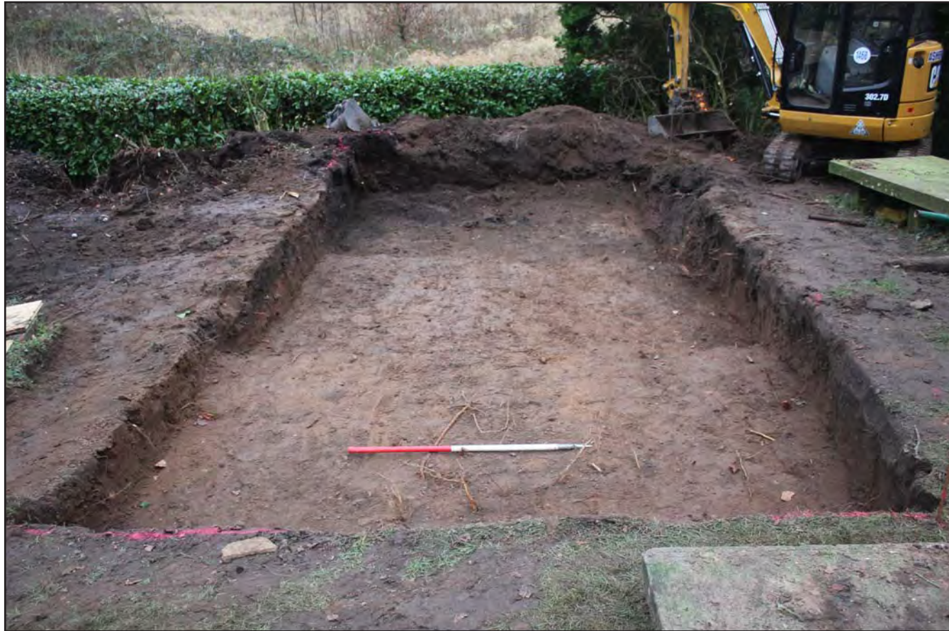
Plate 18: Shot of toilet block trench excavation from west - 1m scale
