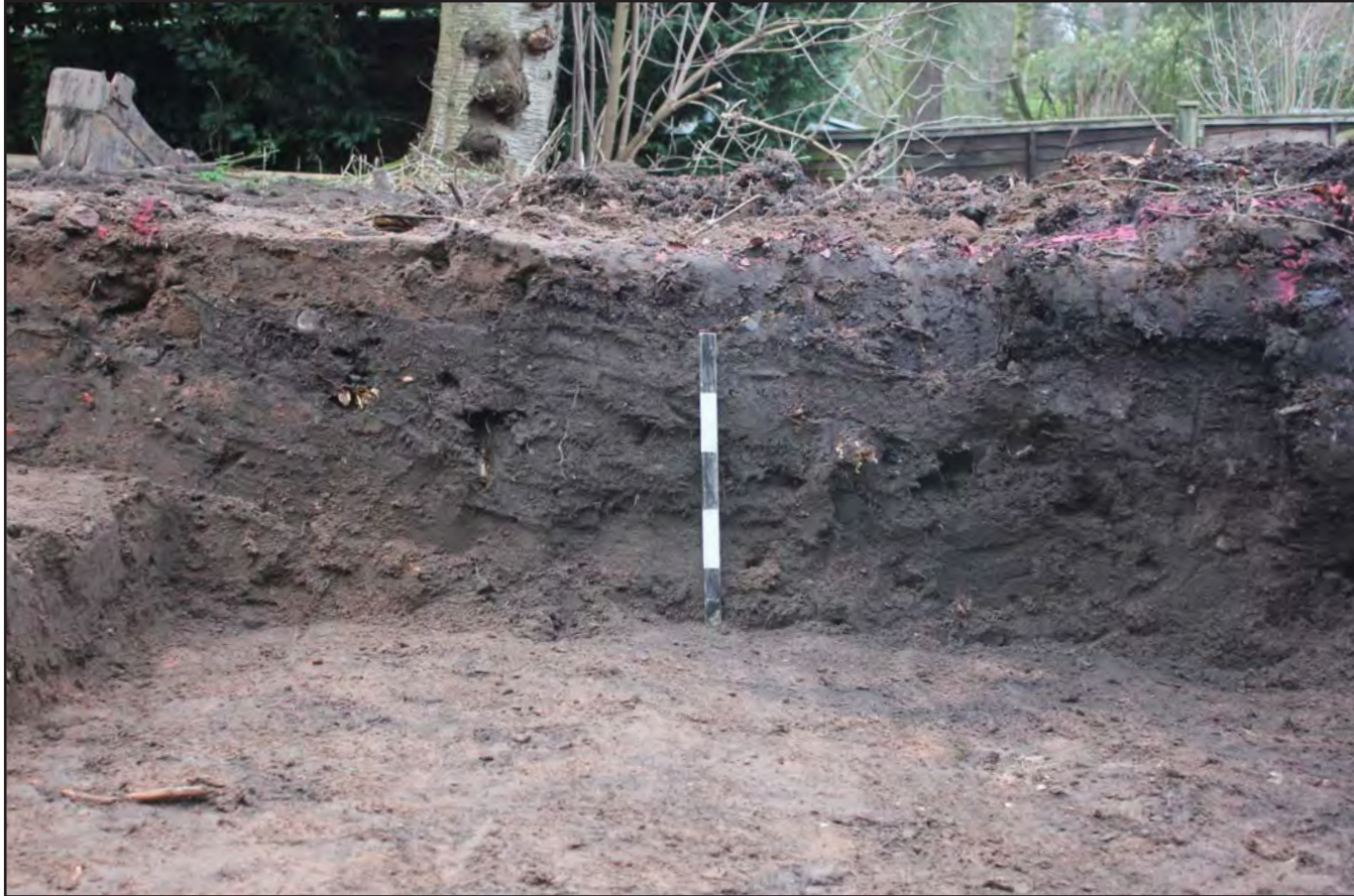
Plate 22: Shot of northern section (right hand end) of toilet block trench excavation from south - 0.5m scale
