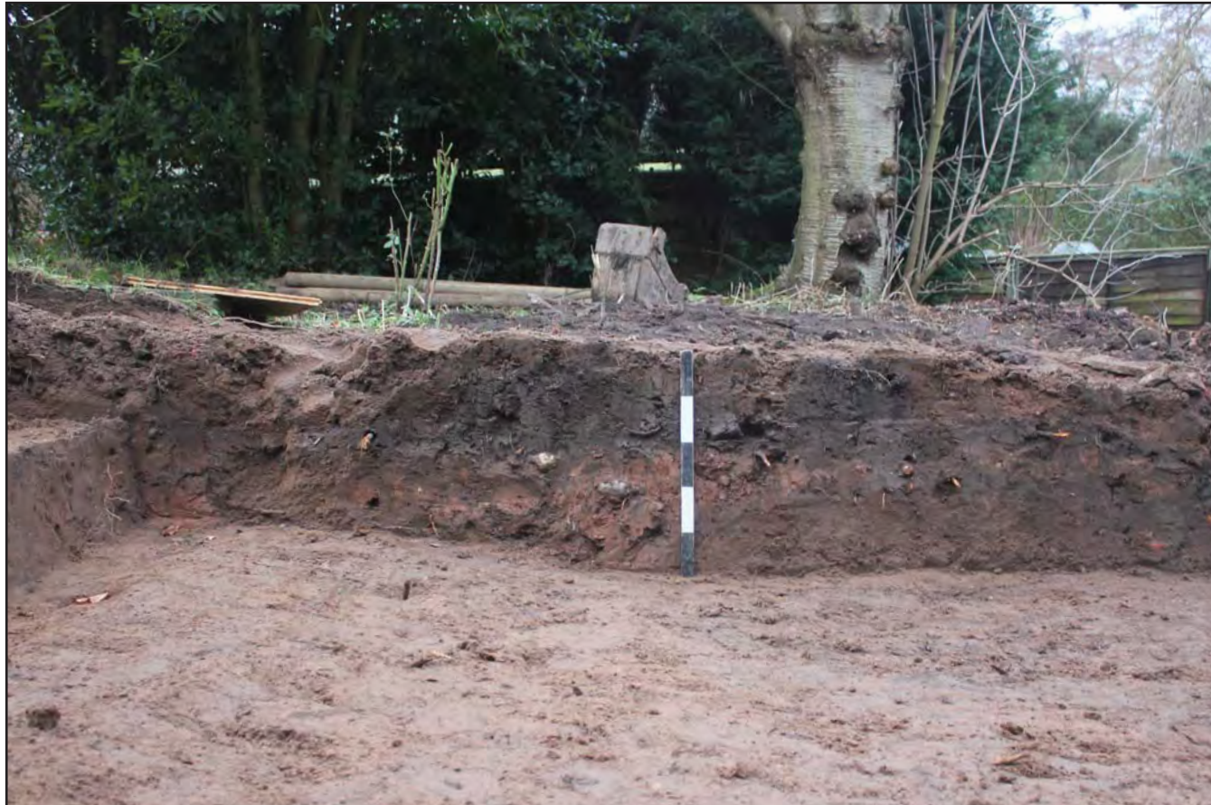
Plate 21: Shot of northern section (centre) of toilet block trench excavation, showing clay (1006) from south - 0.5m scale
