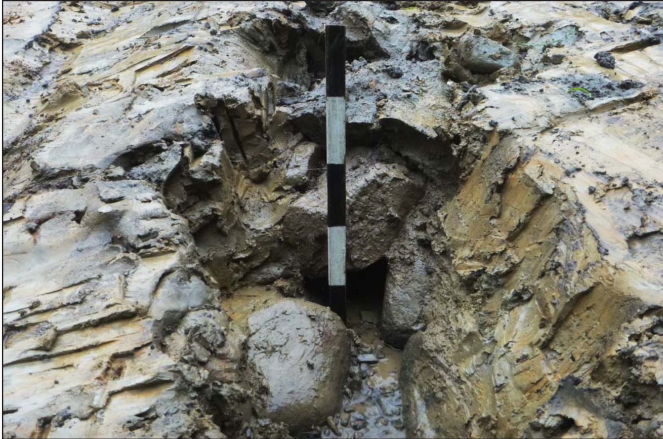
Plate 03: Section of field drain [1006] from Southwest - scale 0.5m
