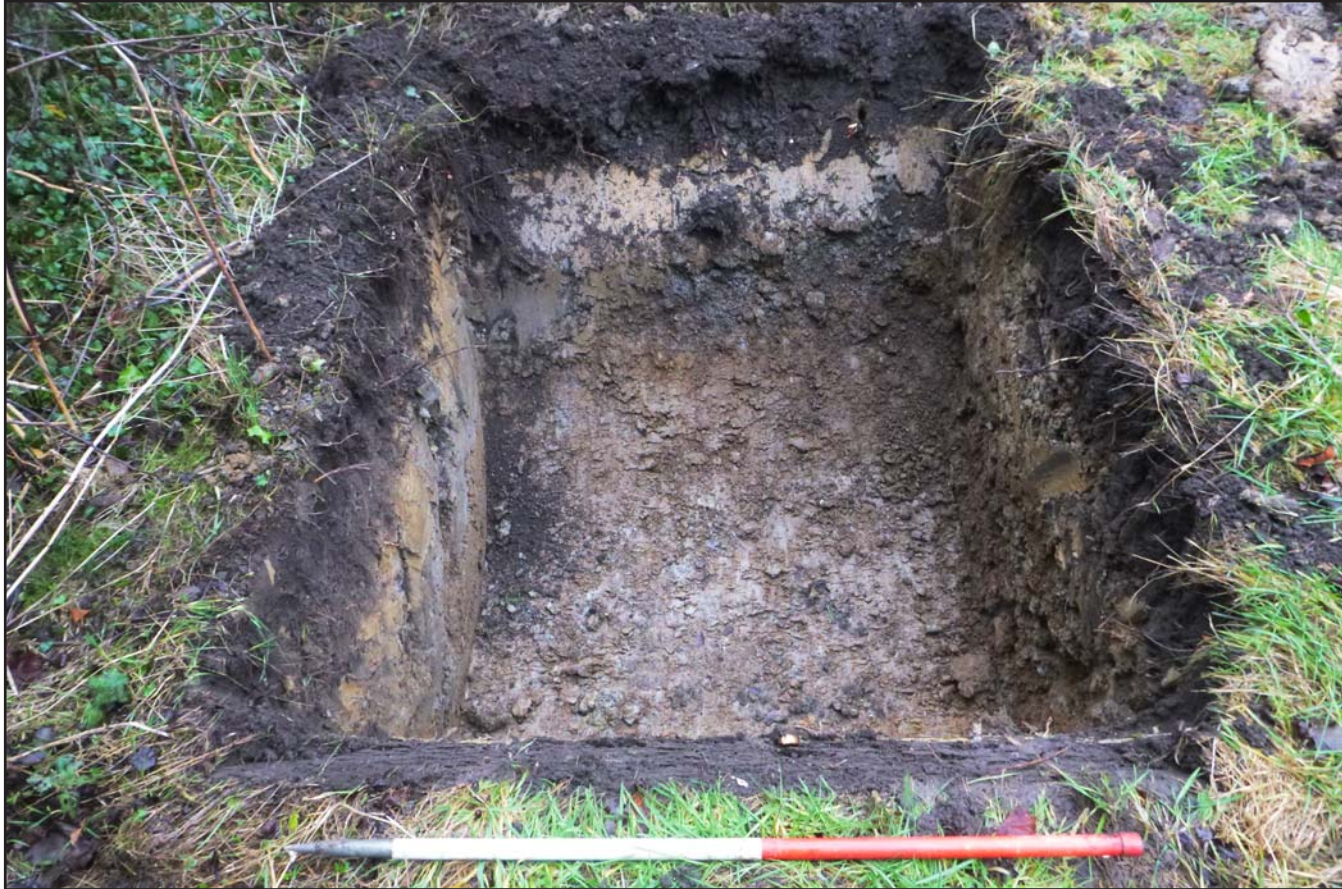
Plate 12: Plan Shot of soakaway trench - scale 1m
