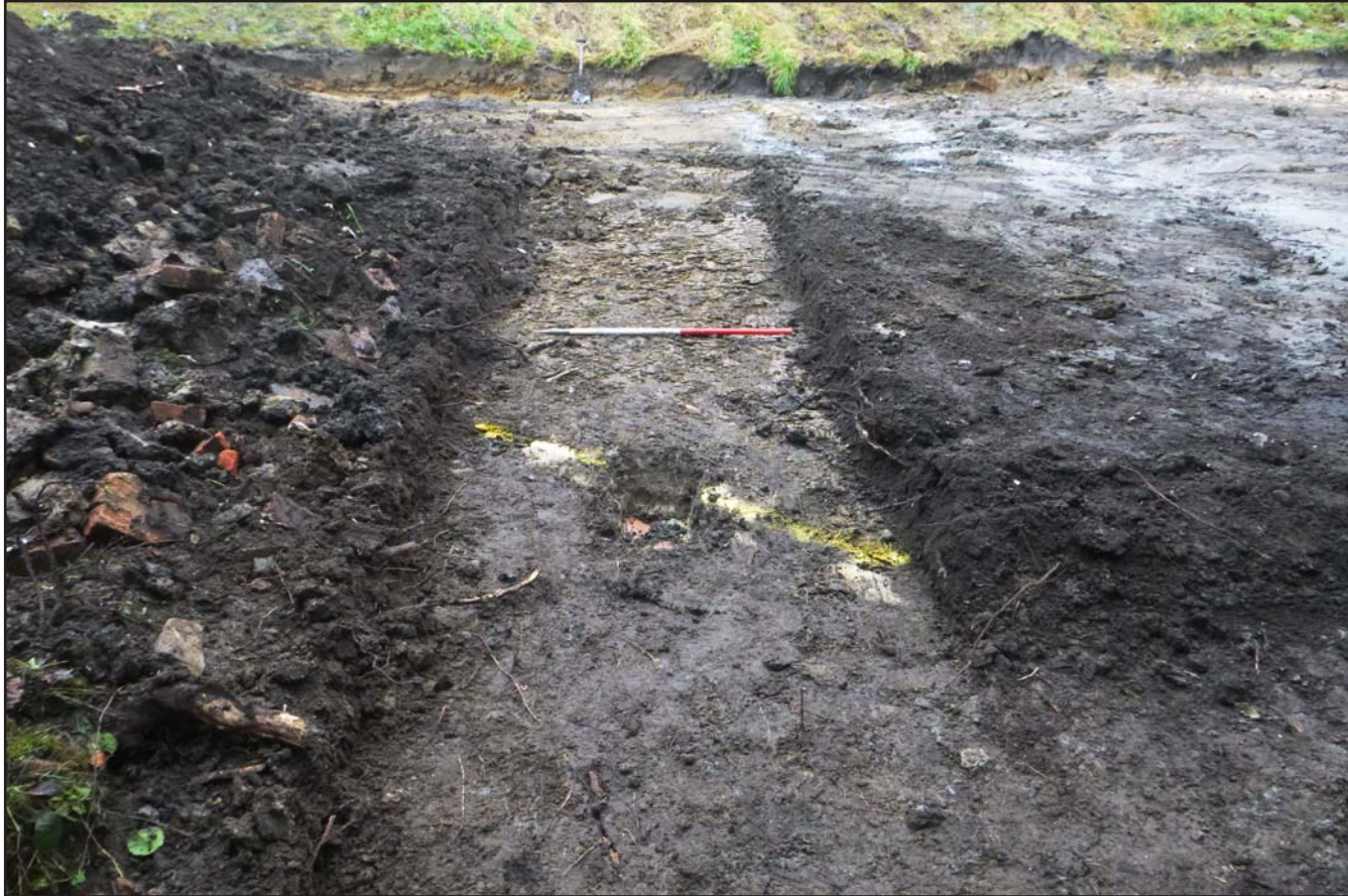
Plate 09: Northern foundation trench showing natural glacial substrata from Northwest - scale 1m
