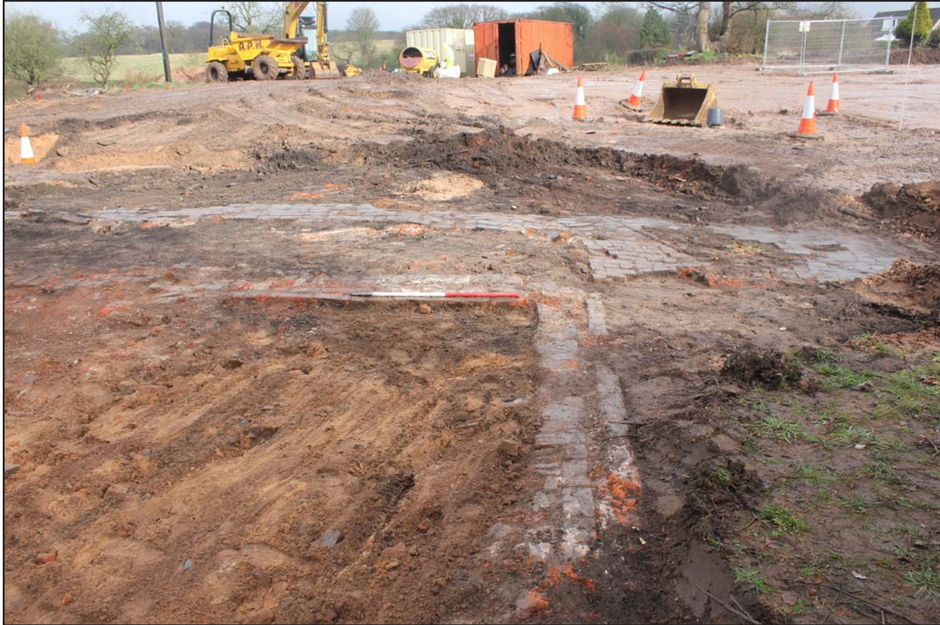
Plate 06: Plan shot of brick foundation wall (1004) foreground and pathway (1005) & floor surface (1007) to rear - from the southwest - scale 1m
