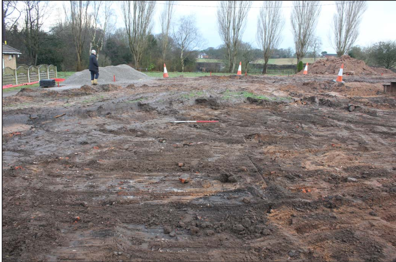
Plate 03: Pre excavation shot from South - scale 1m
