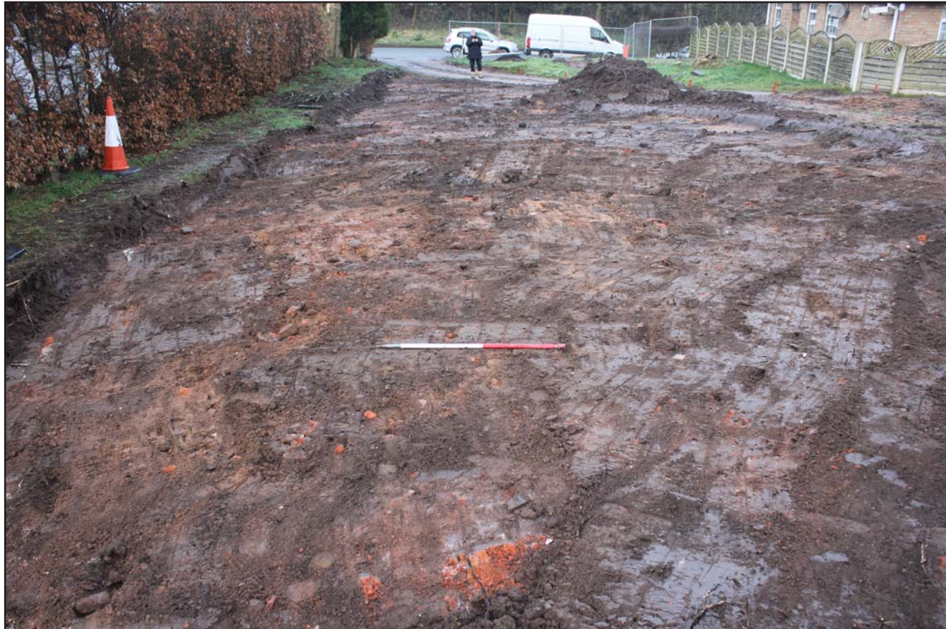
Plate 02: Pre excavation shot from East - scale 1m
