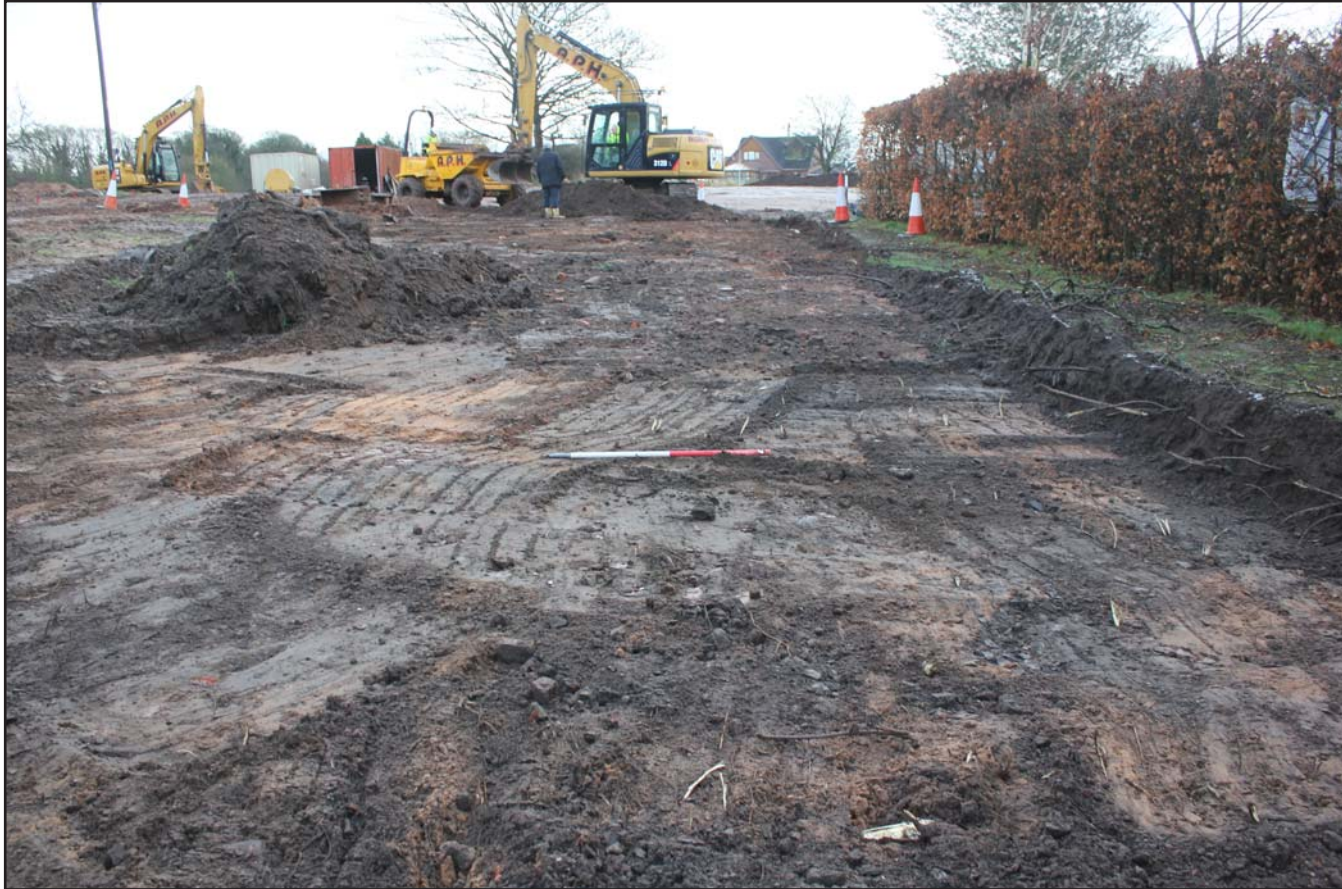
Plate 01: Pre excavation shot from West - scale 1m
