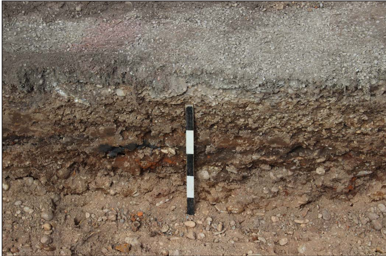
Plate 03: Generic Section; Trench 1 - from East - Scale 0.5m
