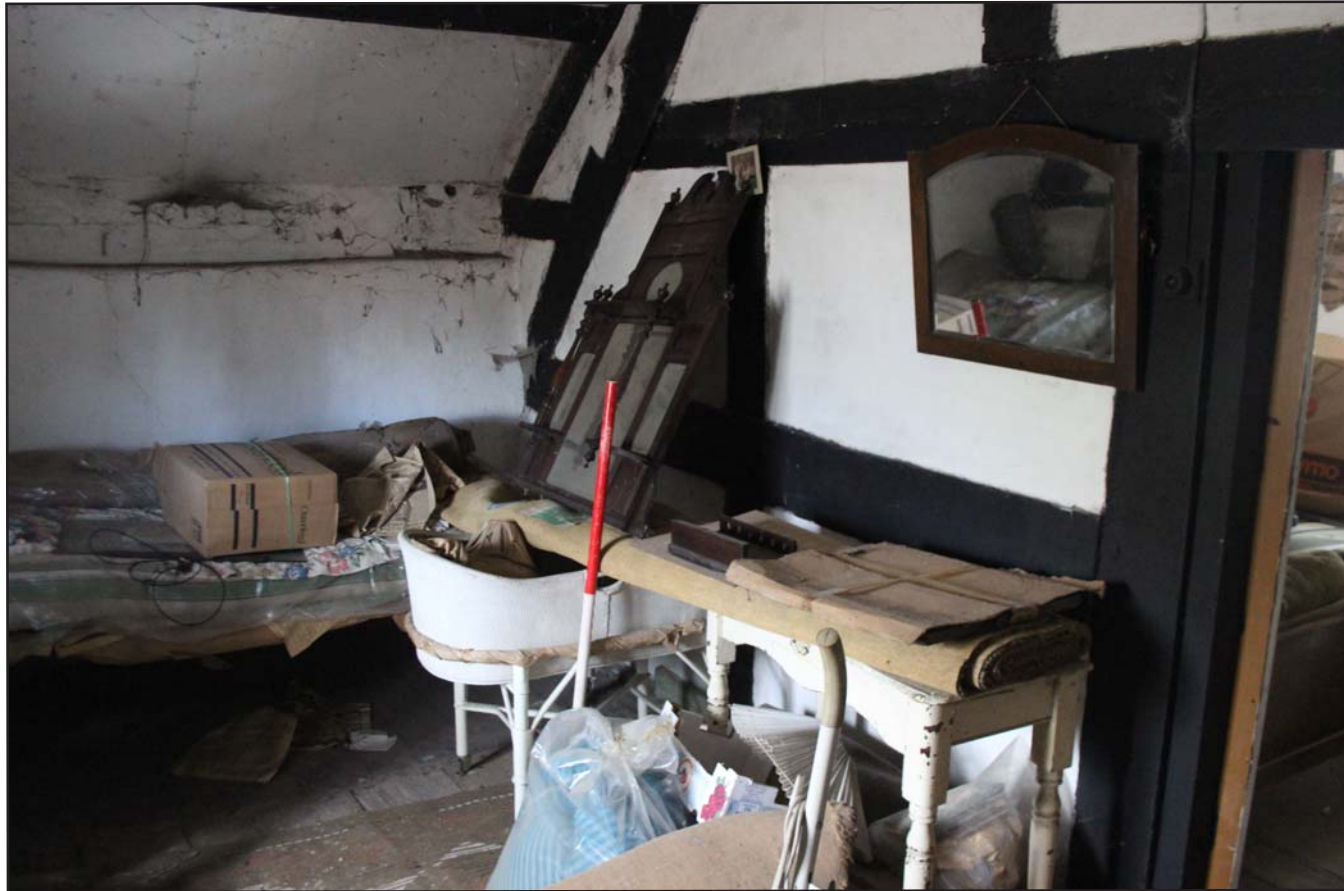
Plate 37: The Roneth- Bedroom 2 showing truss, from the north. Scale 1.0m.
