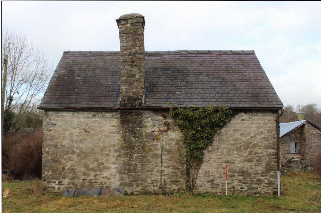
Plate 12: The Roneth- SE external elevation, from the southeast. Scale 1.0m.
