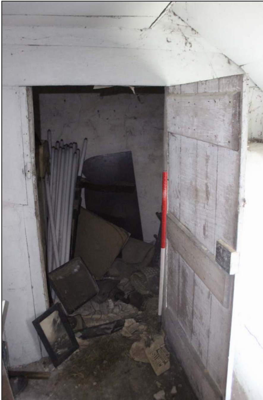
Plate 41: The Roneth- Bedroom 3 showing cupboard, from the southeast. Scale 1.0m.
