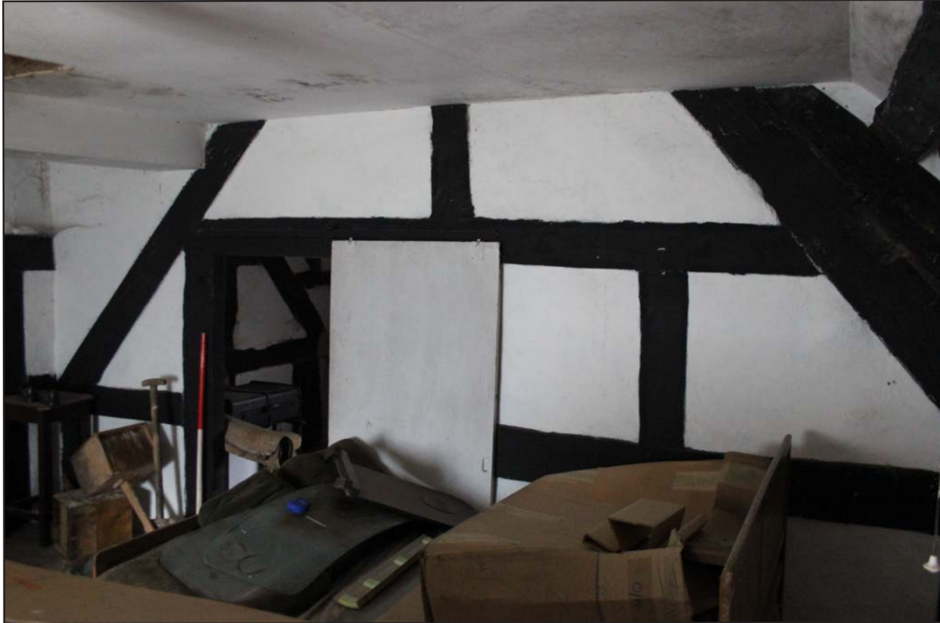
Plate 32: The Roneth- Bedroom 1 showing truss, from the south. Scale 1.0m.
