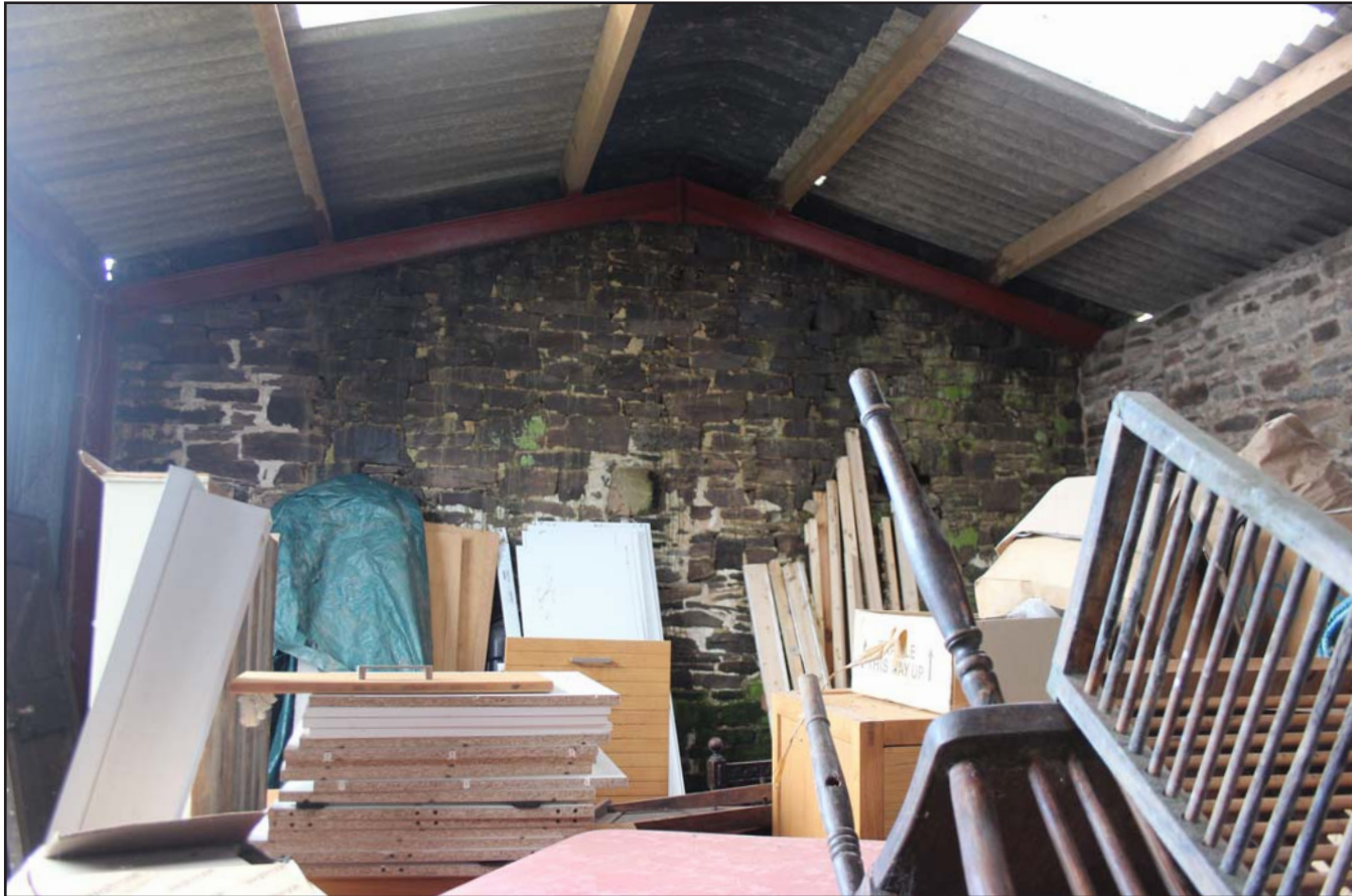
Plate 05: Outbuilding - Room 1, from the northwest.
