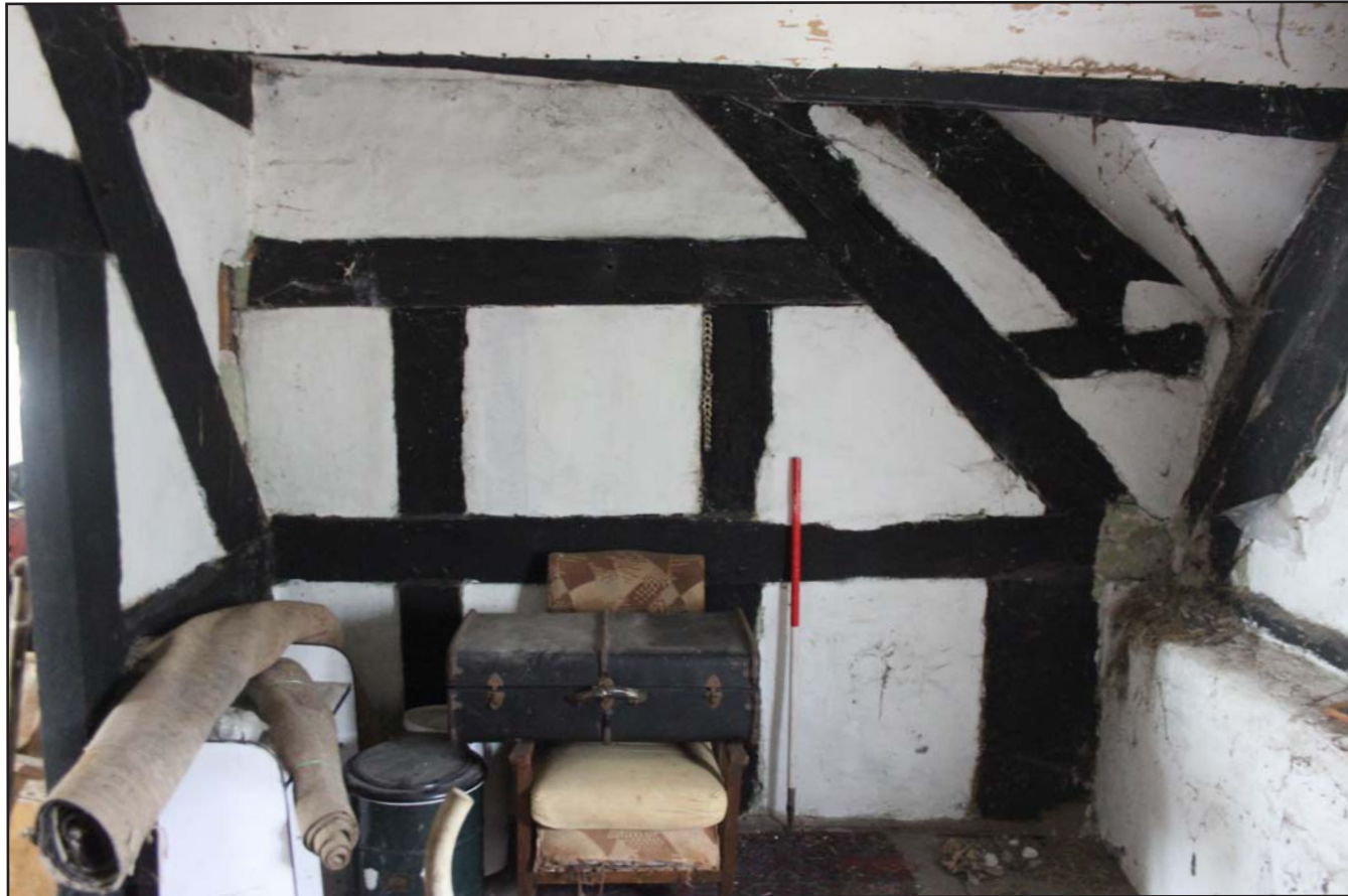
Plate 35: The Roneth- Bedroom 2 showing truss, from the southeast. Scale 1.0m.
