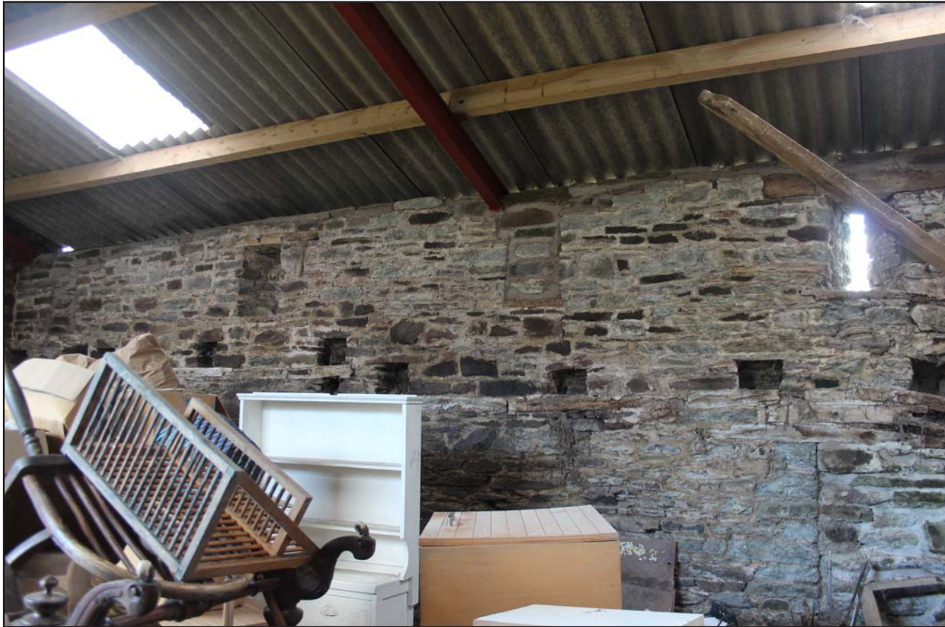
Plate 06: Outbuilding - Room 1 showing beam slots, from the northeast.
