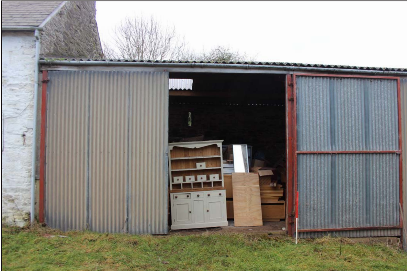
Plate 03: Outbuilding - NE external elevation showing entrance, from the northeast. Scale 1.0m.
