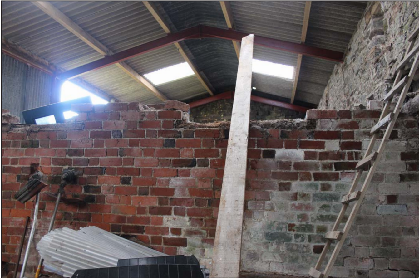
Plate 07: Outbuilding - Room 2, from the northwest.
