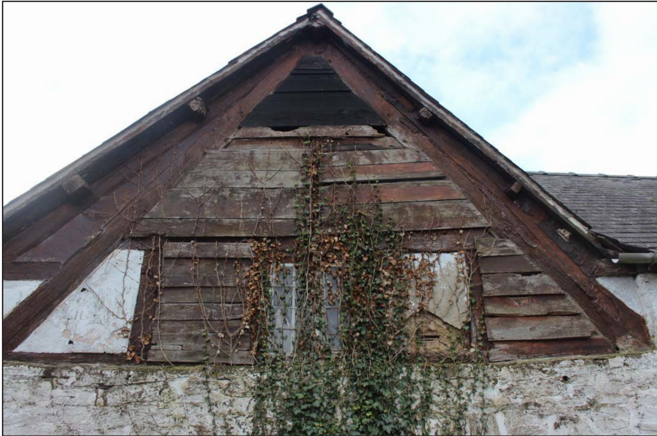
Plate 11: The Roneth- NE external elevation showing roof truss, from the northeast.
