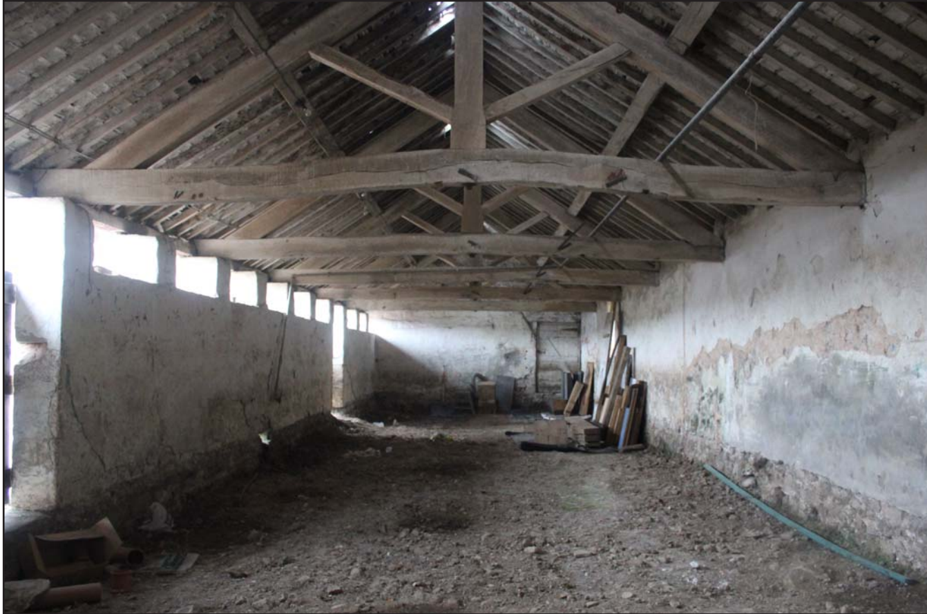
Plate 57: Llwyn y Maen, Oswestry, Shropshire. Room 9 - From the north-east - scale 1.0m
