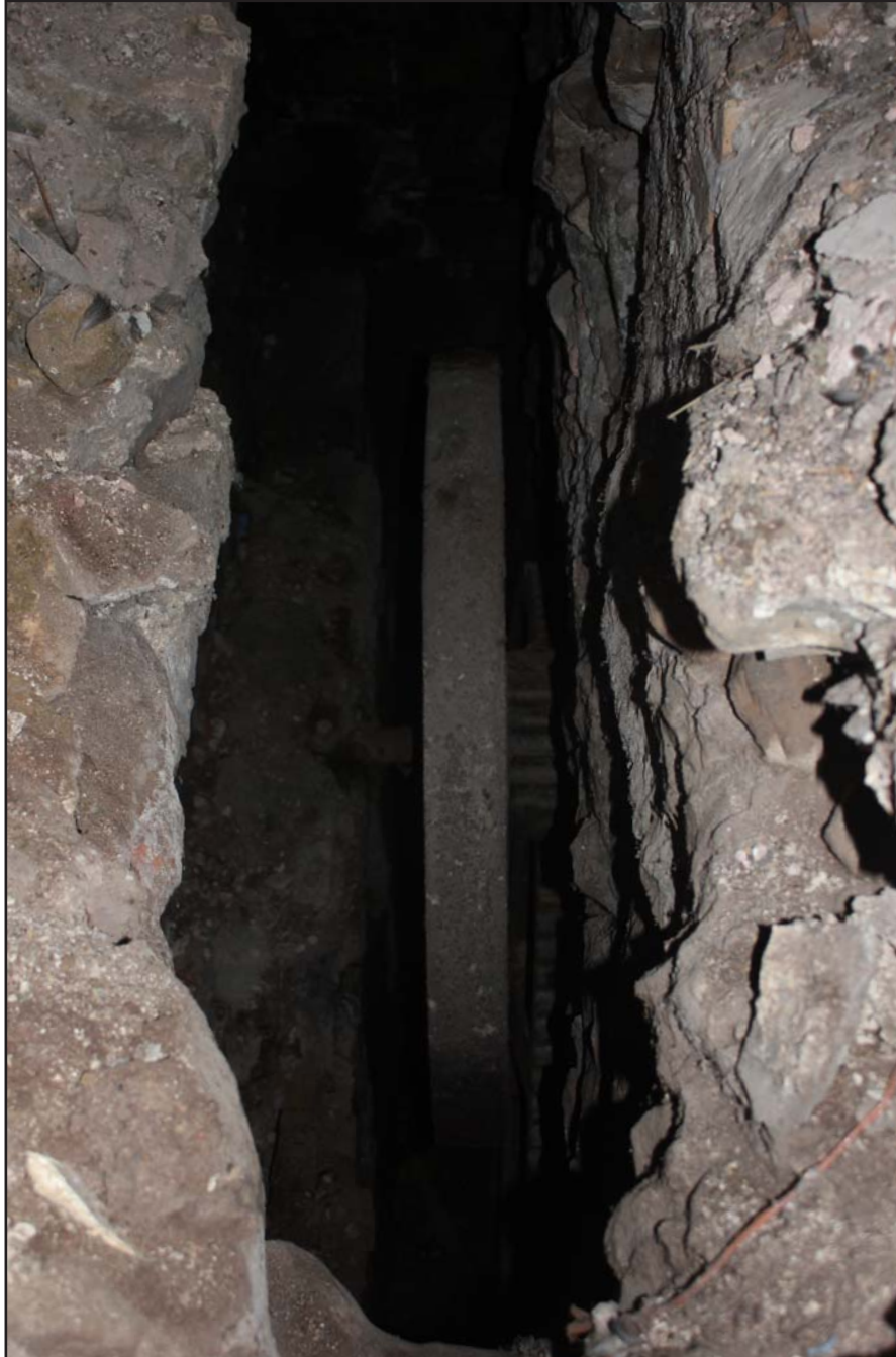
Plate 67: Room 5 - focus on cast iron water wheel in brick lined wheel pit - From the south-west- no scale
