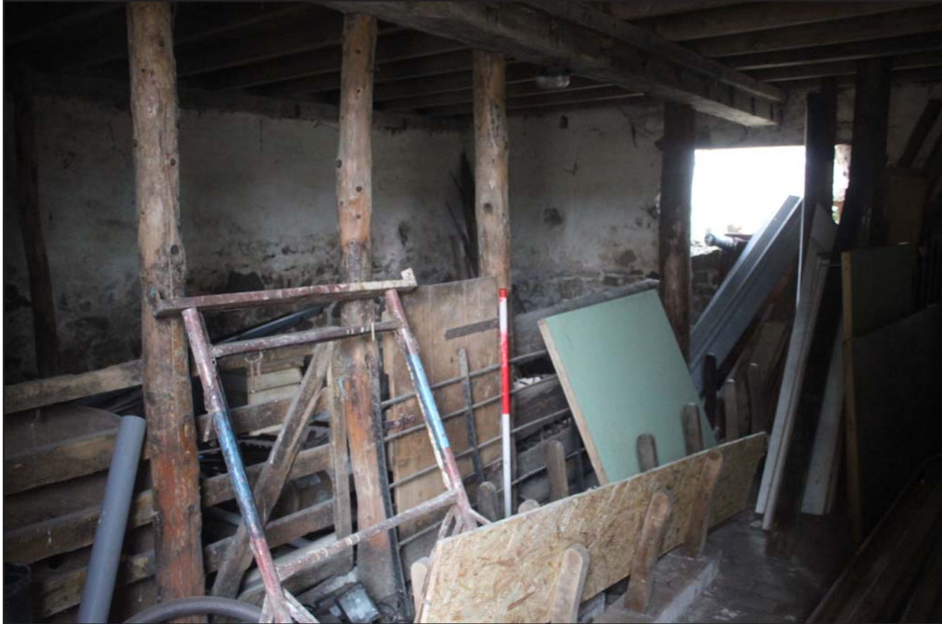
Plate 55: Llwyn y Maen, Oswestry, Shropshire. Room 8 - From the east - scale 1.0m
