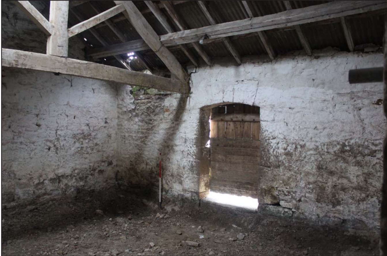
Plate 39: Llwyn y Maen, Oswestry, Shropshire. Room 2 - From the east - scale 1.0m
