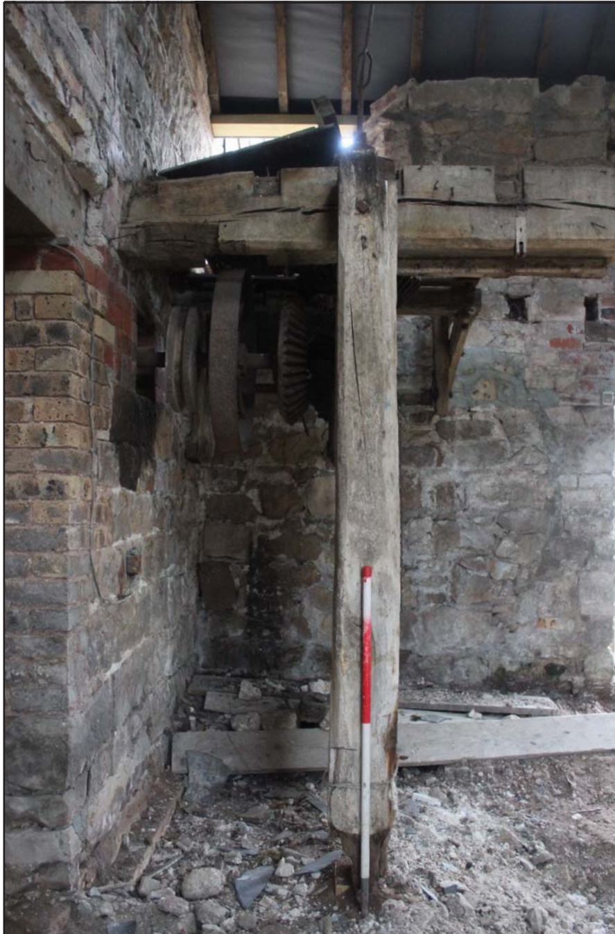
Plate 44: Llwyn y Maen, Oswestry, Shropshire. Room 4 - From the south-east - scale 1.0m
