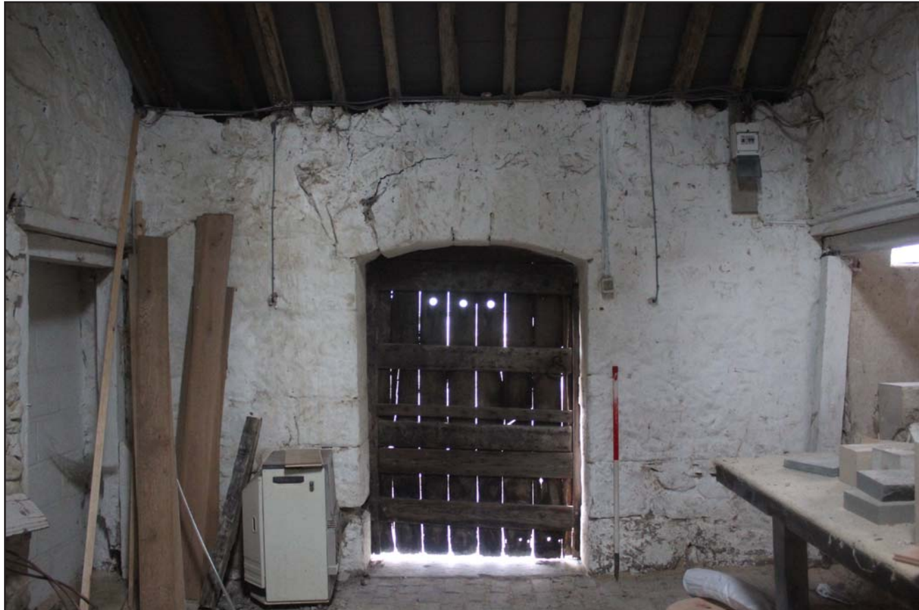
Plate 59: Llwyn y Maen, Oswestry, Shropshire. Room 10 - From the north-west - scale 1.0m
