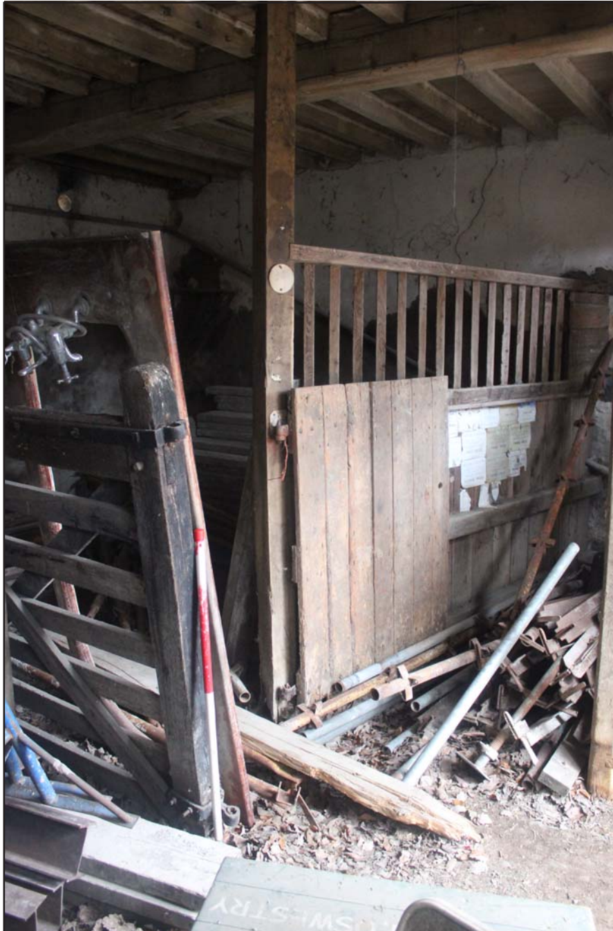
Plate 52: Llwyn y Maen, Oswestry, Shropshire. Room 7 - From the east - scale 1.0m
