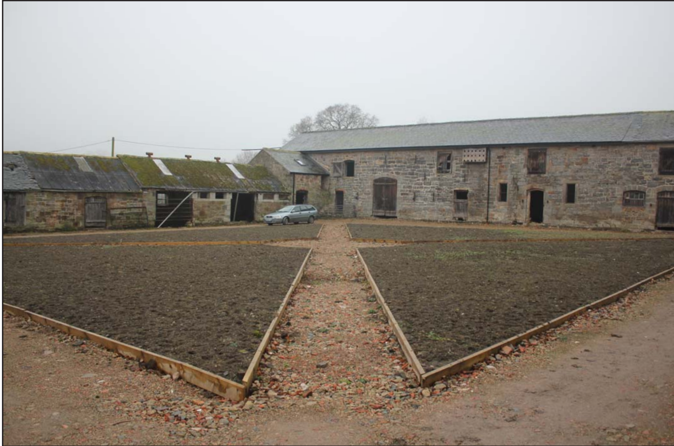
Plate 64: Llwyn y Maen, Oswestry, Shropshire. View across courtyard - Context shot - From the north - no scale
