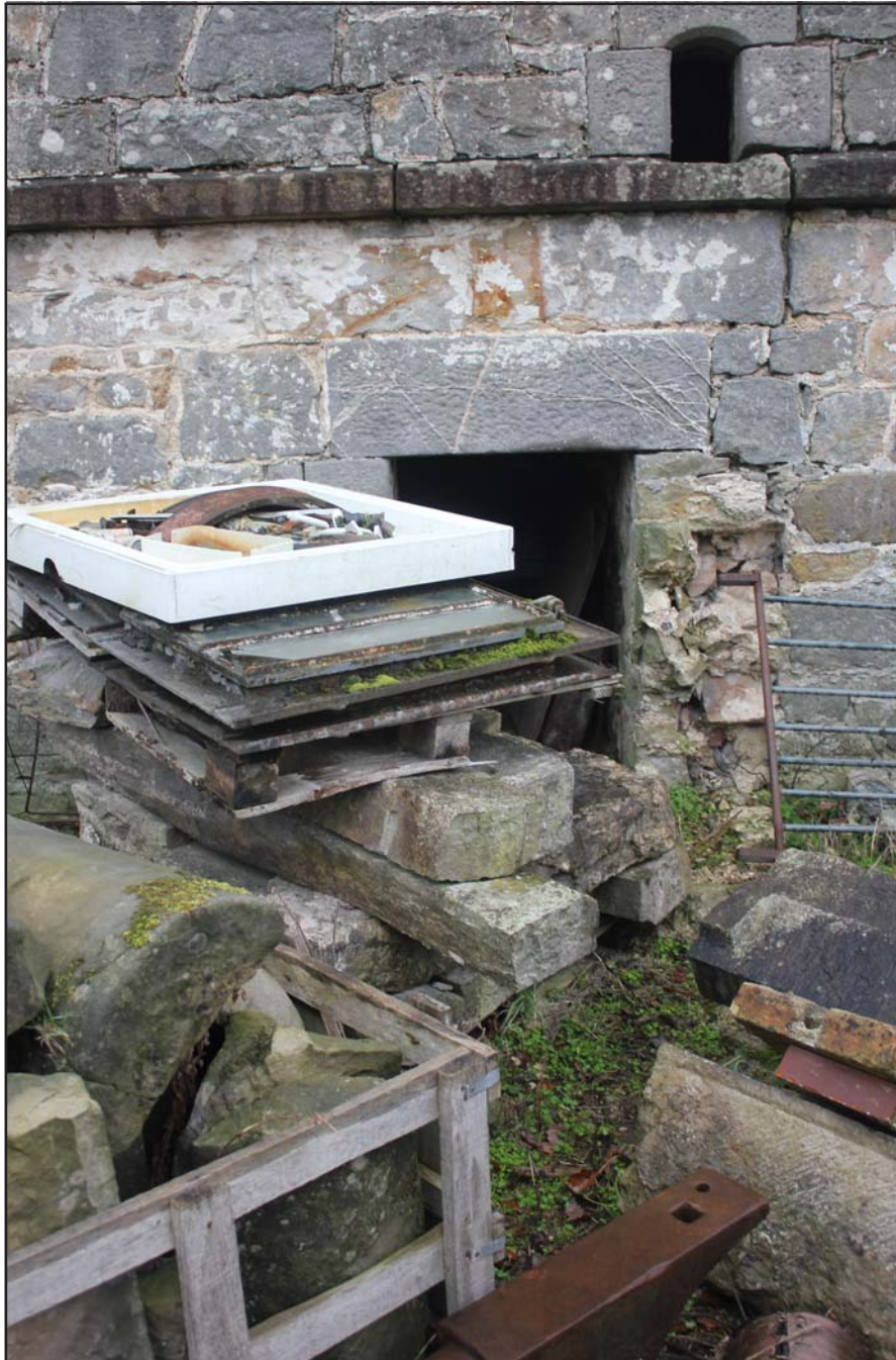
Plate 62: Llwyn y Maen, Oswestry, Shropshire. No access to Pig Sties- From the south-east - scale 1.0m
