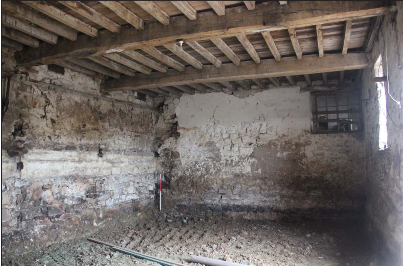
Plate 49: Llwyn y Maen, Oswestry, Shropshire. Room 6 - From the east - scale 1.0m
