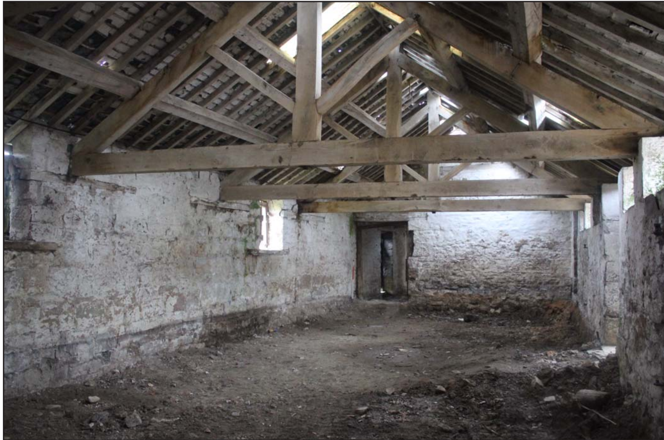
Plate 38: Llwyn y Maen, Oswestry, Shropshire. Room 1 - From the north - scale 1.0m
