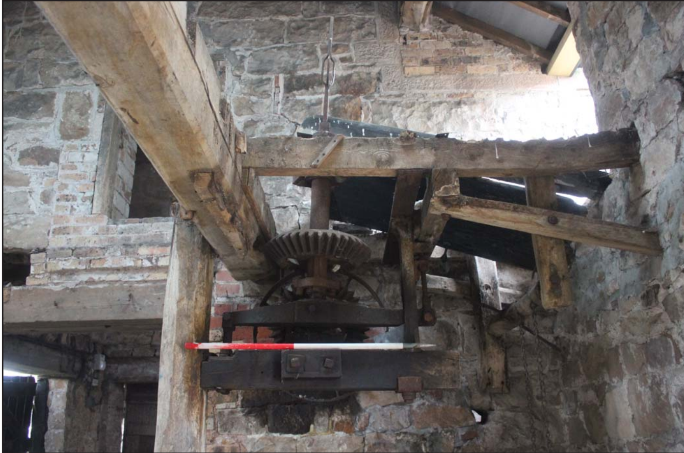
Plate 45: Llwyn y Maen, Oswestry, Shropshire. Room 4 - From the north-east - scale 1.0m
