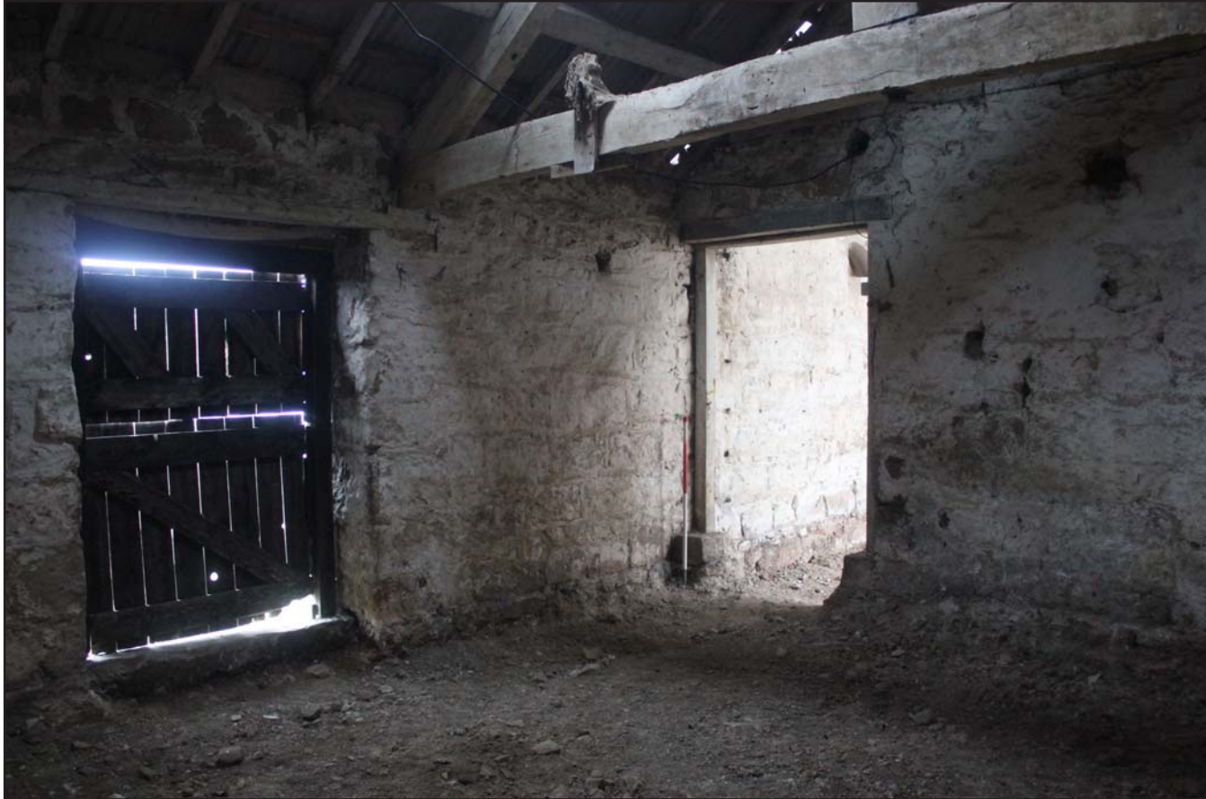
Plate 40: Llwyn y Maen, Oswestry, Shropshire. Room 2 - From the north - scale 1.0m
