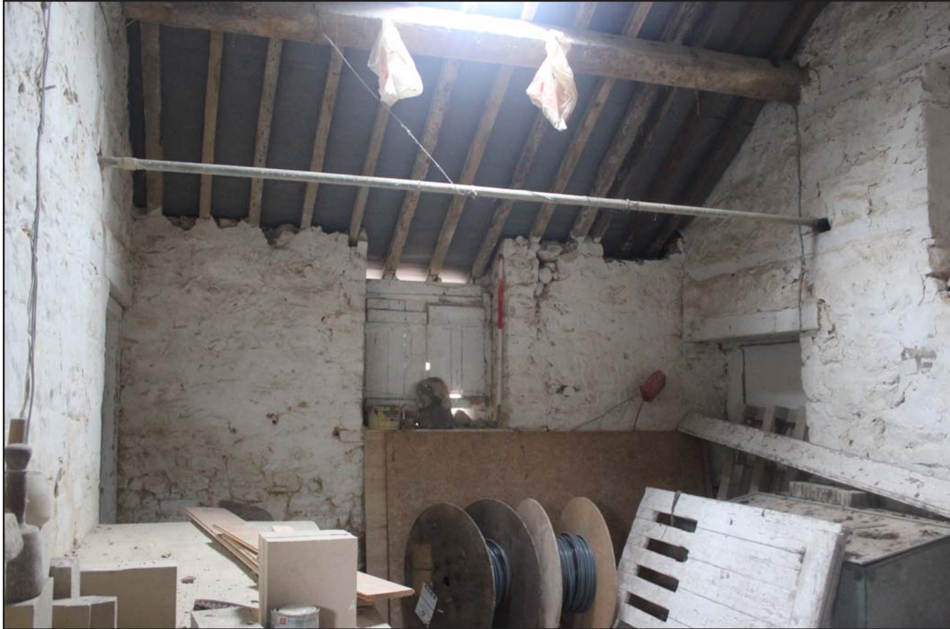
Plate 58: Llwyn y Maen, Oswestry, Shropshire. Room 10 - From the south - scale 1.0m
