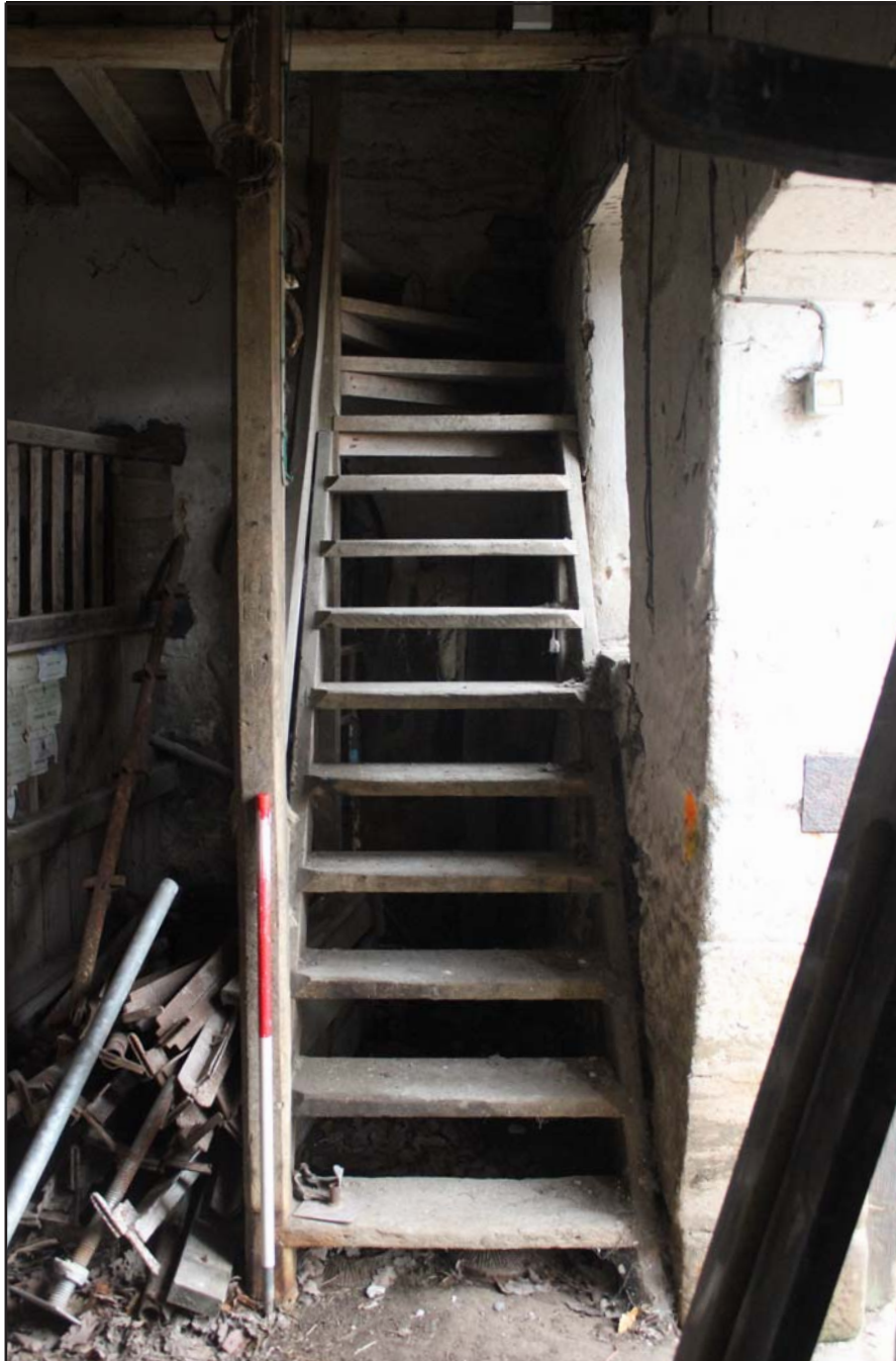
Plate 53: Llwyn y Maen, Oswestry, Shropshire. Room 7 - From the south-east - scale 1.0m
