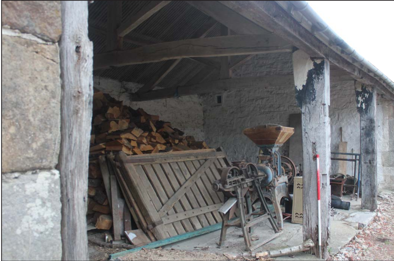
Plate 60: Llwyn y Maen, Oswestry, Shropshire. Room 11 - From the south - scale 1.0m
