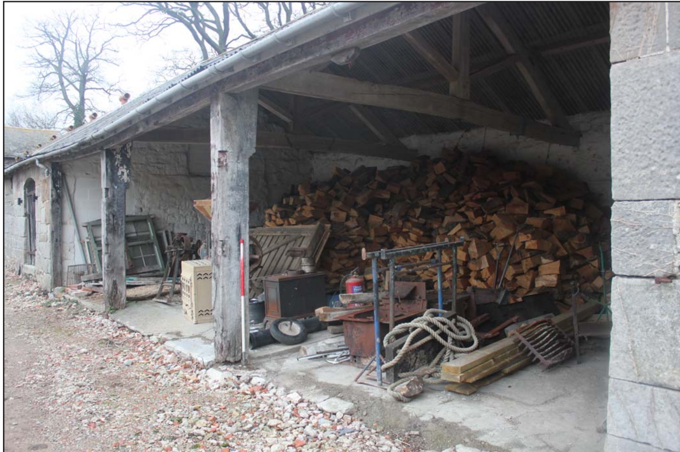
Plate 61: Llwyn y Maen, Oswestry, Shropshire. Room 11 - From the east - scale 1.0m
