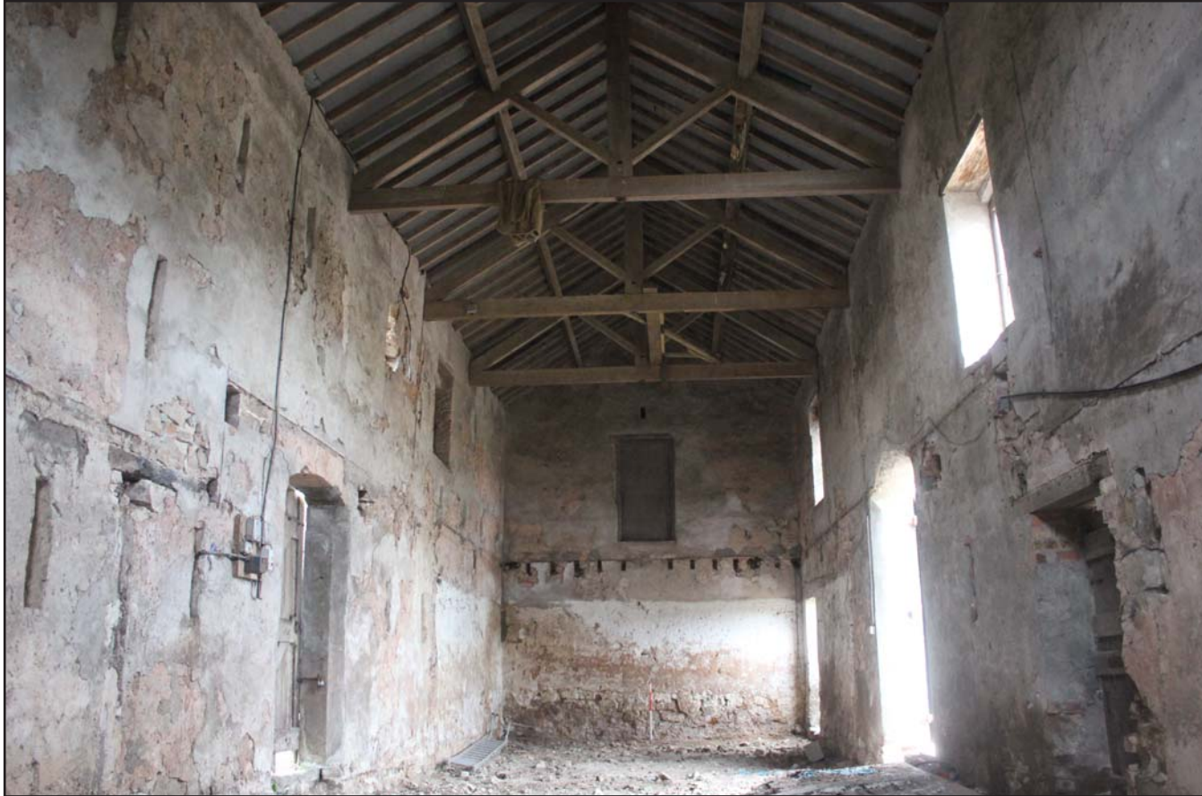
Plate 47: Llwyn y Maen, Oswestry, Shropshire. Room 5 - From the south-east - scale 1.0m
