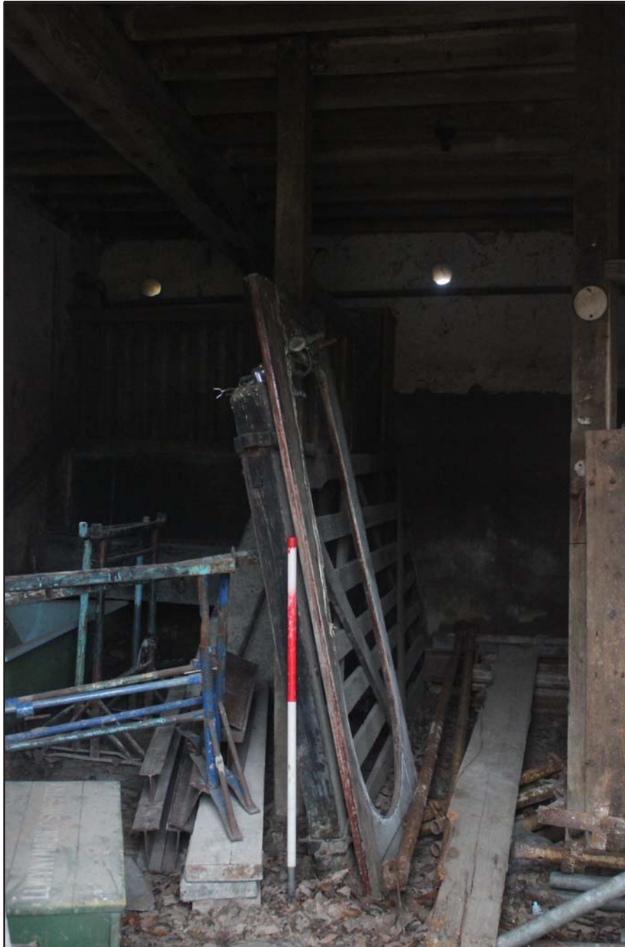
Plate 51: Llwyn y Maen, Oswestry, Shropshire. Room 7 - From the north-east - scale 1.0m
