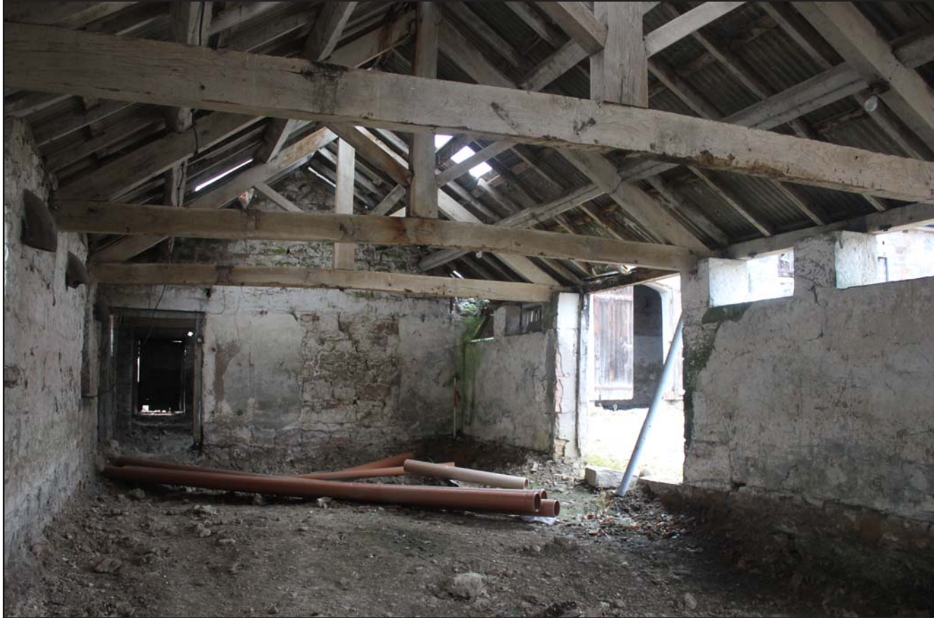
Plate 41: Llwyn y Maen, Oswestry, Shropshire. Room 3 - From the east - scale 1.0m
