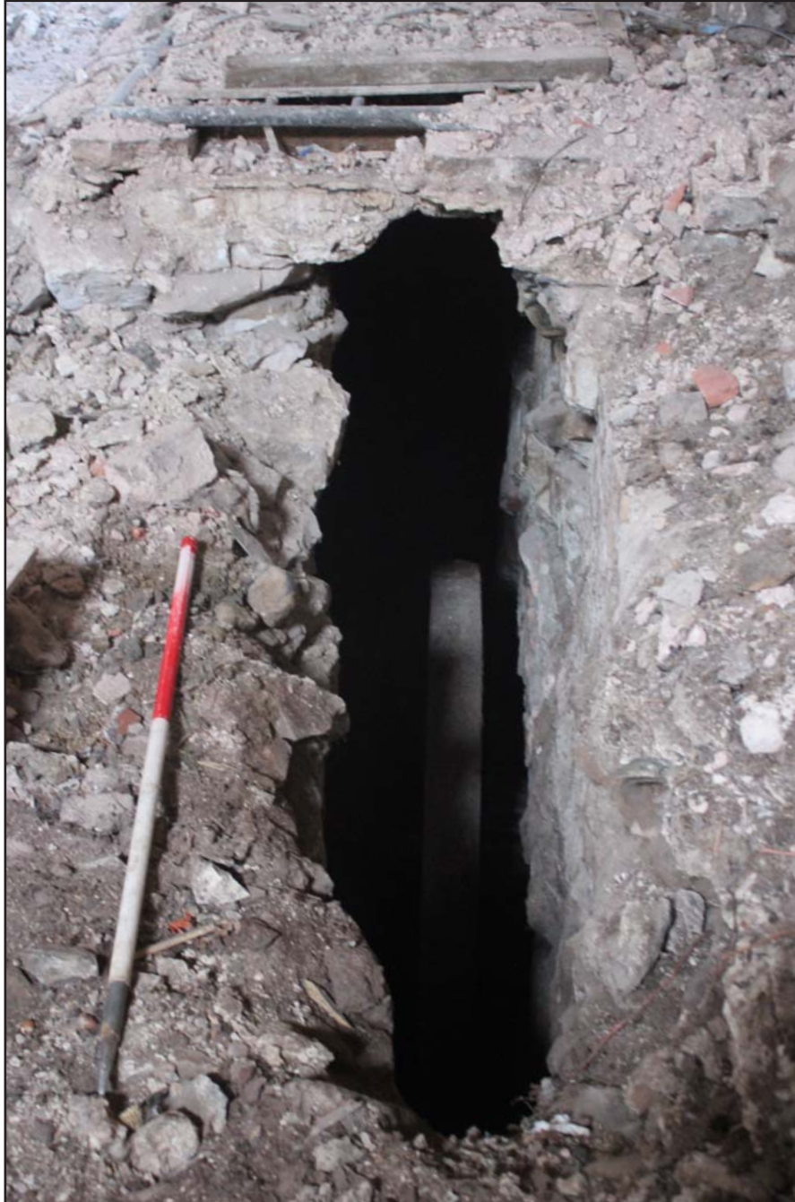
Plate 66: Room 5 - showing the subterranean water wheel and wheel pit - From the south-west- scale at 1m
