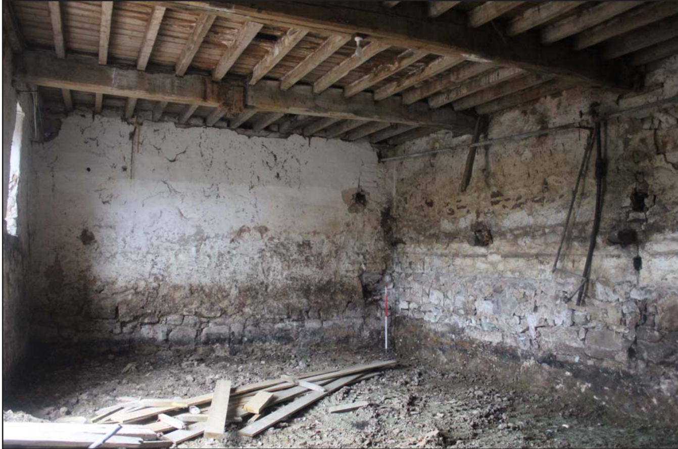
Plate 50: Llwyn y Maen, Oswestry, Shropshire. Room 6 - From the north - scale 1.0m
