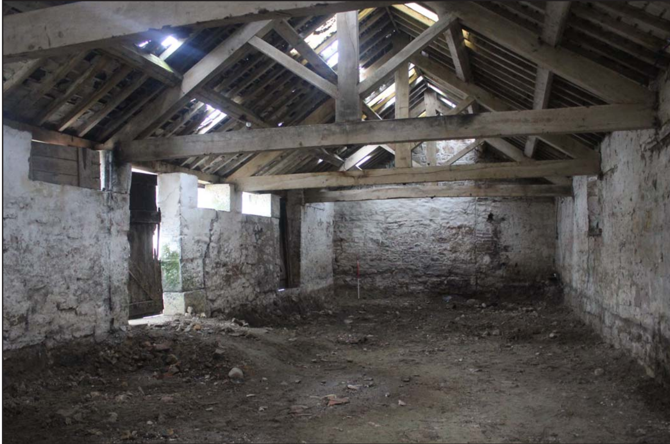
Plate 37: Llwyn y Maen, Oswestry, Shropshire. Room 1 - From the south - scale 1.0m
