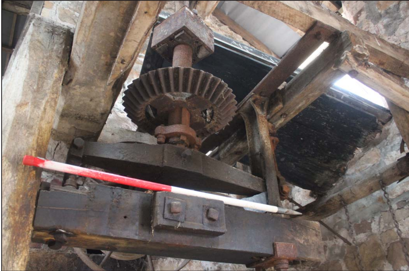
Plate 46: Llwyn y Maen, Oswestry, Shropshire. Room 4 - From the east - scale 1.0m
