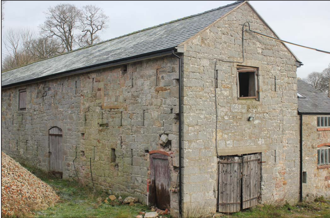
Plate 07: Llwyn y Maen, Oswestry, Shropshire. South-west and south-east elevations - From the south- scale at 1m
