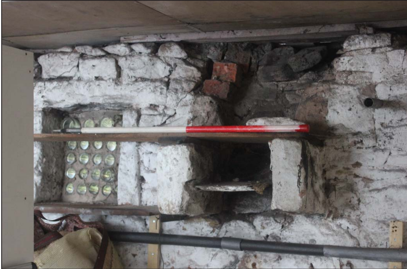
Plate 31: 317, Upton Lane, Widnes - Internals; Room 1 - Flue on north western elevation - scale 1.0m
