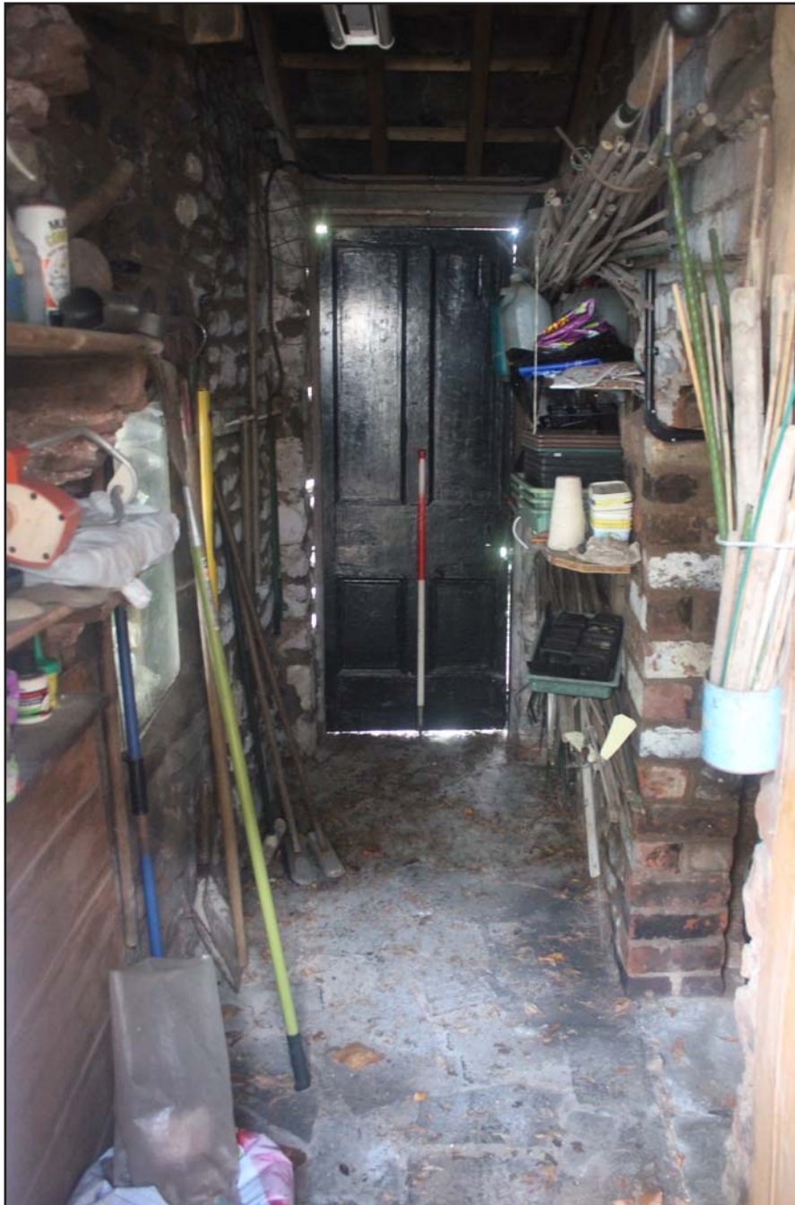
Plate 34: 317, Upton Lane, Widnes - Internals; Room 3 - From the northwest - scale 1.0m
