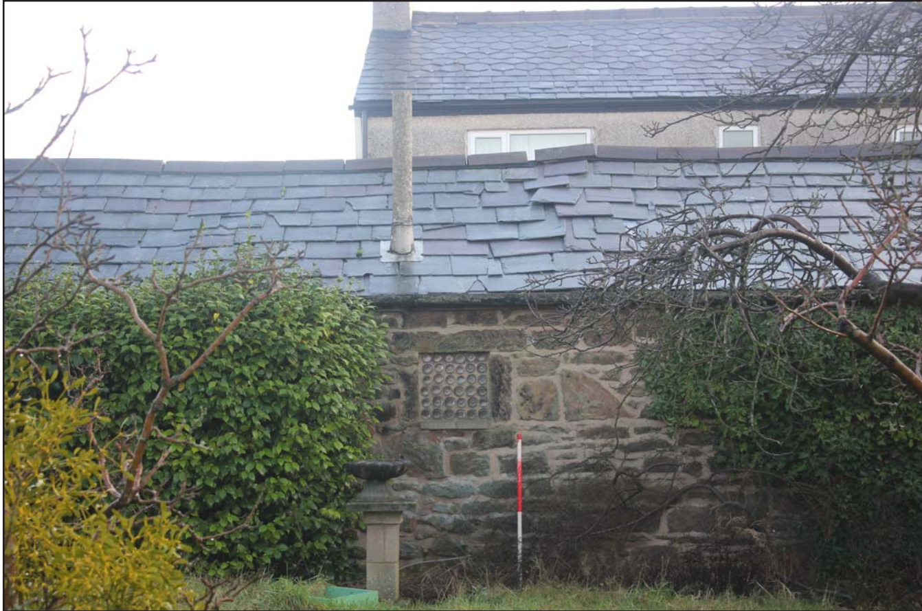
Plate 26: 317, Upton Lane, Widnes - Externals; north-western elevation of Outbuilding (centre) - From the northwest - scale 1.0m
