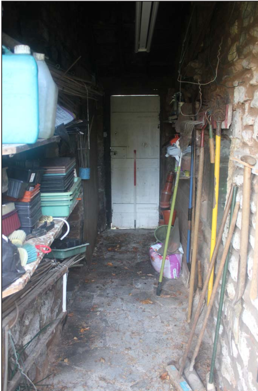
Plate 33: 317, Upton Lane, Widnes - Internals; Room 3 - From the southeast - scale 1.0m
