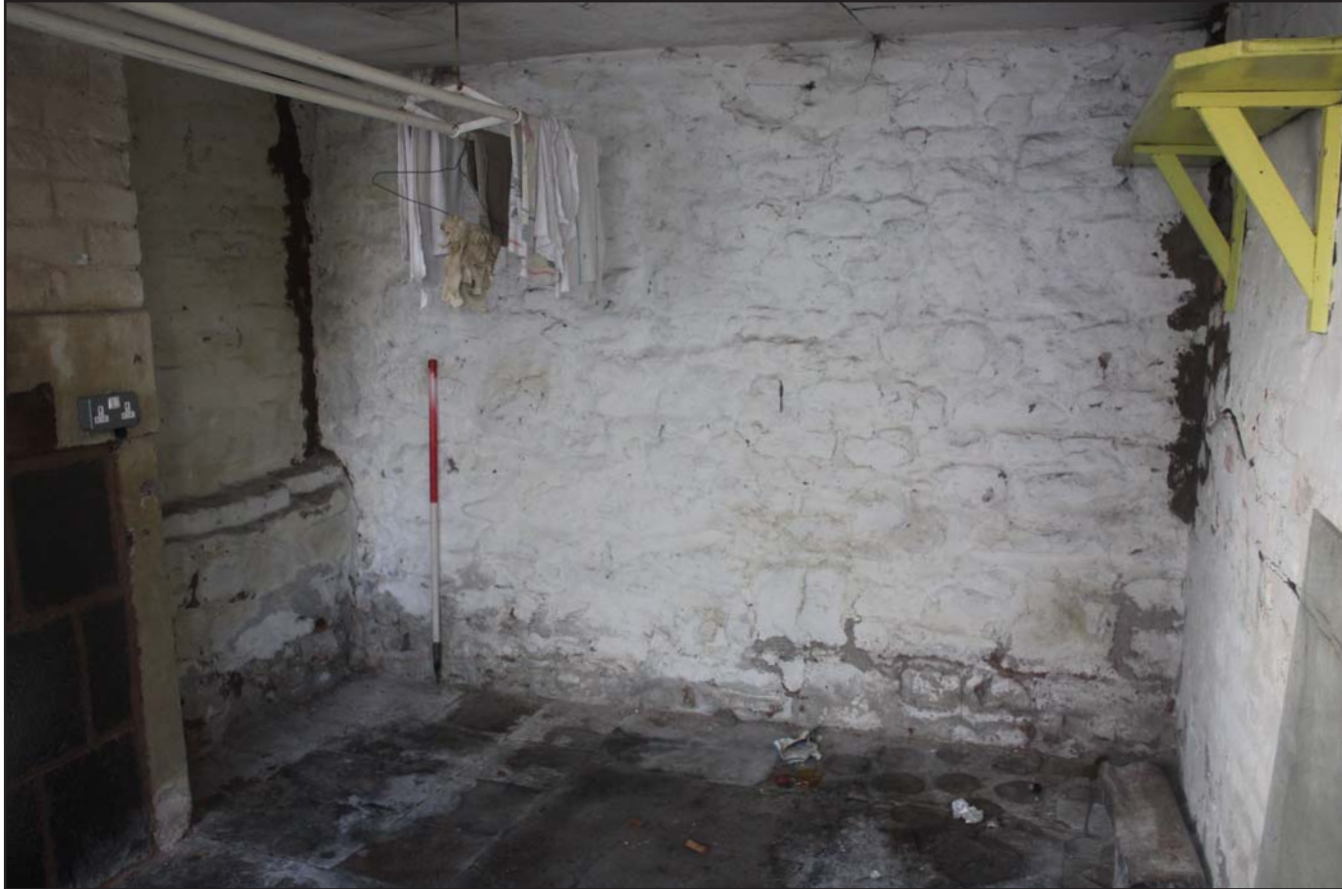
Plate 32: 317, Upton Lane, Widnes - Internals; Room 2 - From the east - scale 1.0m
