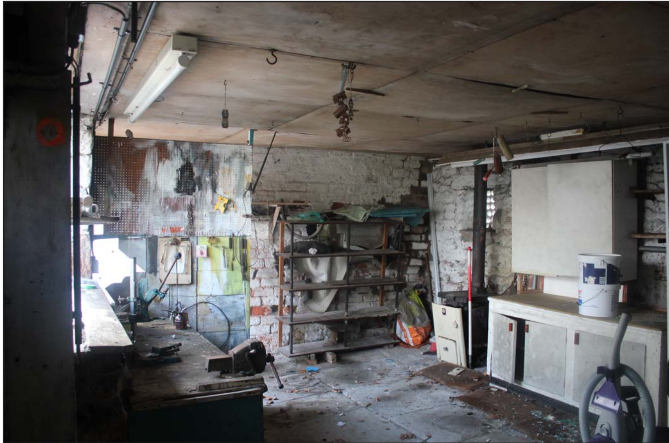
Plate 29: 317, Upton Lane, Widnes - Internals; Room 1 - From the east - scale 1.0m
