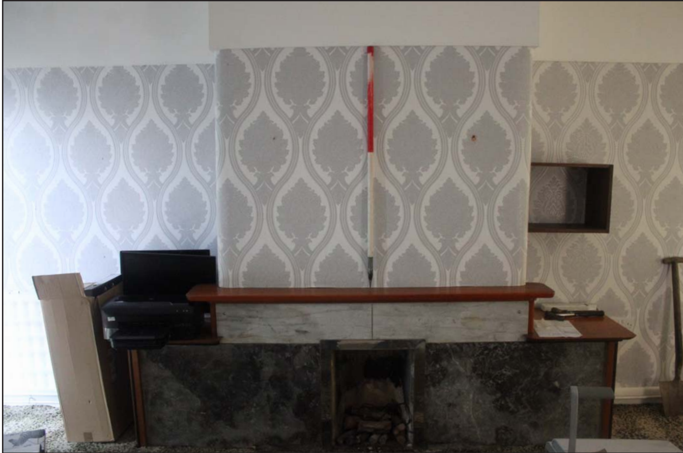
Plate 10: 317, Upton Lane, Widnes - Internal: Living room fireplace - From the northeast - scale 1.0m
