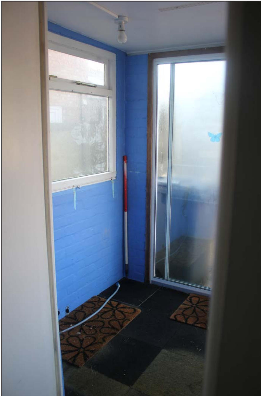
Plate 15: 317, Upton Lane, Widnes - Internal: Back Porch - From the east - scale 1.0m
