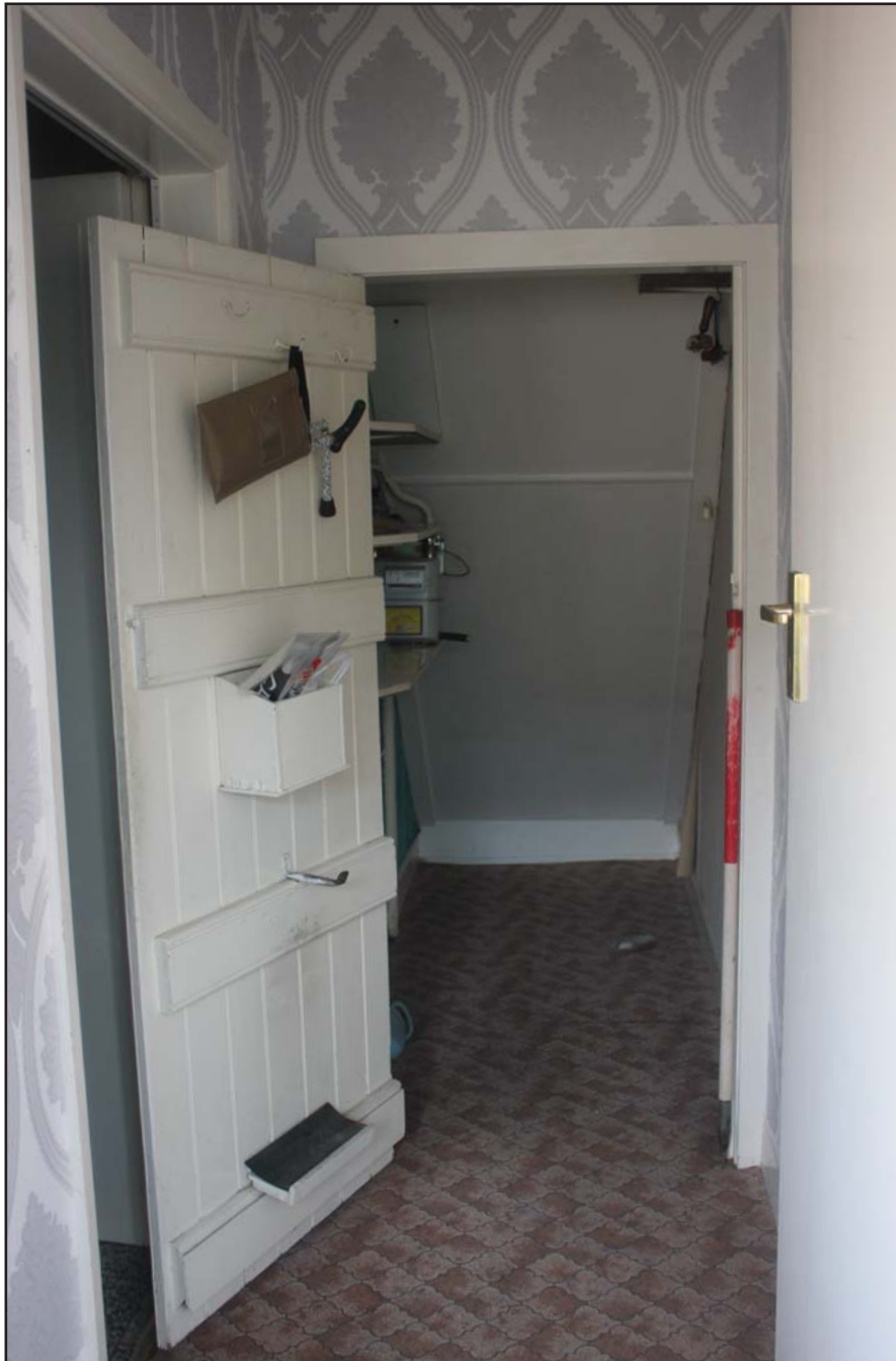
Plate 14: 317, Upton Lane, Widnes - Internal: Below stairs store - From the northeast - scale 1.0m
