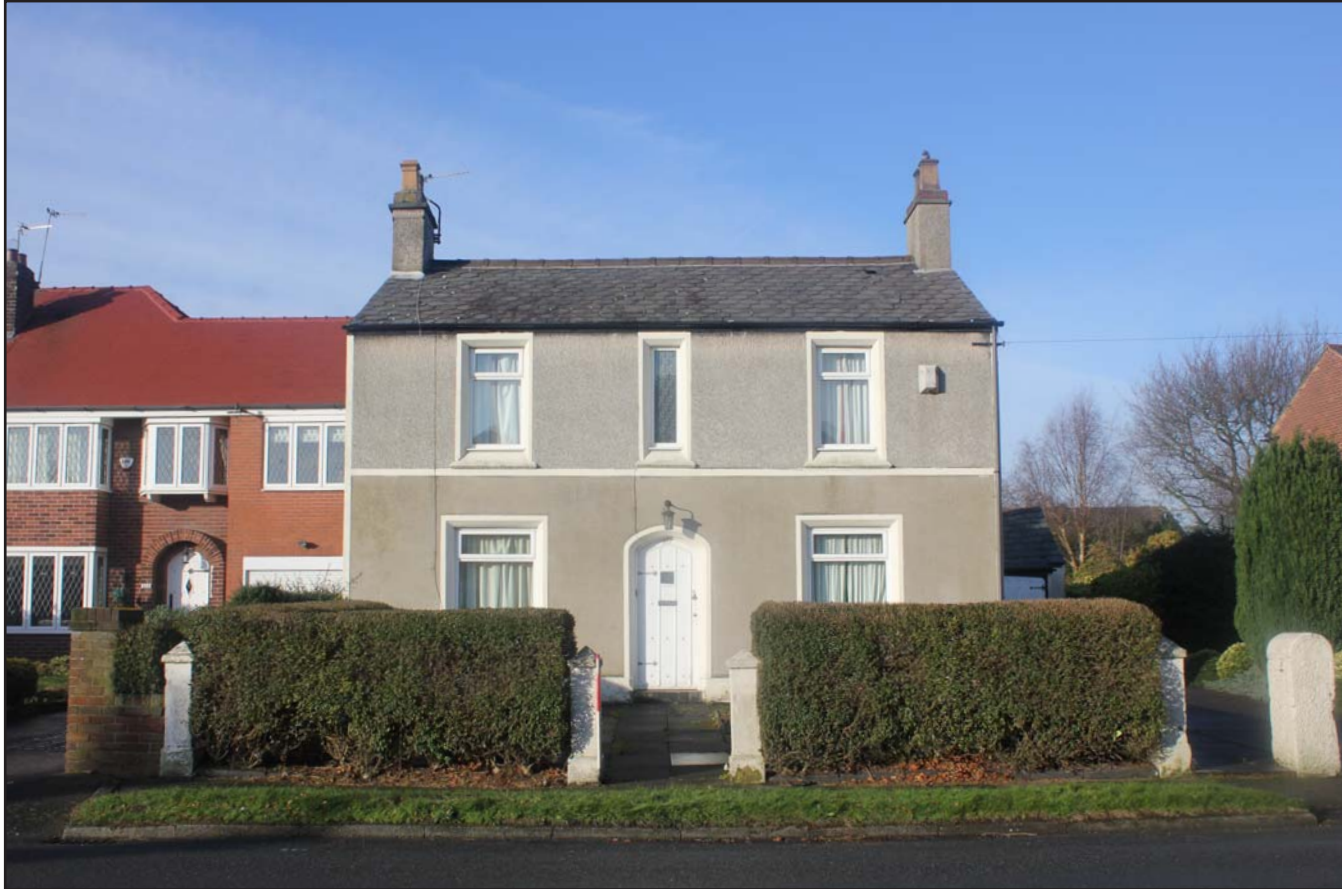
Plate 02: 317, Upton Lane, Widnes external south-eastern elevation - From the southeast - scale 1.0m
