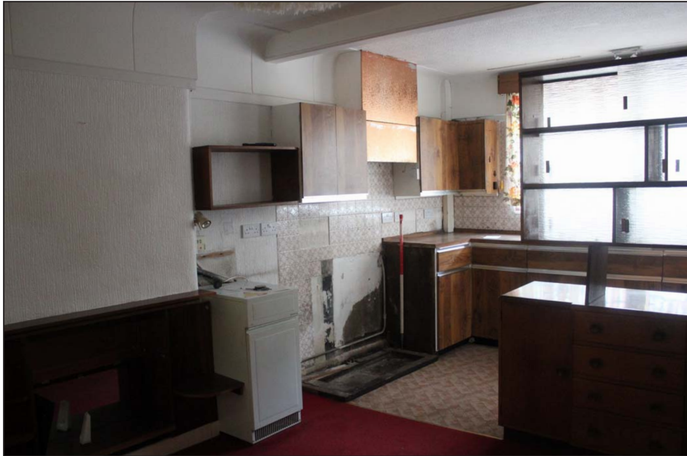
Plate 12: 317, Upton Lane, Widnes - Internal: Kitchen - From the south - scale 1.0m
