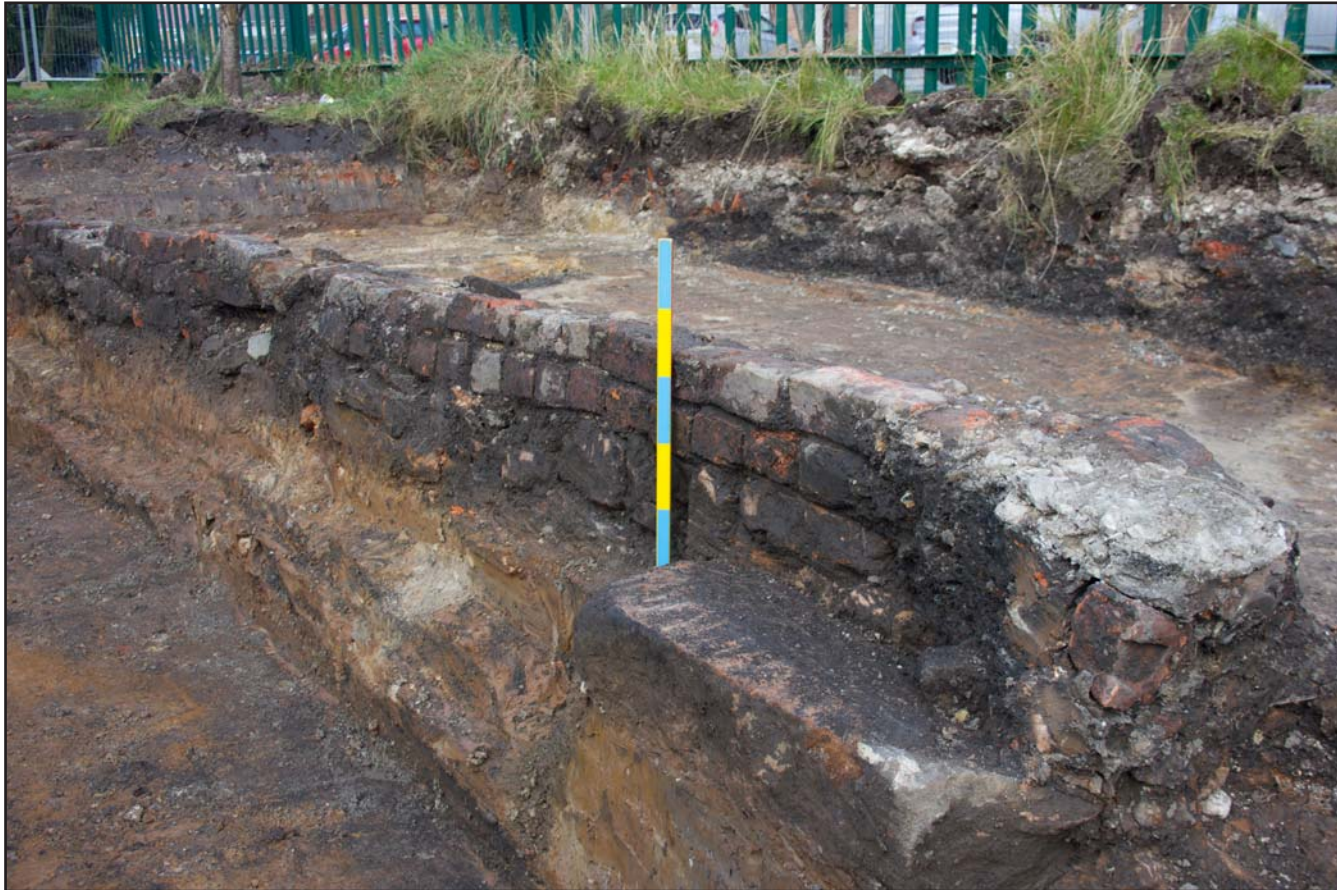
Plate 09: Oblique shot of wall (102) at Mill Wood Avenue, Eccleston, St. Helens, Merseyside - from the south - scale 0.50m
