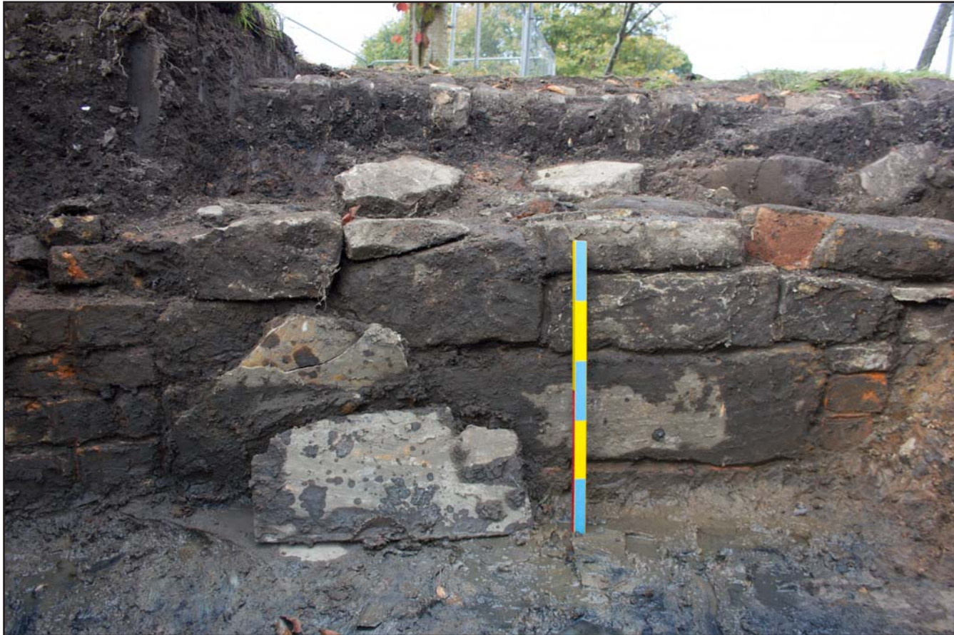
Plate 15: Elevation shot of wall (103) at Mill Wood Avenue, Eccleston, St. Helens, Merseyside - from the southeast - scale 0.50m
