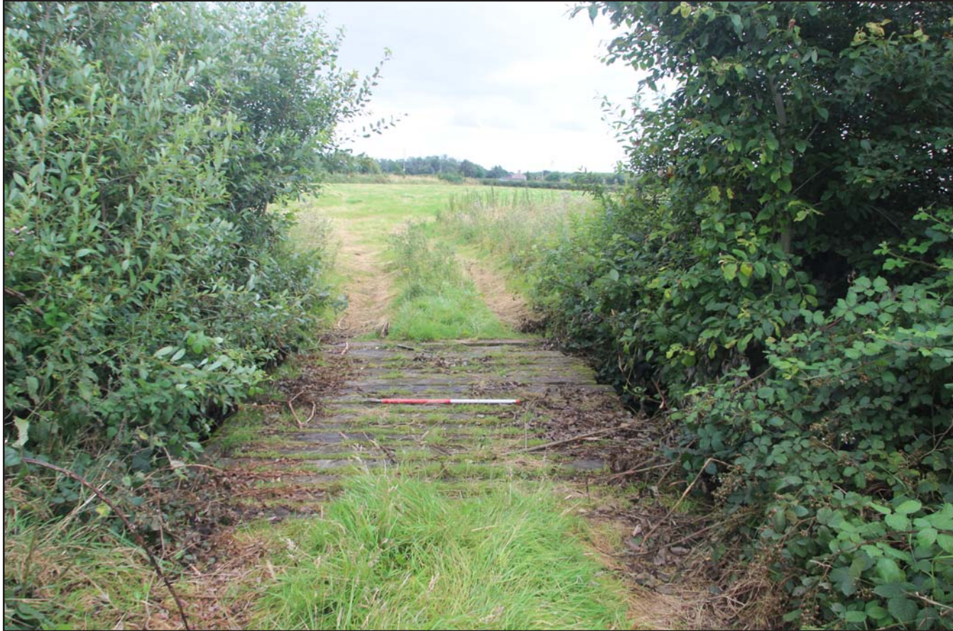
Plate 07: Bridge (feature 5), from the northwest. Scale 1.0m.
