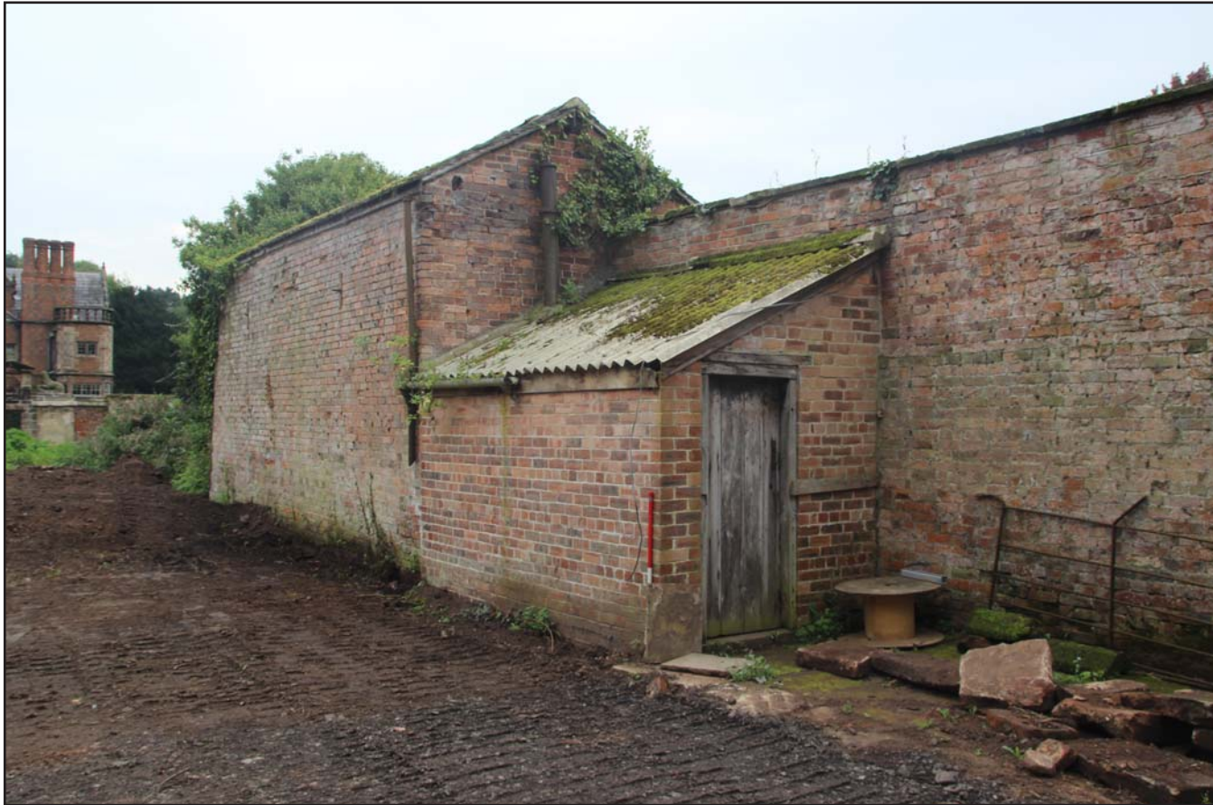
Plate 07: Outbuilding (feature 4), from the northeast. Scale 1.0m.
