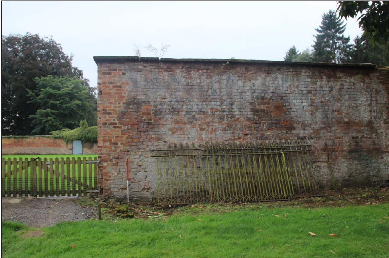
Plate 08: Kitchen garden north wall (feature 5), from the north. Scale 1.0m.
